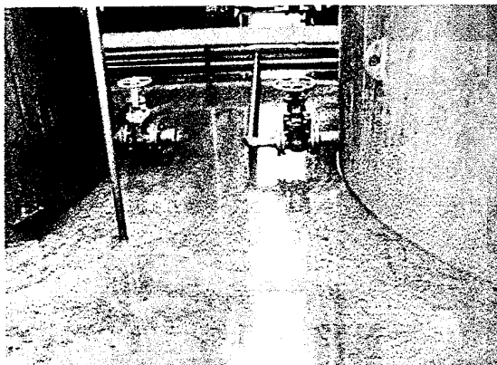
9. Oily wastewater in tankyard secondary containment
