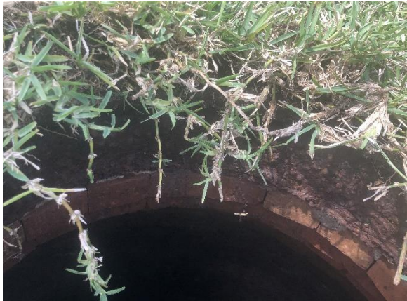
Offset Lateral (earth showing) 103'
