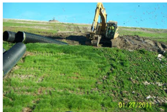
(Sediment Removal & Pipe Installation Along Southern Slope)
