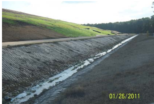
(Stormwater Conveyance System Located on Southern Perimeter of Landfill)
