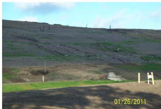
(Erosions Along Eastern Slope of Landfill)
