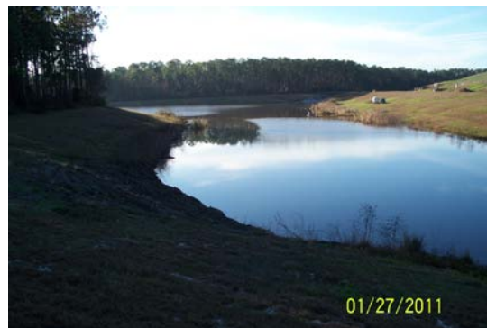
(Northern Section of SW Pond 2 With Debris Removed)
