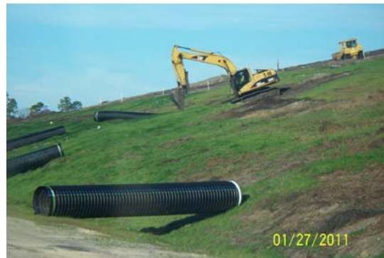
(Sediment Removal & Pipe Installation Along Southern Slope)
