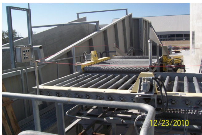
Empty primary conveyor
