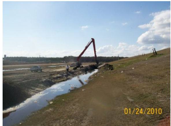
Reworking of Toe Berm
