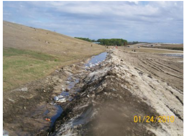
Pooled Leachate Along Toe Berm
