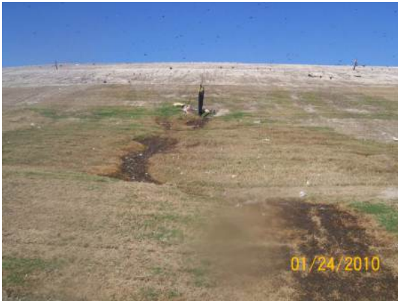
South Side Slope Leachate Seepage
