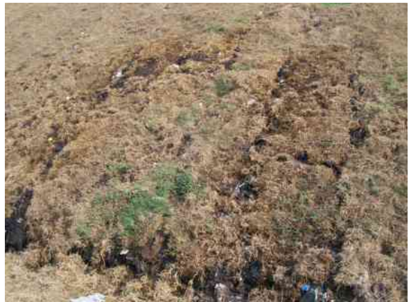
Seepage Collected by Toe Drain
