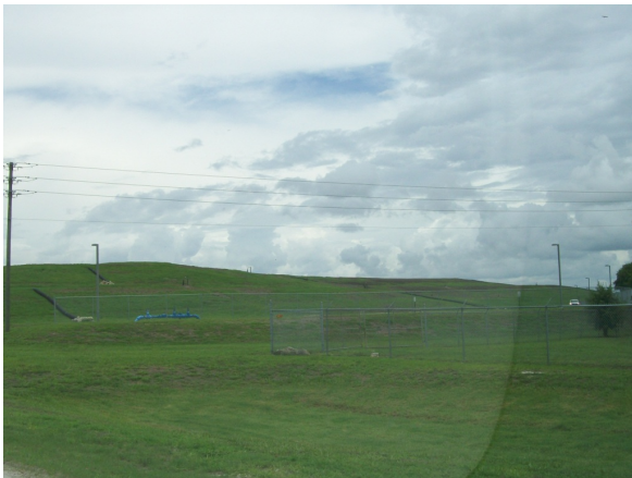
West side Stage III
