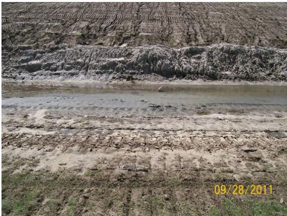
Berm at the bottom of slope
