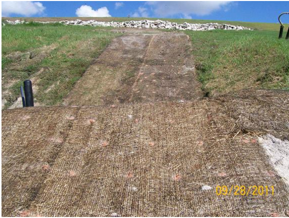
South slope reinforcement mat
