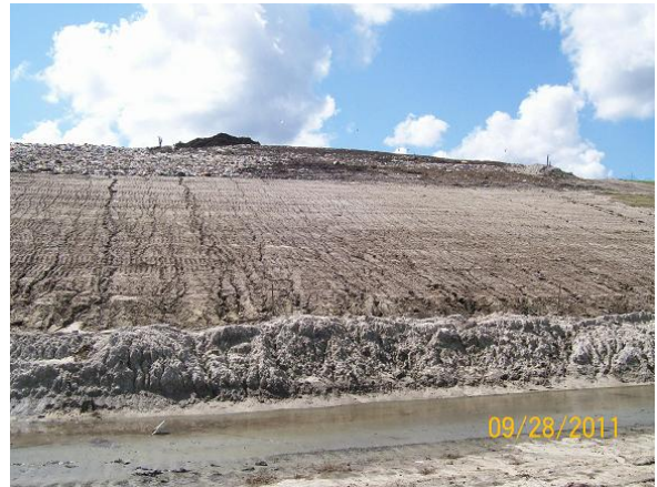
North - disposal area
