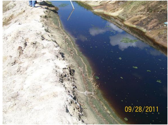
South slope toe drain
