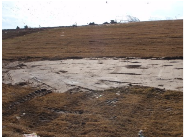
North Side Slope Seepage Repair
