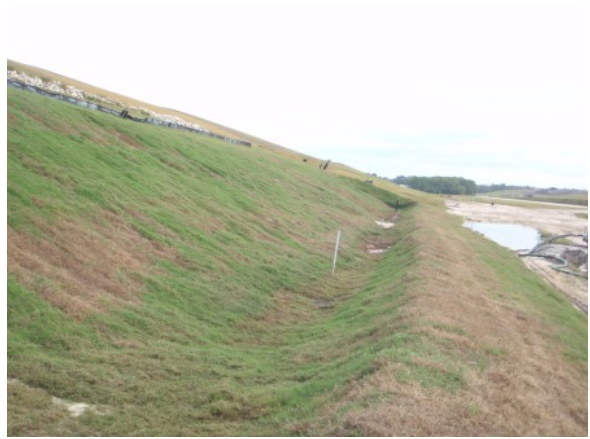
South Side Slope Toe Drain
