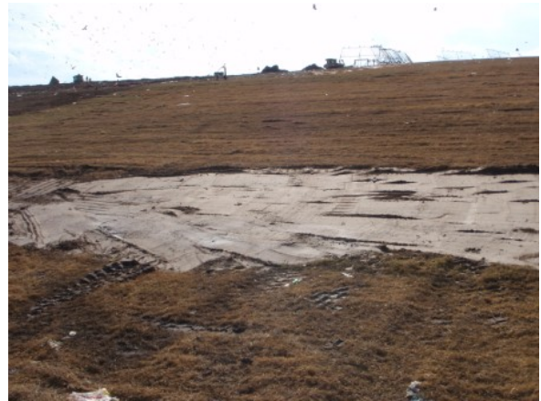
North Side Slope Seepage Repair
