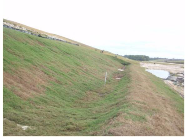
South Side Slope Toe Drain
