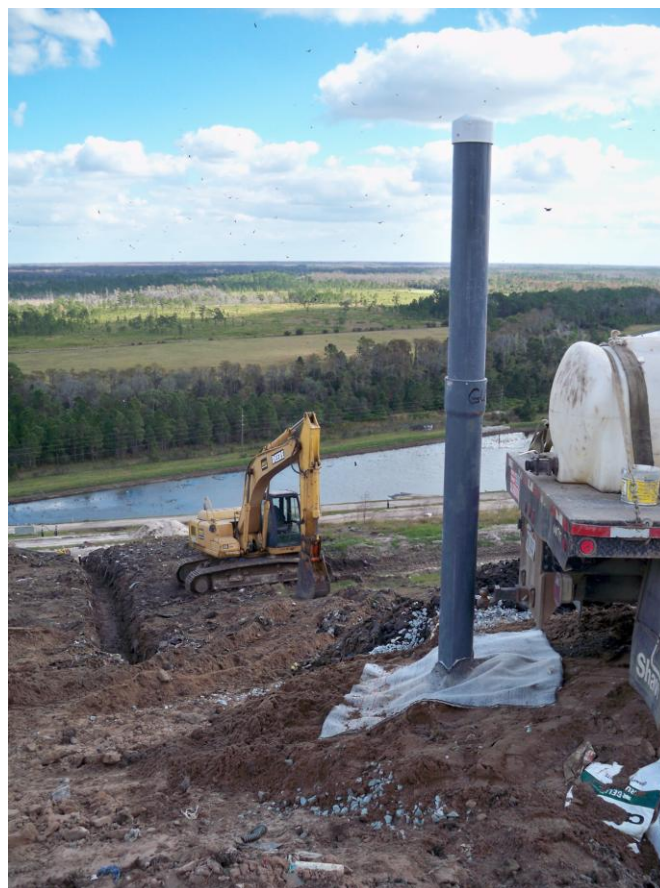
Photograph 38: GCL sheet at extraction well (typical).
