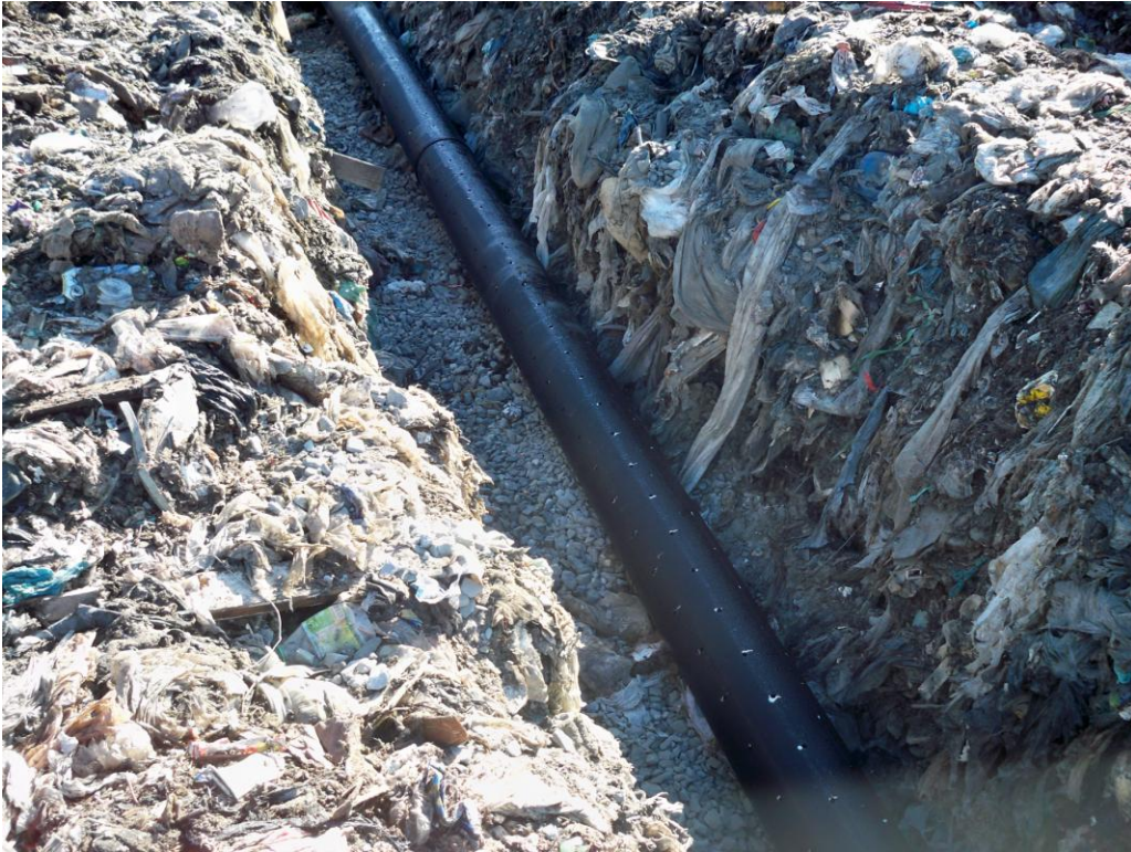
Photograph 47: 10" HDPE SDR 11 pipe above top of coarse stone. 10" First 100' of pipe to be solid 10" HDPE and remaining pipe to be perforated 10" HDPE. (typ).
