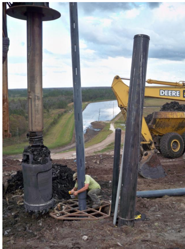
Photograph 32: Lag bolting joints to provided additional support (typical).
