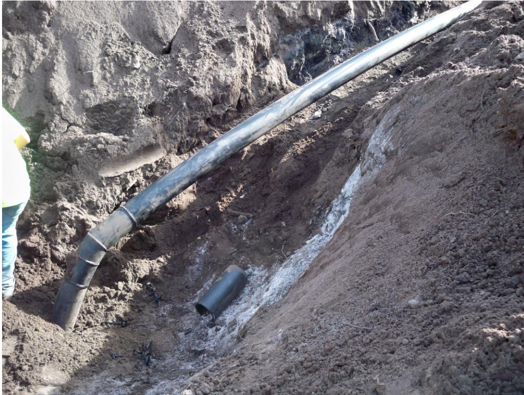
Photograph 41: Extending existing lateral towards redrill well (typ).
