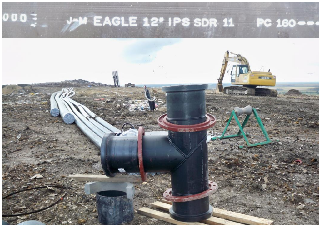
Photograph 18: 12" HDPE SDR 11 tee with flange adapters and backup rings.
