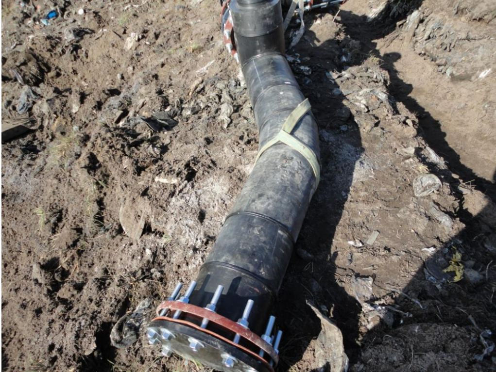
Photograph 21: 12" HDPE SDR 17 blind flange for future expansion.
