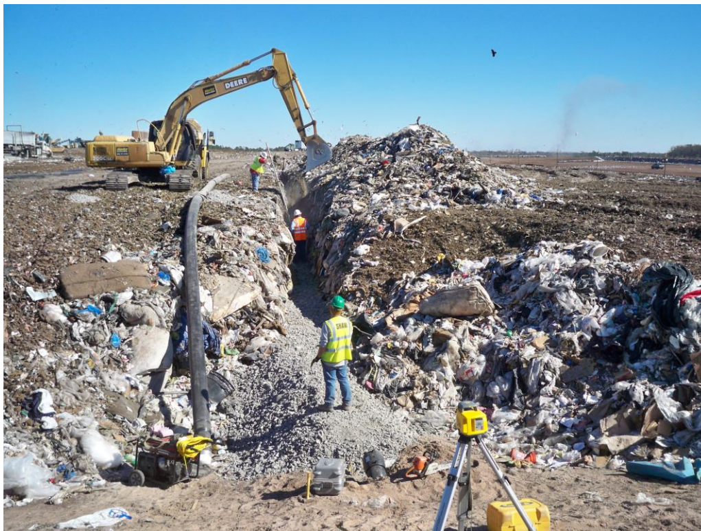
Photograph 43: For horizontal gas collectors (HGC), survey slope construction laser set at 3% for trenching solid pipe portion and 5% for perforated pipe portion (typical).
