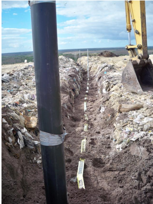
Photograph 29: Backfilled trench. Caution tape applied and survey posts every 50 'and at points of interest (typical).
