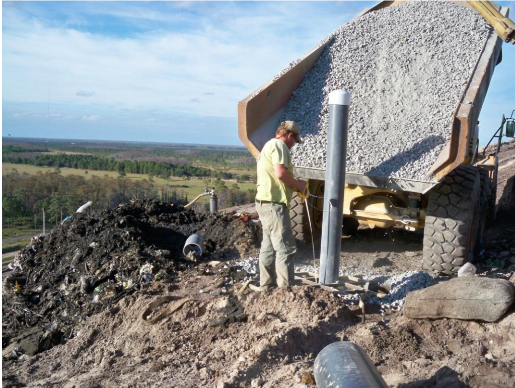
Photograph 33: Backfilling extraction well with stone and measuring stone depth (typ).
