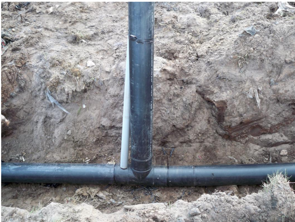
Photograph 28: Lateral riser with tee and top-of-pipe survey riser (typical).
