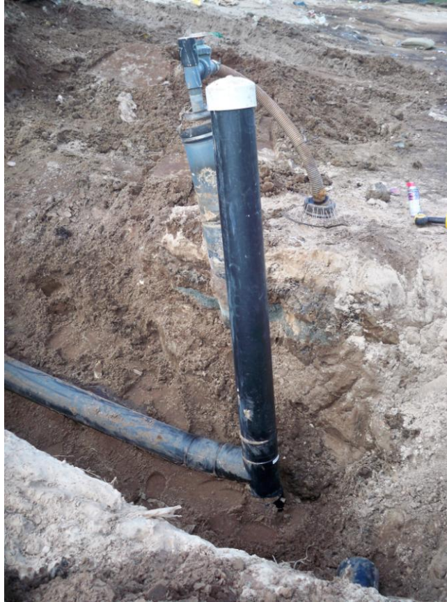
Photograph 25: Tie-in to existing lateral riser for lateral expansion (typical).
