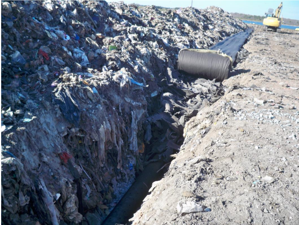
Photograph 49: Backfill trench approximately 1 ½ ft above top of 10-inch HDPE SDR 11 pipe with tire chips. Place 8 oz geotextile above tire chip backfill
