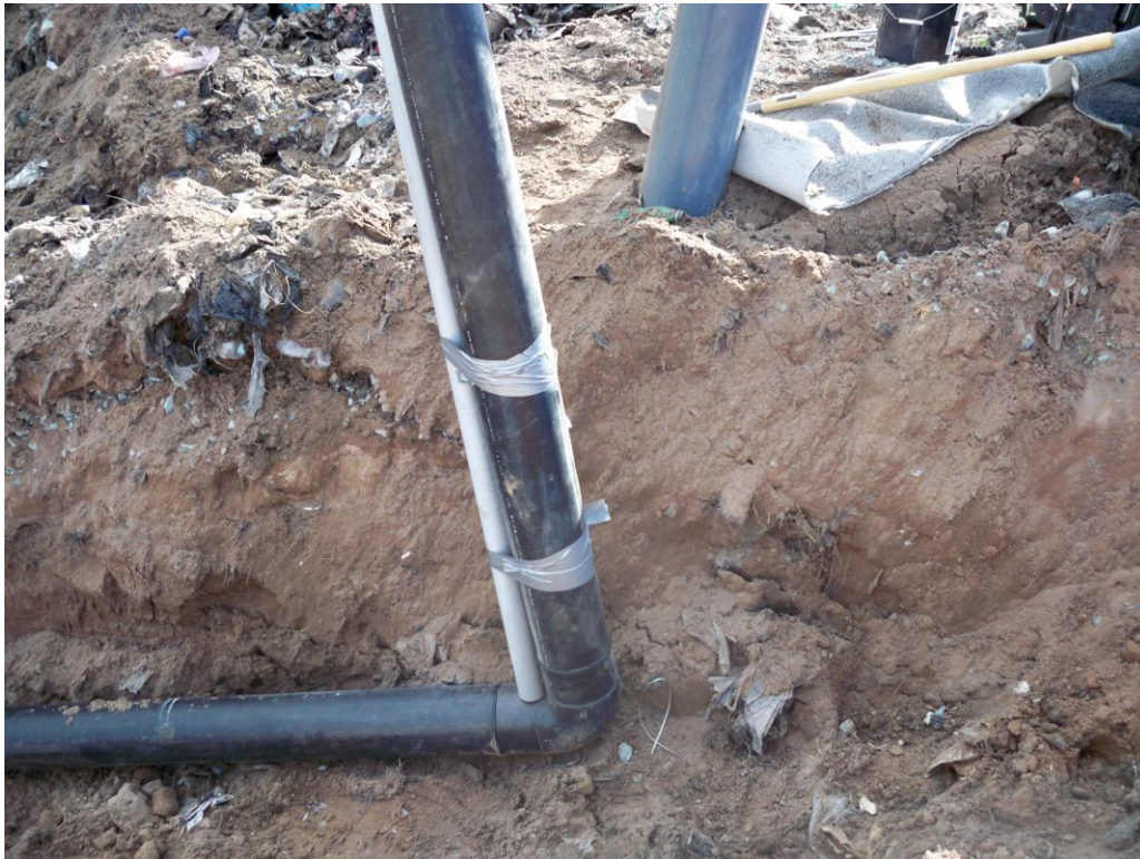
Photograph 27: Lateral riser with 90° elbow and top-of-pipe survey riser (typical).
