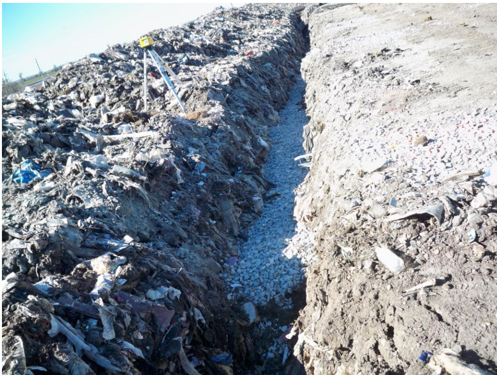
Photograph 46: Backfill HGC trench with 1-ft thick coarse stone (typical).
