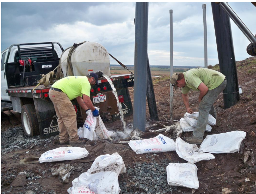
Photograph 36: Hydrating bentonite plug at extraction well (typical).
