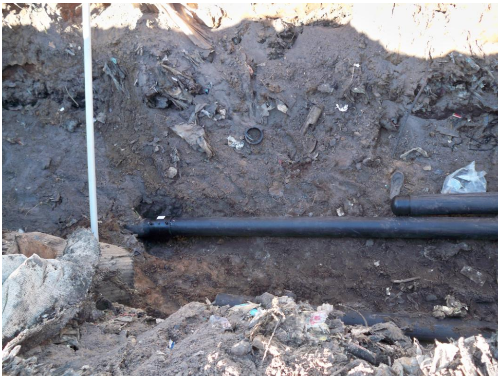
Photograph 42: Abandoned a portion of lateral GW-53 to GW-54 and replaced compromised pipe.
