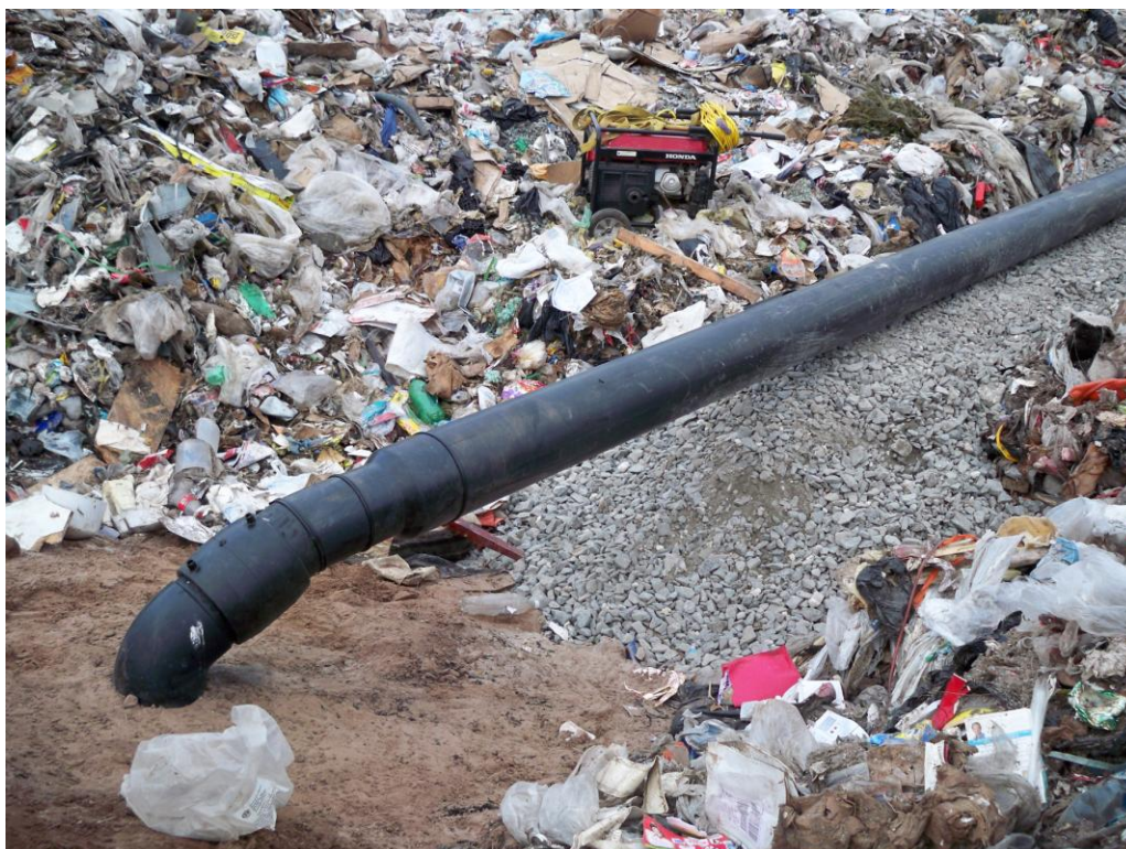
Photograph 44: HGC tie-in to 8" side-slope riser with electrofusion coupling and 8"x10 reducer.
