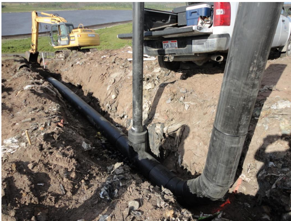
Photograph 26: 12" header in Cell 5 with 12"x6" lateral riser.
