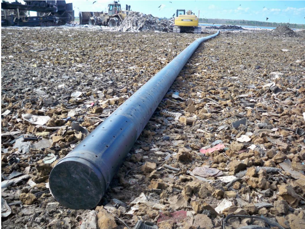
Photograph 17: 10" HDPE SDR 11 perforated pipe with end cap.
