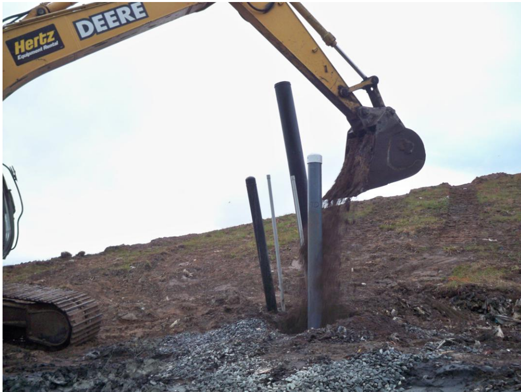
Photograph 37: Adding sandy soil backfill in between bentonite plugs (typical).
