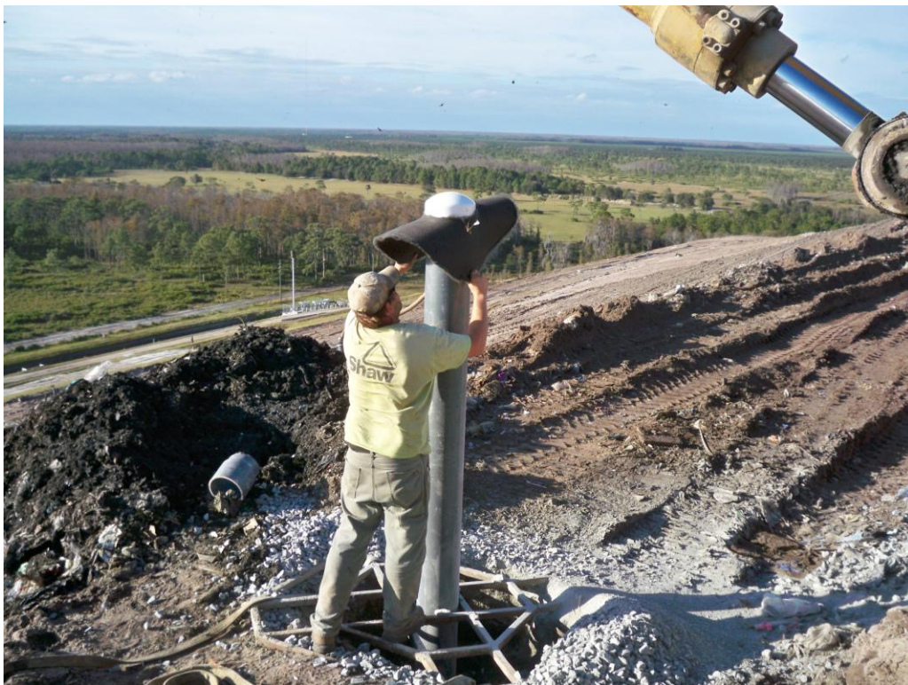
Photograph 34: Applying geotextile donut at extraction well (typical).
