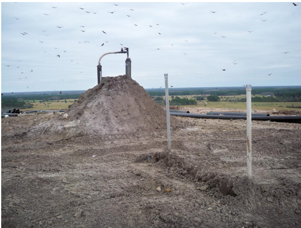
Photograph 30: Backfilled trench with survey posts every 50 'and at points of interest. Well head assembly installed with access bound (typical).
