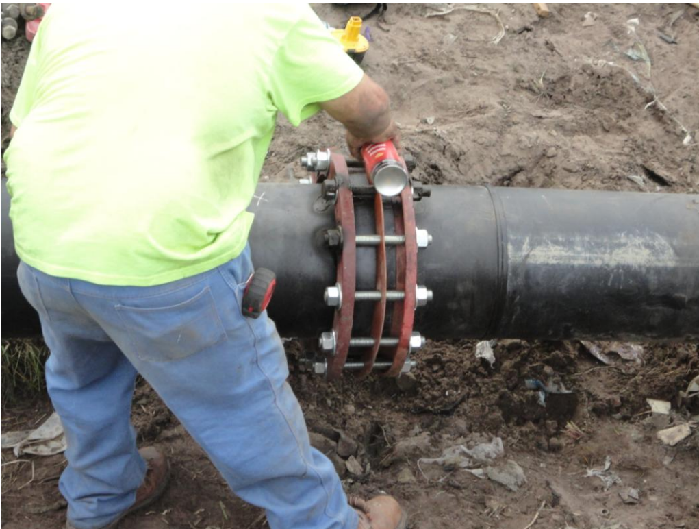
Photograph 22: Applying anti-rust spray on bolts.
