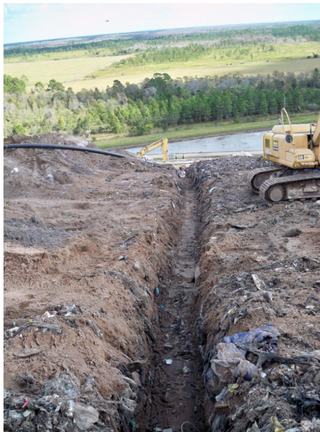
Photograph 24: Sanded trench for lateral (typical).
