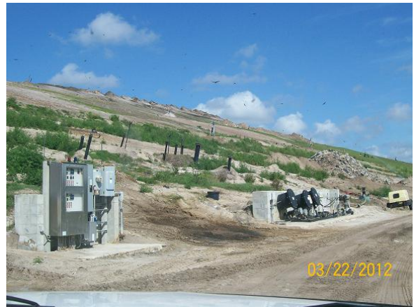
East Slope Leachate Seep Repairs
