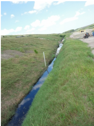
South Side Toe Drain
