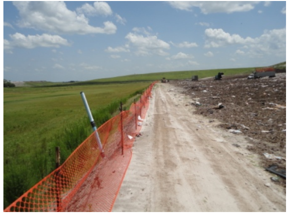
East Side Reversed Berm
