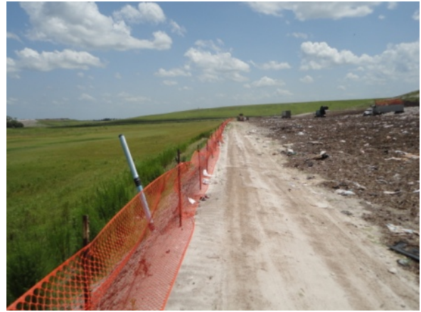
East Side Reversed Berm
