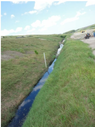
South Side Toe Drain
