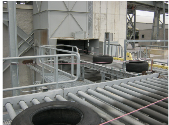
Tire conveyor to elevator
