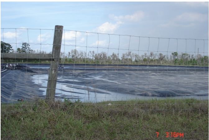
Fig 3 & 4 – Fenced Leachate Collection Pond with covers to prevent mixing of rain water with leachate.
