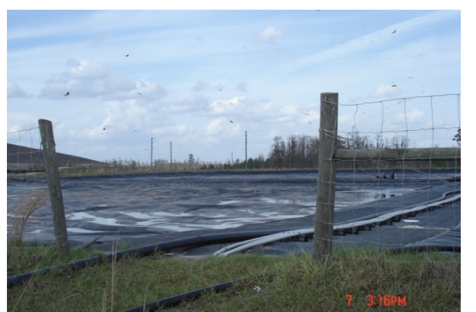
Fig 3 & 4 – Fenced Leachate Collection Pond with covers to prevent mixing of rain water with leachate.
