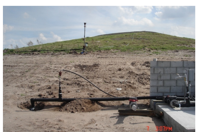
Fig. 6 – Leachate manhole replacement work in progress.
