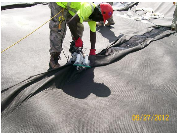
Sewing of Geocomposite
