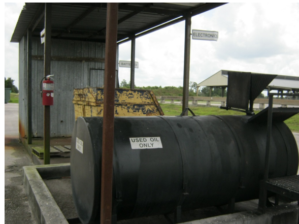
Used Oil and battery containment
