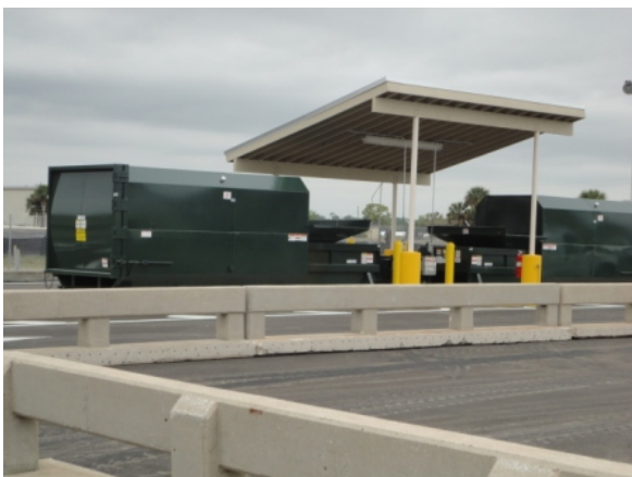
Compactors at new CDA Area
