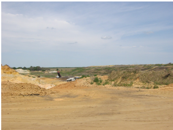
Filling new cell bottom
