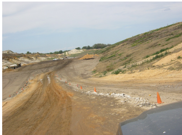
Road into new cell
