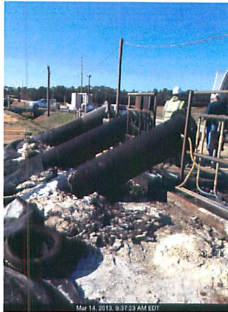
Photo 1: Date: 3/14/13 Phase 3 side slope riser pipes.
