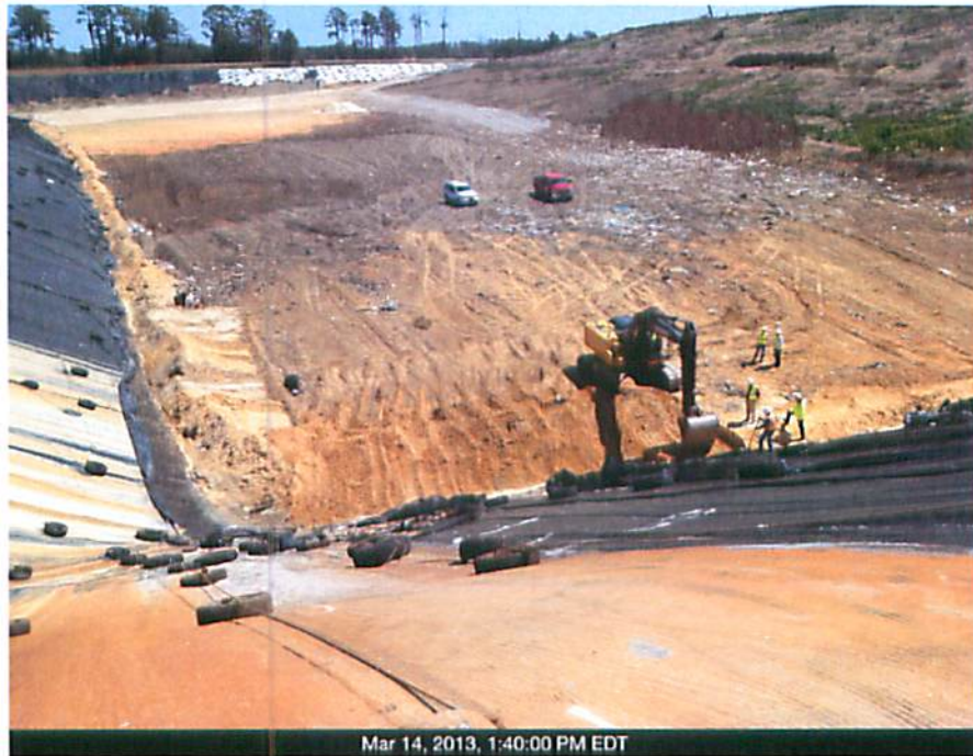
Photo 4: Date: 3/14/2013 Northwest corner of Phase 3.
