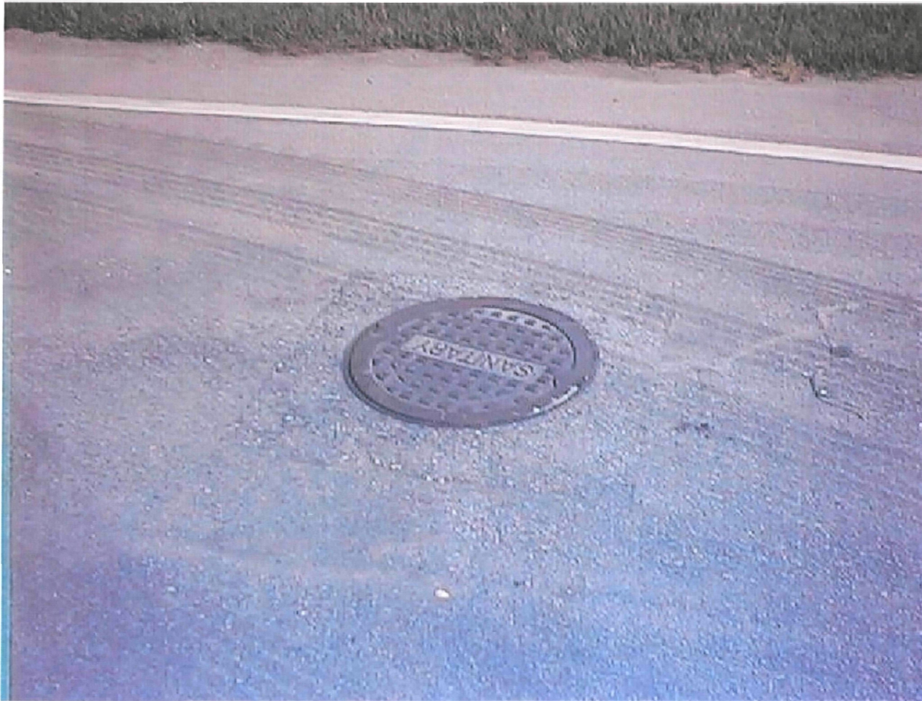
5) Paved CDA – MW-2 Manhole cover in place.
