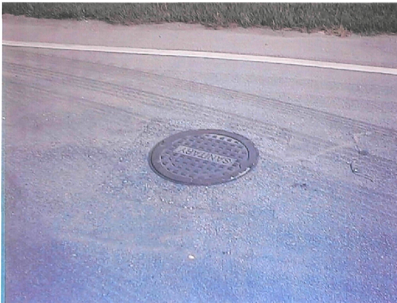
5) Paved CDA – MW-2 Manhole cover in place.
