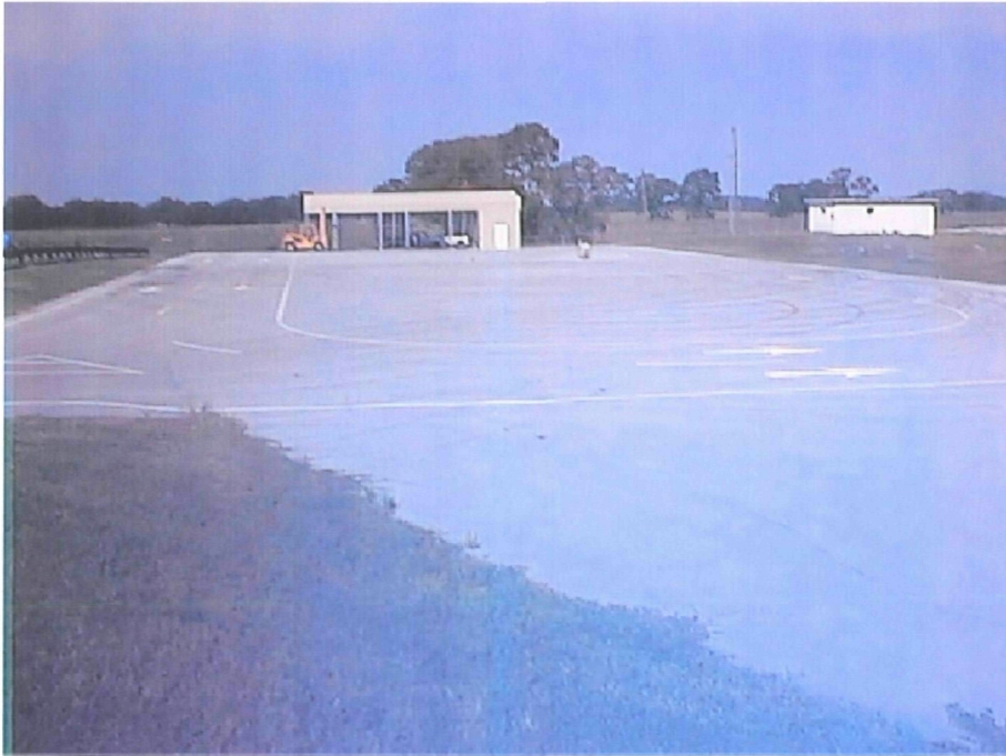
1) Looking west – Paved Community Drop-off Area (CDA) Wood Recycling Building at the far end.
