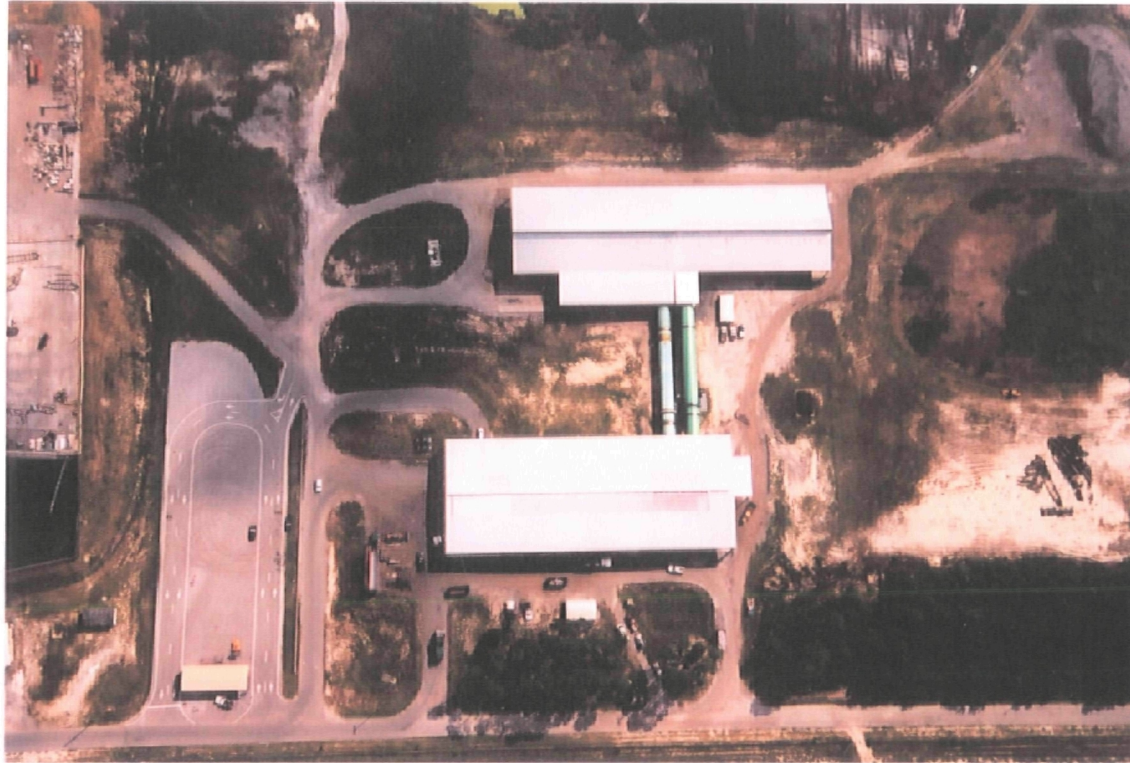
Aerial Photograph of MRF, Digester, Finish Building and Community Drop-off Area
