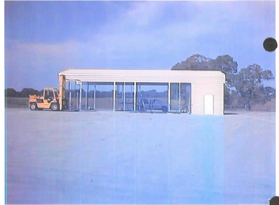
2) Wood recycling building on west end of CDA
