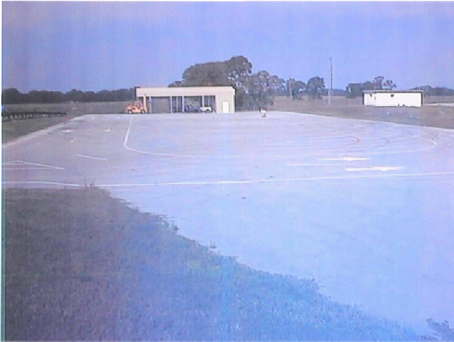
1) Looking west – Paved Community Drop-off Area (CDA) Wood Recycling Building at the far end.
