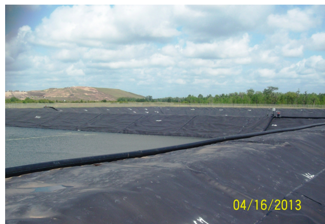
Newly Constructed Leachate Pond
