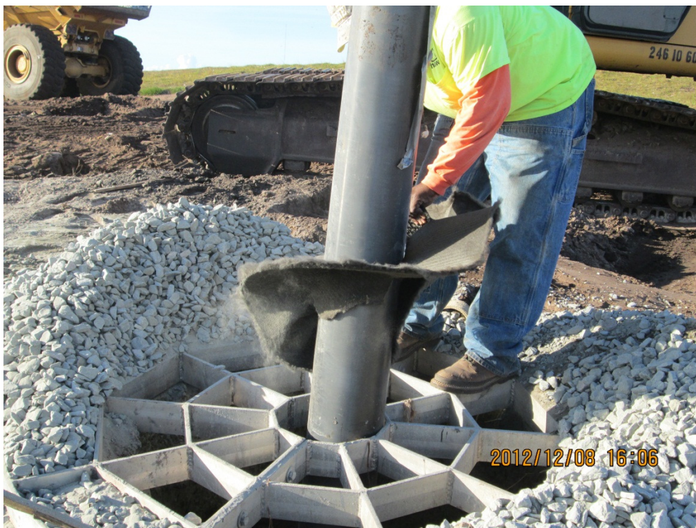
Photograph 17: Applying geotextile donut at extraction well (typical).
