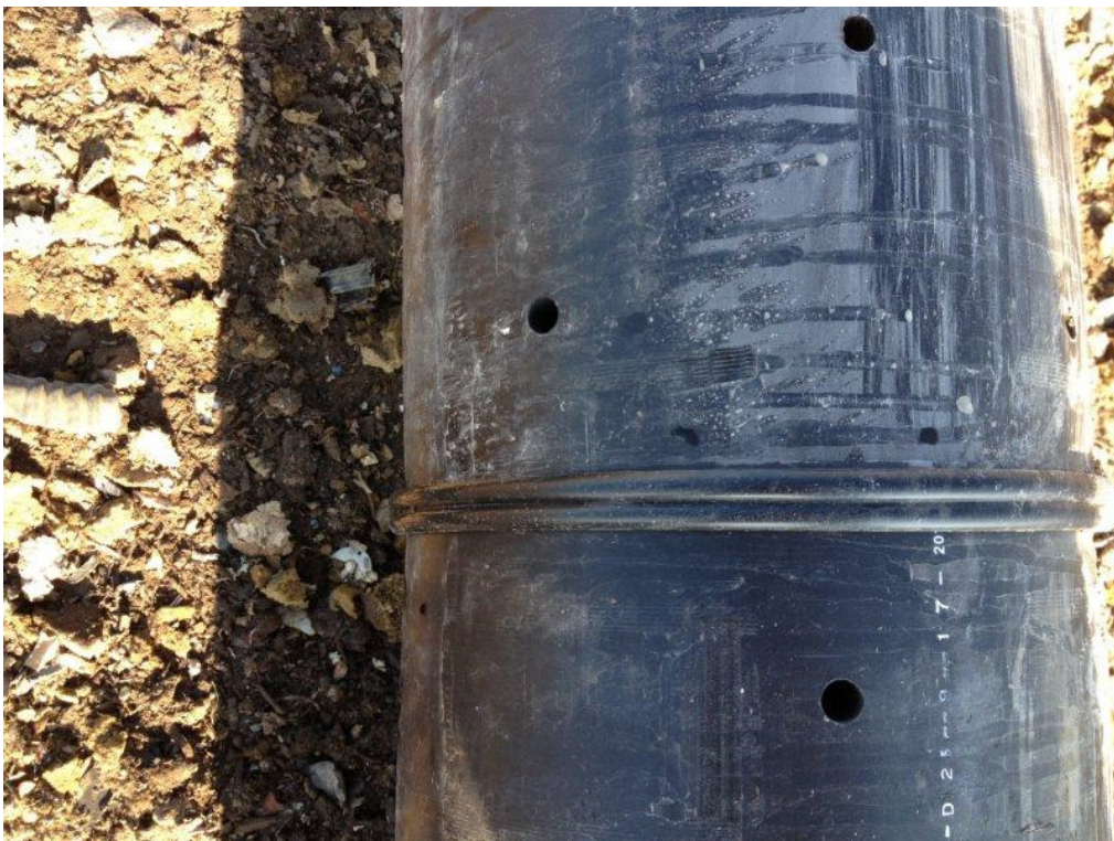
Photograph 50: 10" HDPE SDR 11 pipe weld.
