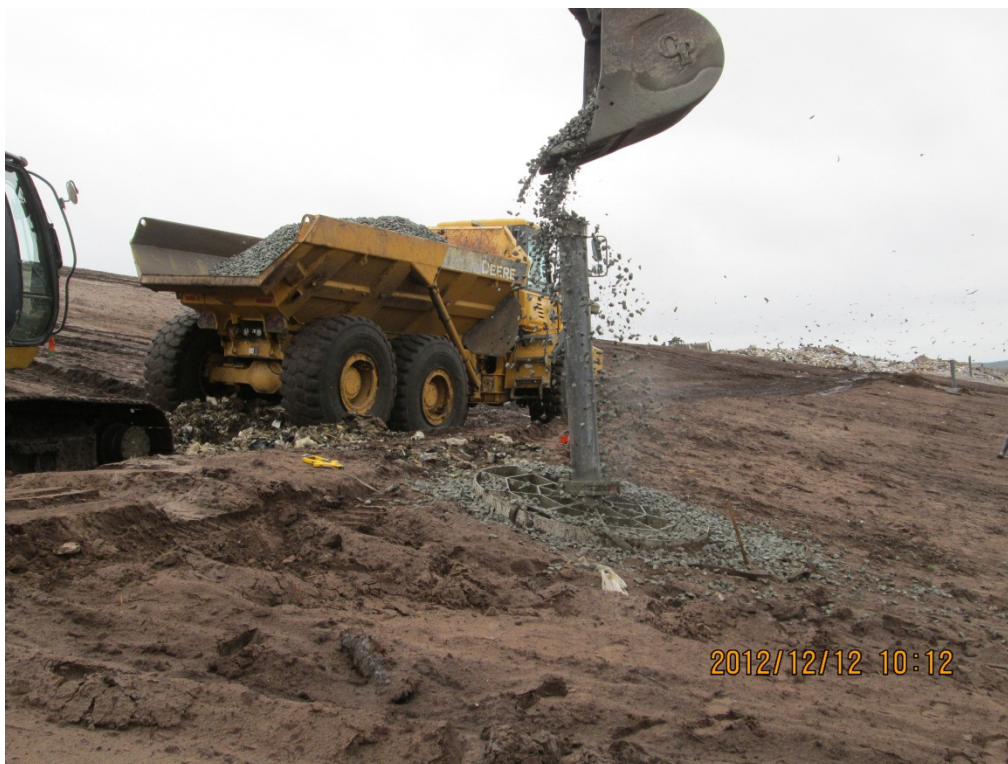
Photograph 16: Backfilling extraction well with approved stone (typical).
