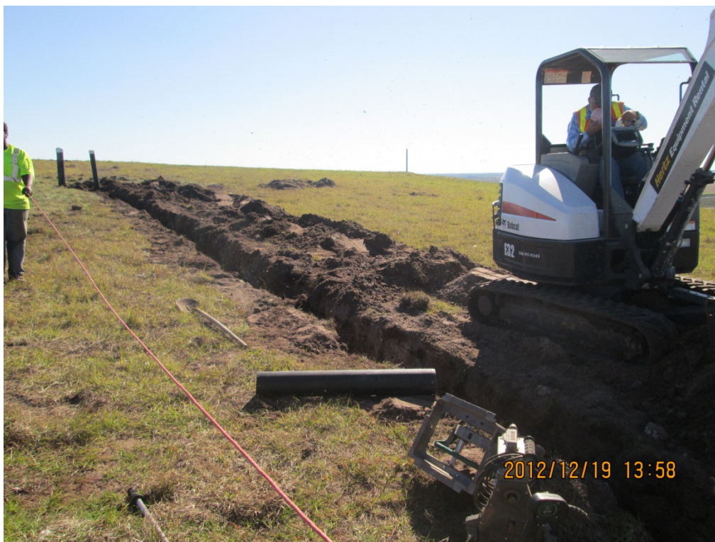
Photograph 31: Trenching with mini-excavator in capped areas to prevent damage (typical).
