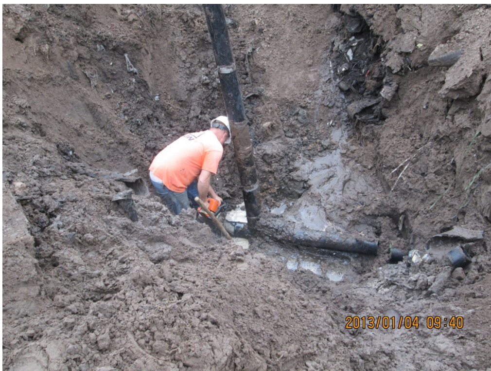
Photograph 36: Removal of existing 6" riser pipe in Cell 6.
