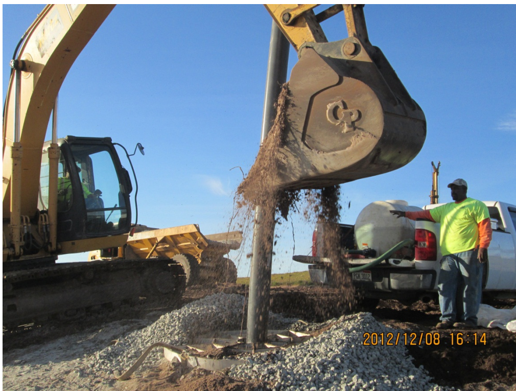
Photograph 19: Adding sandy soil backfill in between bentonite plugs (typical).
