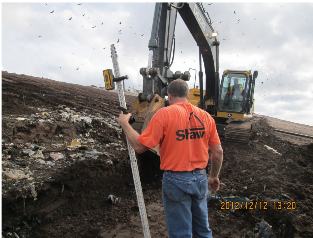
Photograph 22: Verifying minimum 5% slope for laterals and header while trenching (typical).
