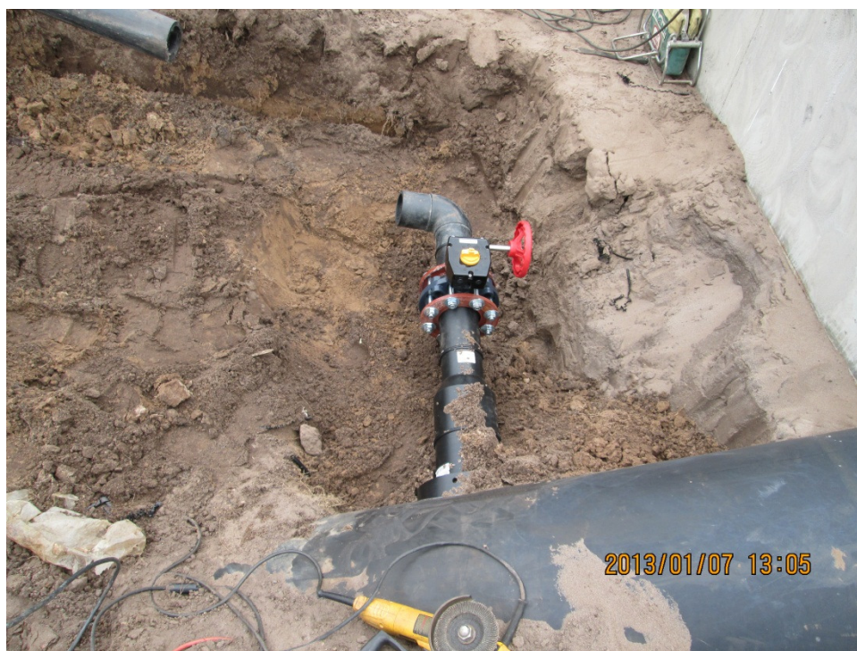
Photograph 40: 24" x 6" electro fusion saddle reduced to a 4" valve and 4" 90° elbow in Cell 7 (typical).
