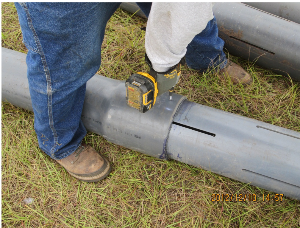
Photograph 5: 8" SCH 80 PVC 45° apart, staggered rows.
