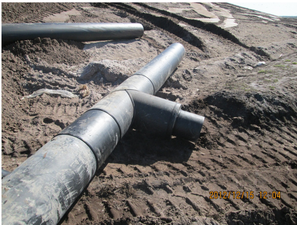
Photograph 27: 18" x 12" header reducer in Cell 8.
