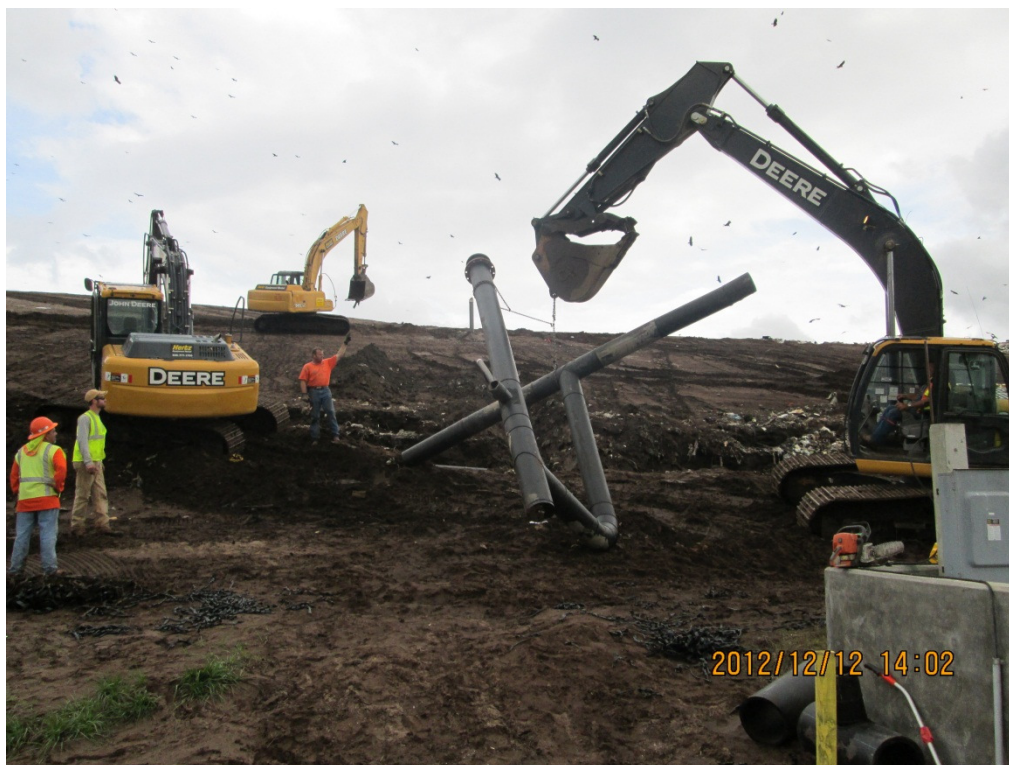
Photograph 23: Placement of pre-assembled U-trap (typical).
