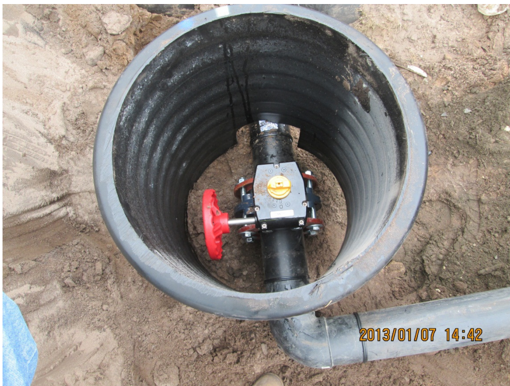
Photograph 42: 18" valve box (typical)
