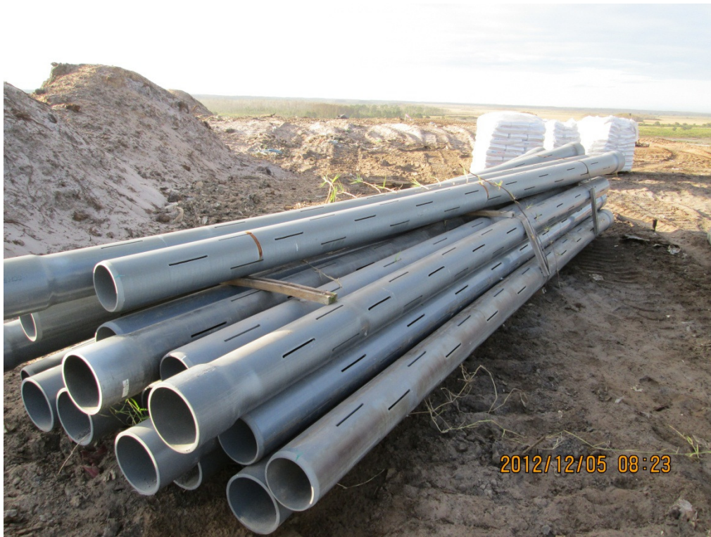
Photograph 2: 8" SCH 80 slotted PVC pipe.
