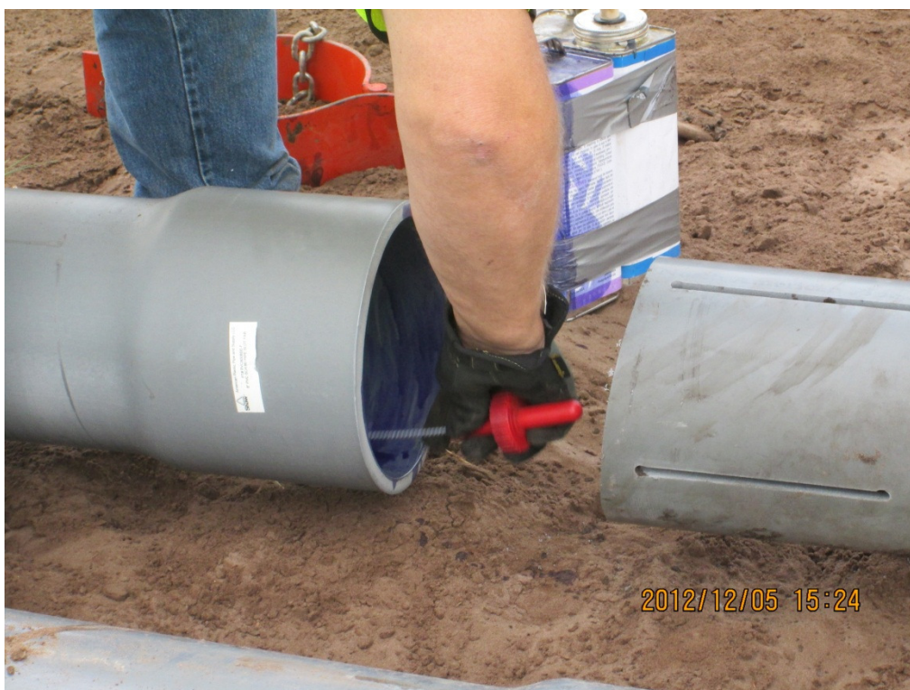
Photograph 14: Applying PVC primer and cement when joining well casing joints (typical).
