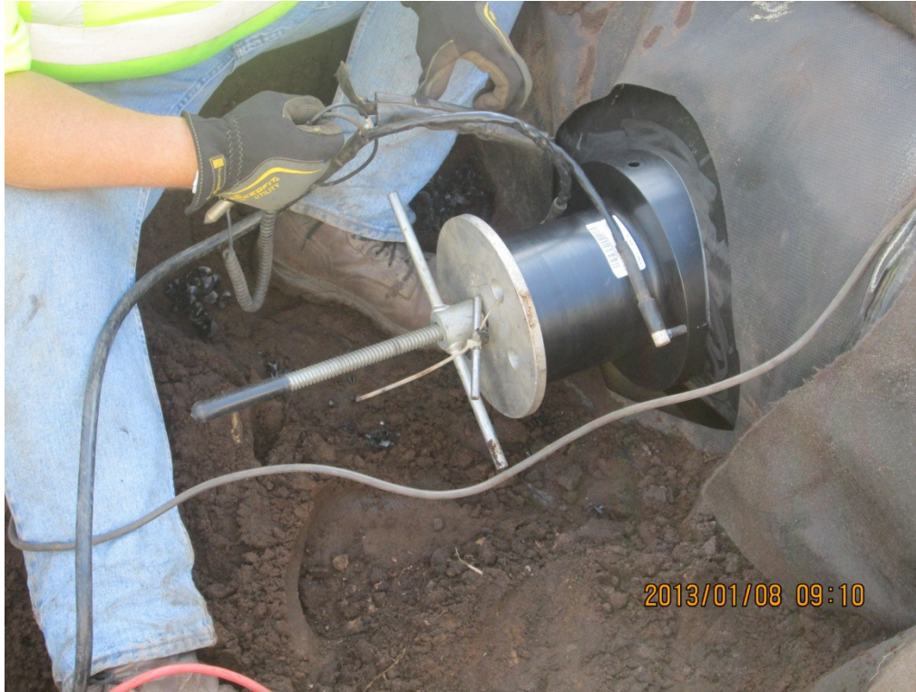
Photograph 43: Installing 24" x 6" electro fusion saddle on 24" primary sump in Cell 8 (typical).
