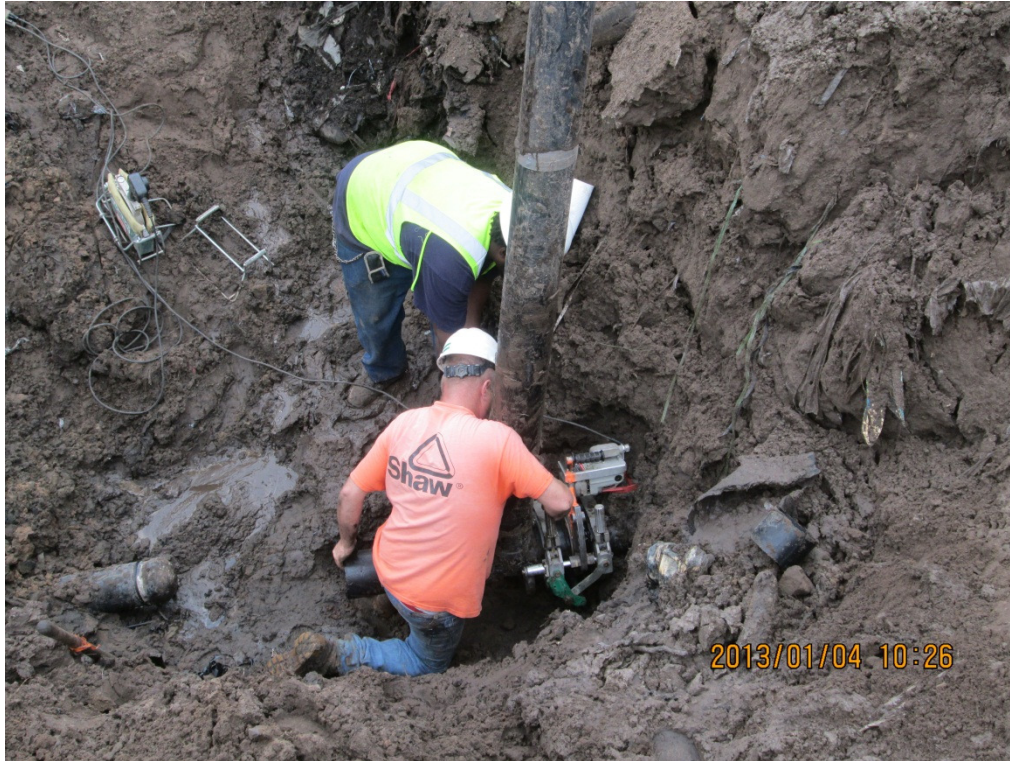
Photograph 37: Capping and abandoning existing 6" line and relocating 6" riser pipe in Cell 6.
