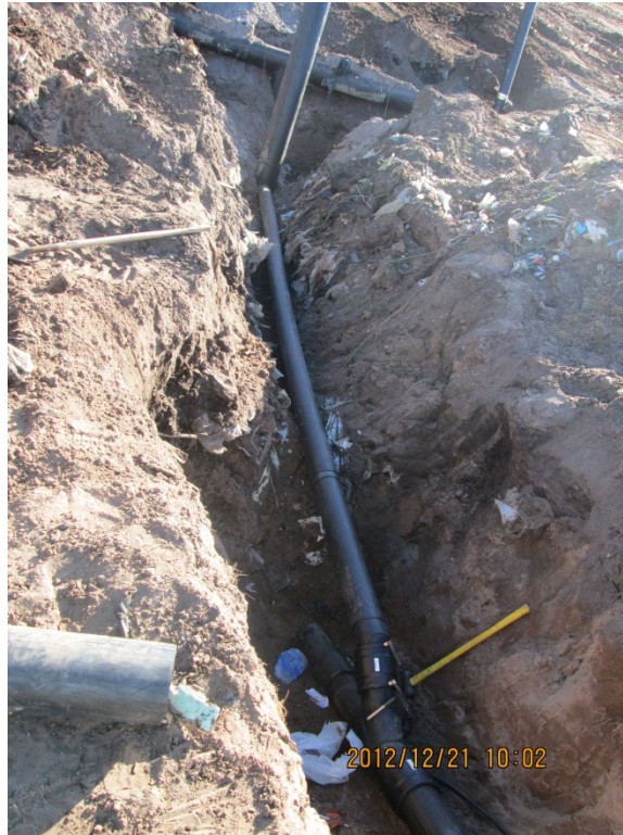
Photograph 33: U-trap drain line tie-in to existing 6" cleanout in Cell 7 (typical).
