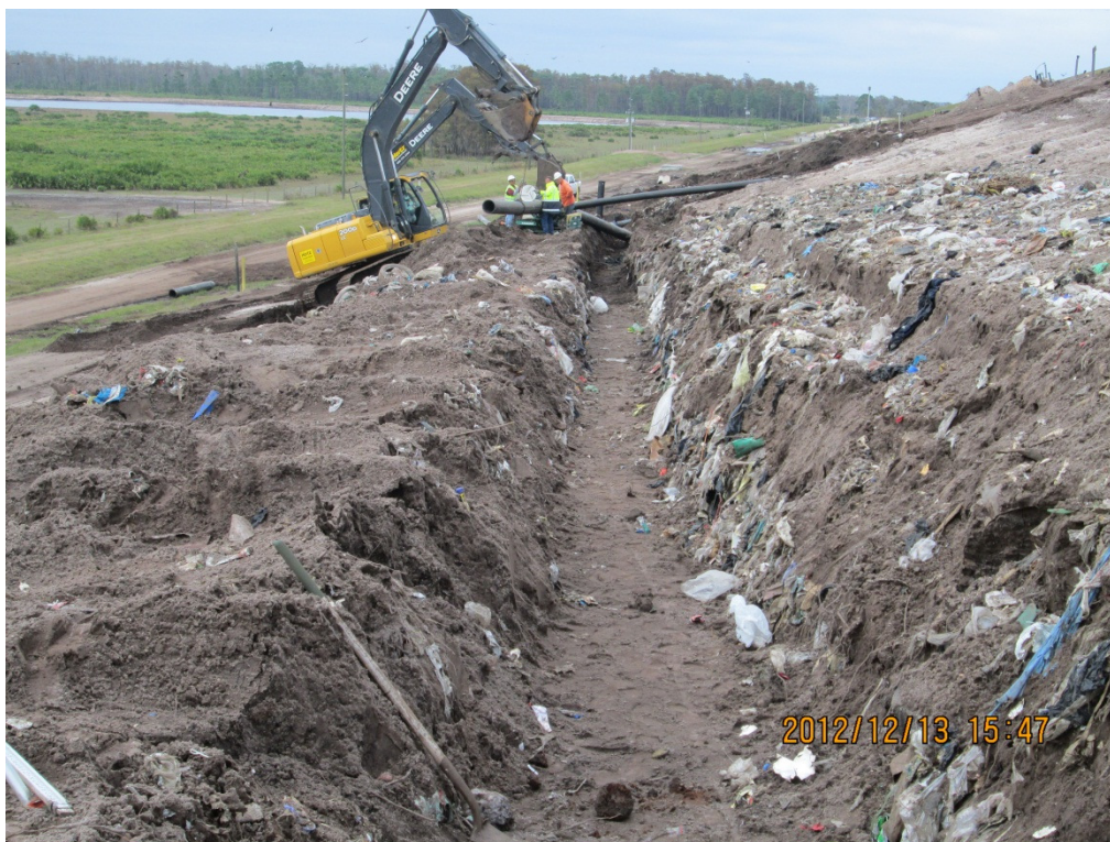
Photograph 13: Standard trench for lateral (typical).
