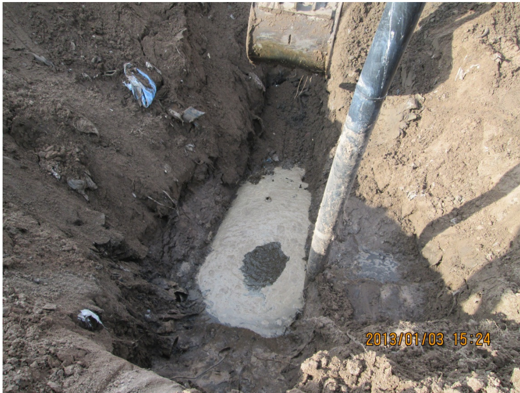
Photograph 35: Leachate infiltration in Cell 6.
