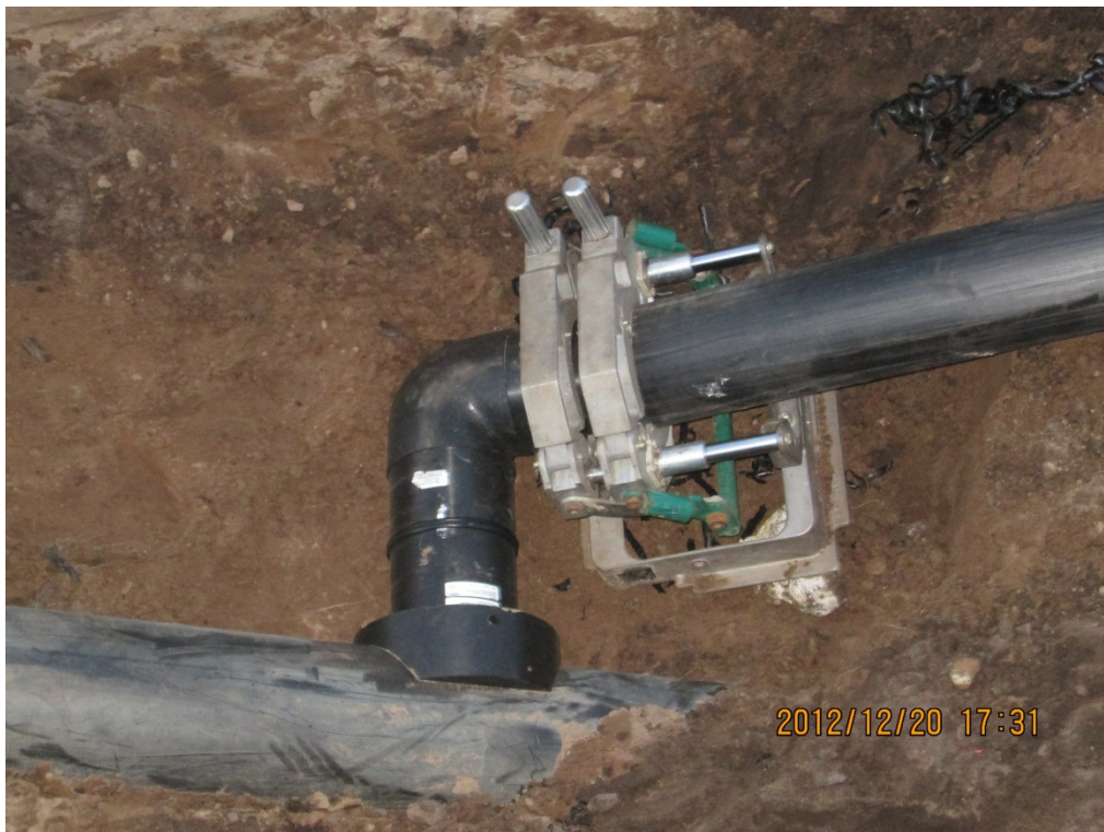
Photograph 34: 6" lateral tie-in to existing horizontal gas collector (typical).
