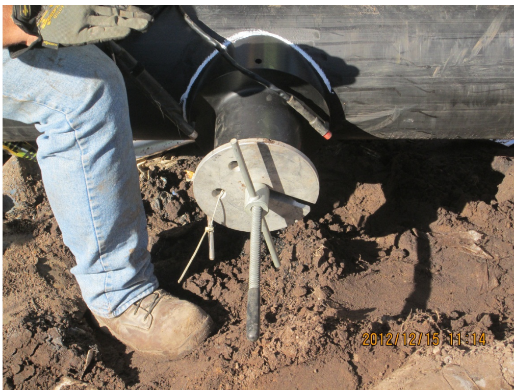
Photograph 28: Installation of 12" x 6" electro fusion saddle for horizontal gas collector lateral tie-in in Cell 7 (typical).
