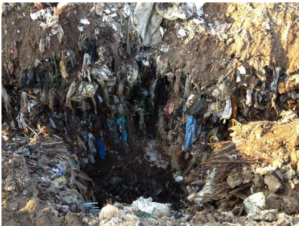
Photograph 48: Excavation hole for sumps at low points along HGC (typical).
