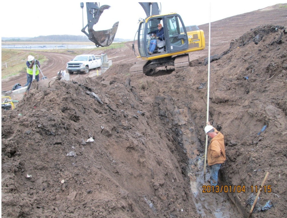
Photograph 39: Verifying sufficient below ground fall while trenching in Cell 6 (typical).
