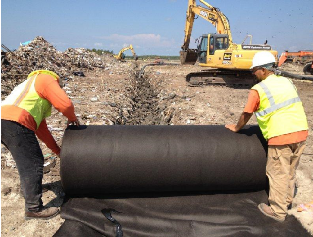
Photograph 53: Placing filter fabric over tire chips and HGC piping (typical).
