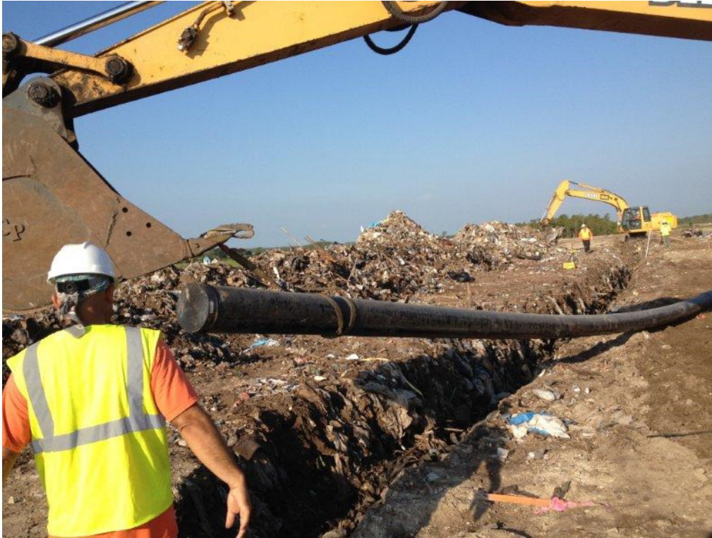
Photograph 51: Placing horizontal gas collector into excavated trench (typical).
