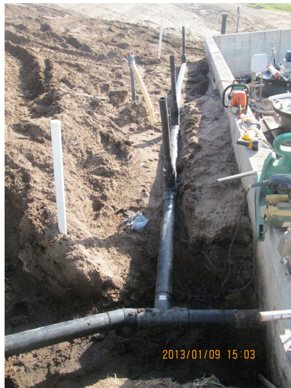
Photograph 44: 4" lateral with 2" risers to tie-in 1 existing 2" PVC well and 2 new 2" PVC wells in Cell 5.
