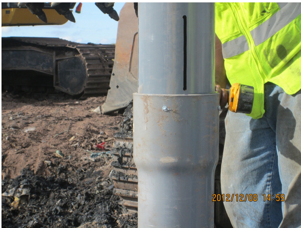
Photograph 15: Lag bolting joints to provide additional support (typical).
