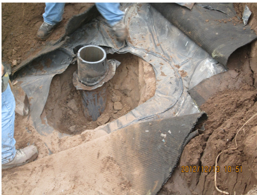
Photograph 24: Cutting and capping abandoned well casing minimum 1' below liner (typical).
