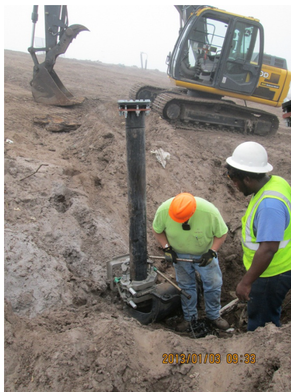
Photograph 32: 12" x 6" electro fusion saddle with riser for clean out at U-trap in Cell 7 (typical).
