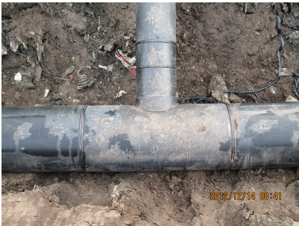
Photograph 20: 6" lateral tie-in to 12" header in Cell 7 (typical).
