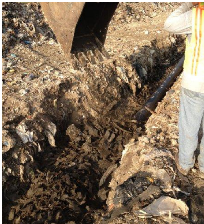
Photograph 52: Covering HGC pipe with tire chips (typical).
