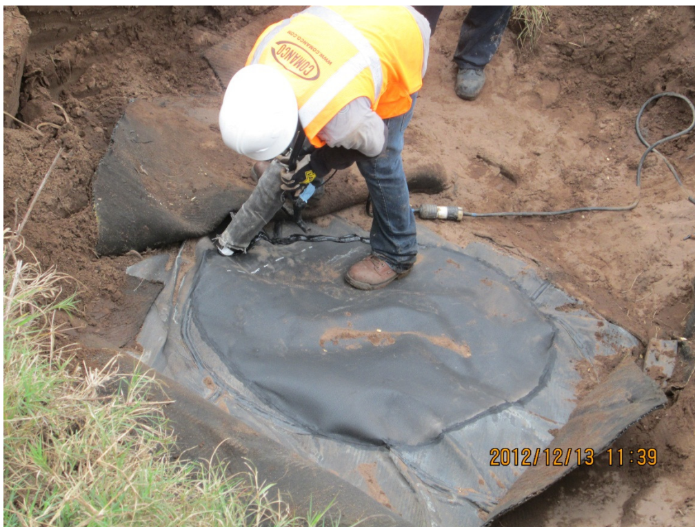
Photograph 25: Repairing liner over abandoned well casing (typical).
