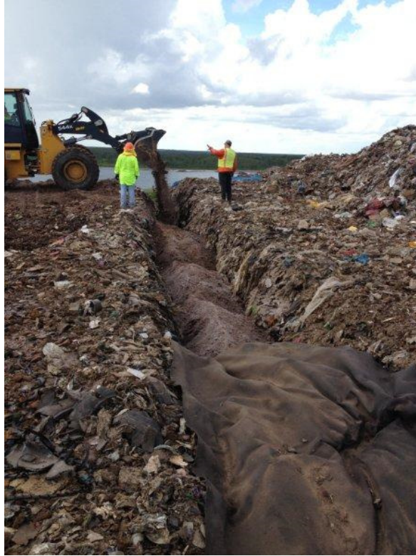
Photograph 55: Covering solid pipe sections of HGC with clean fill (typical).
