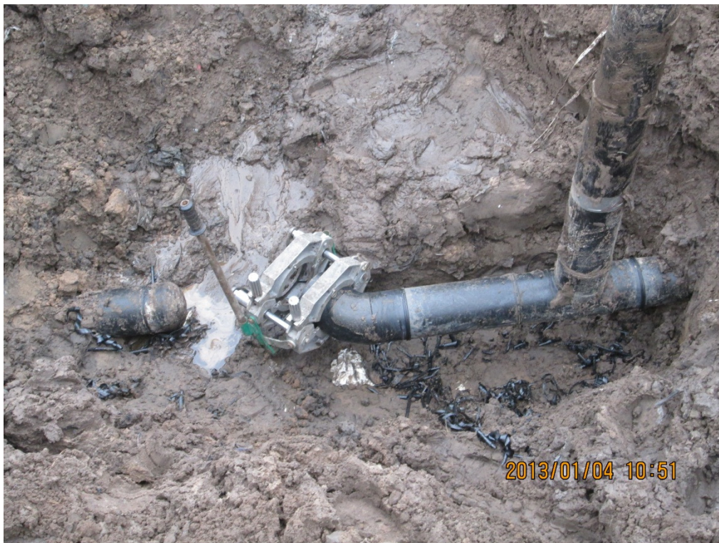
Photograph 38: 6" HDPE 45° elbow to re-route U-trap drain line towards 24" primary sump in Cell 6.
