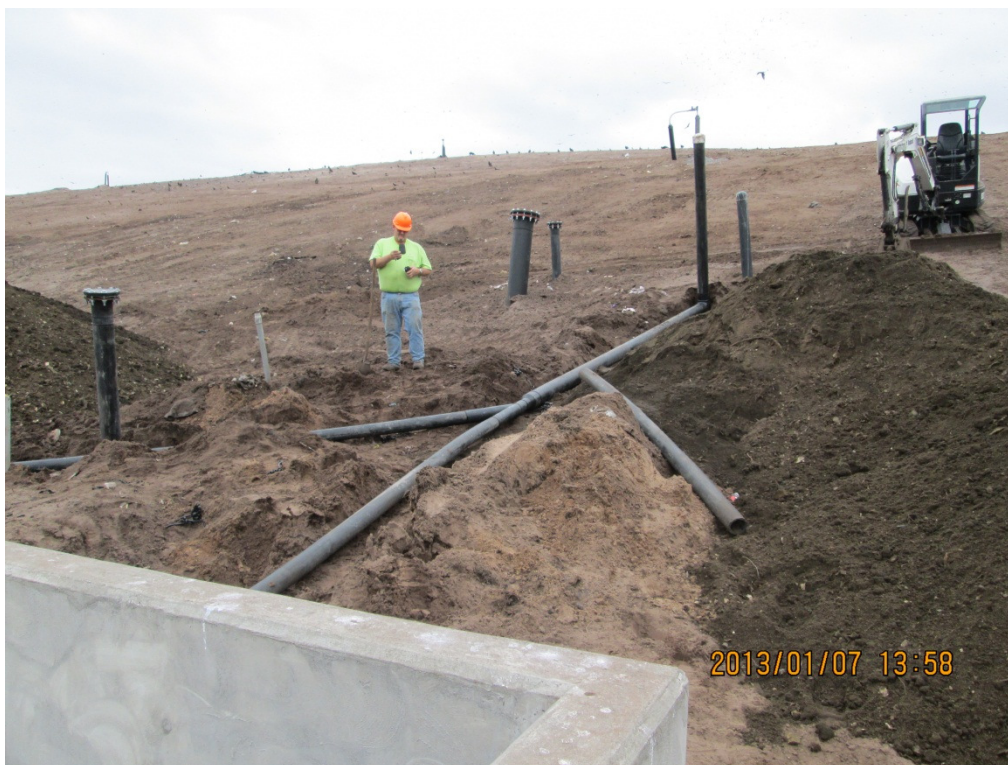
Photograph 41: 4" Laterals increasing to 6" HDPE SDR 17 with a vertical riser in Cell 7 (typical).
