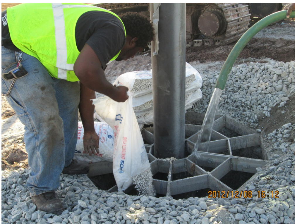
Photograph 18: Hydrating bentonite plug at extraction well (typical).
