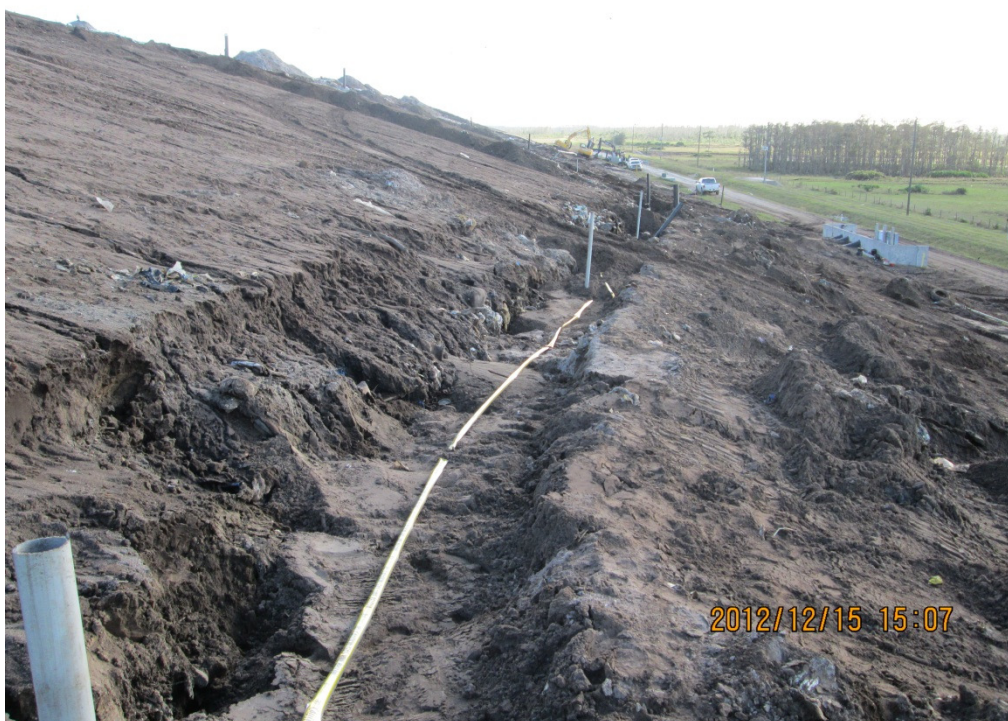
Photograph 21: Backfilled trench. Caution tape applied and survey posts every 50' and at points of interest (typical).
