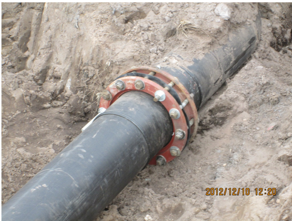
Photograph 11: Tie-in to existing gas conveyance header.
