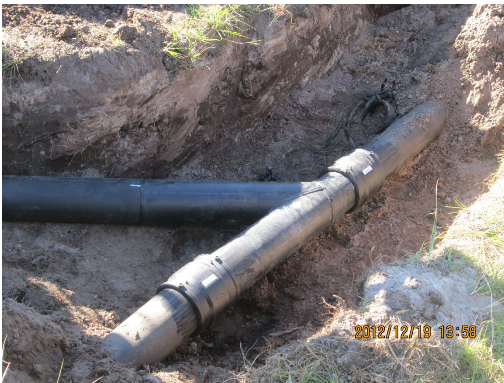
Photograph 30: Tie-in to existing 6" lateral for well GW-28B in capped area of landfill.
