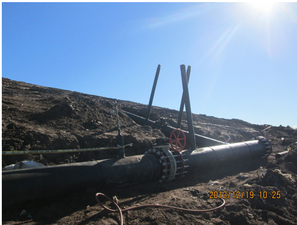
Photograph 29: 18" and 12" valves and blind flanges in Cell 8 for future expansion.
