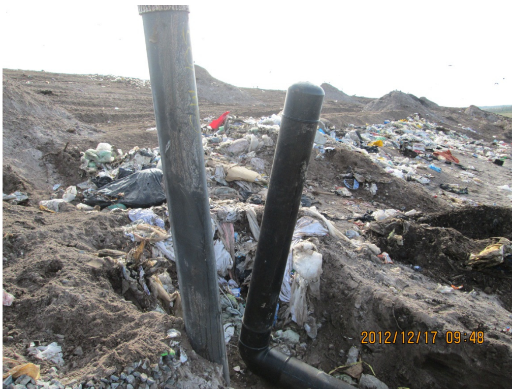
Photograph 26: 90° 6" elbow with riser for wellhead vacuum source (typical).
