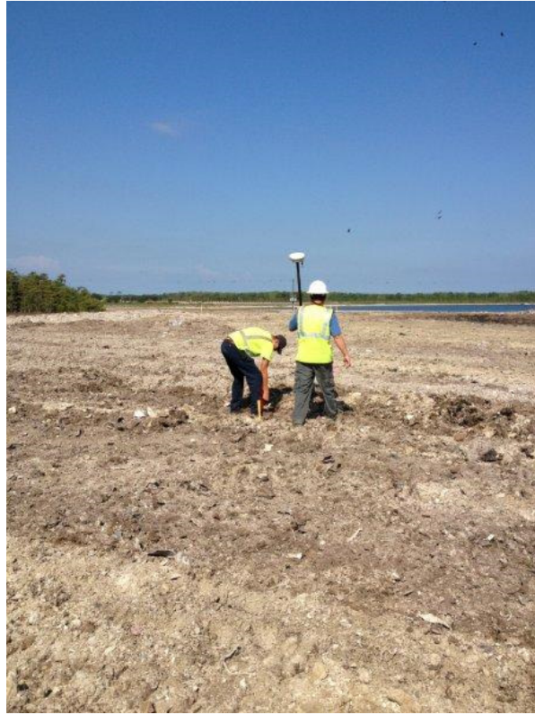
Photograph 45: WSI crew staking horizontal gas collector (HGC) locations.
