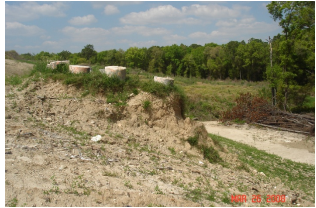
Fig 2. - Location of MW-4 that will be abandoned. Mild Erosion noted to the eastern side of MW-4
