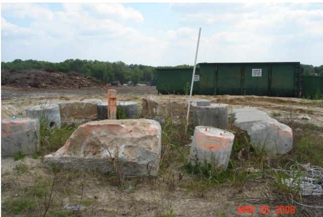
Fig - 5 Monitoring well MW-2 that will be abandoned
