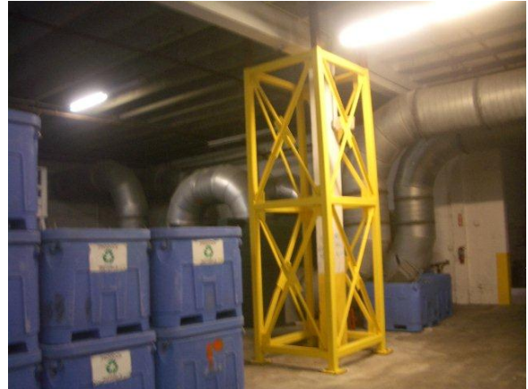
damaged column repair work
