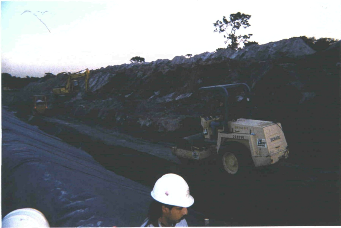
COMPACTING COVER SOIL
