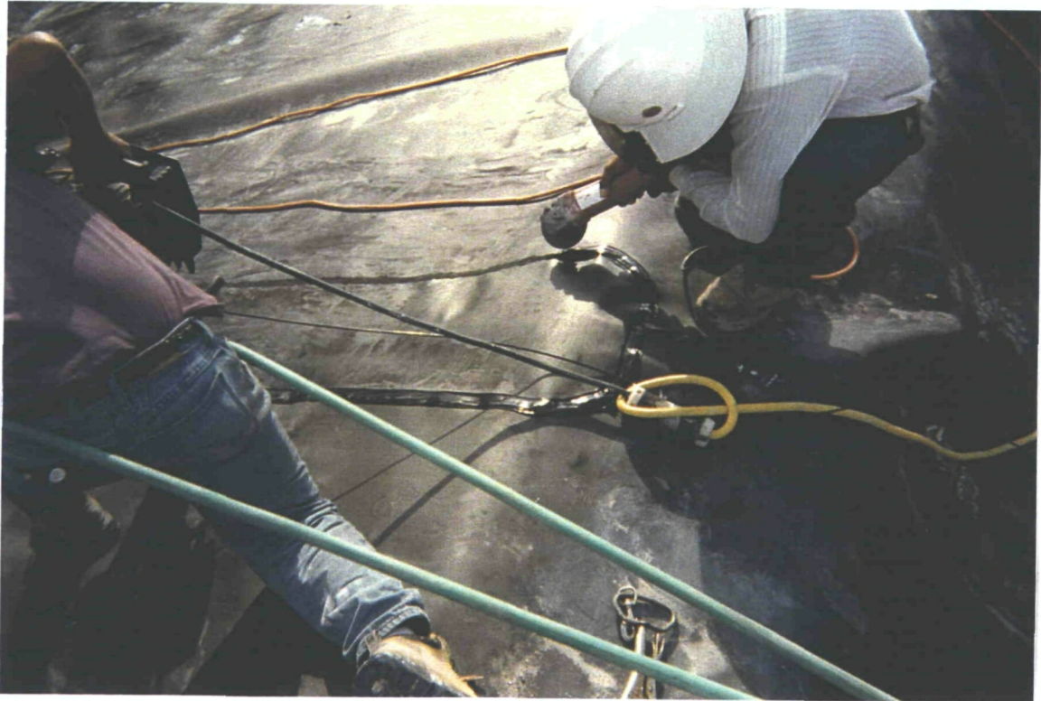
REPAIRING PATCH UTILIZING EXTRUDE WELDING
