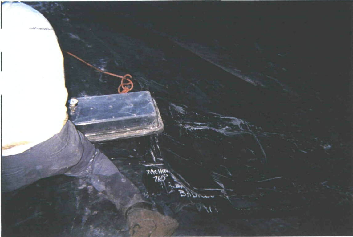
VACUUM TESTING REPAIR
