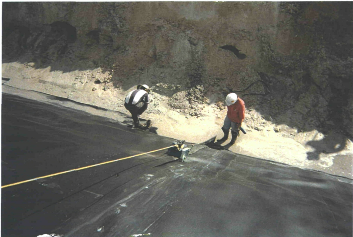
FUSION WELDING SEAM ON ADJACENT PANELS
