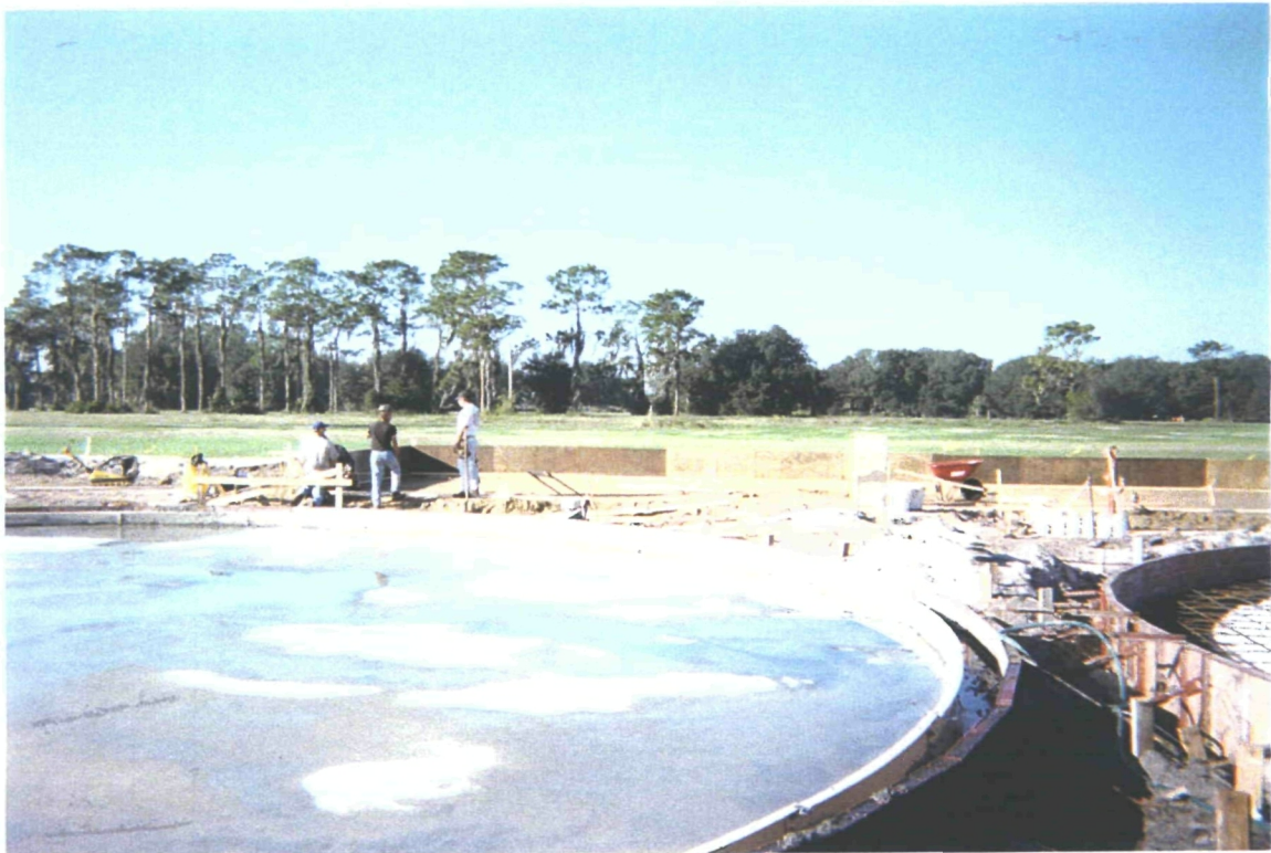
LEACHATE STORAGE TANK CONCRETE SLAB
