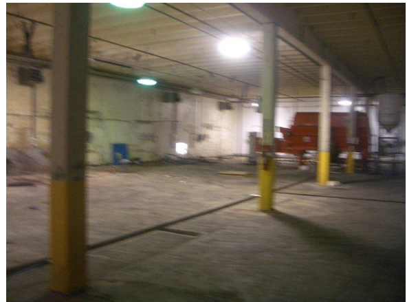
dismantled process area
