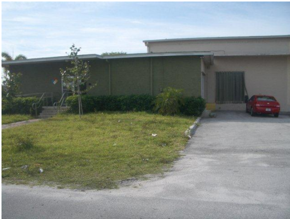
North end of facility
