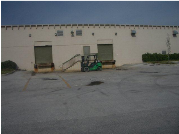
East side of facility
