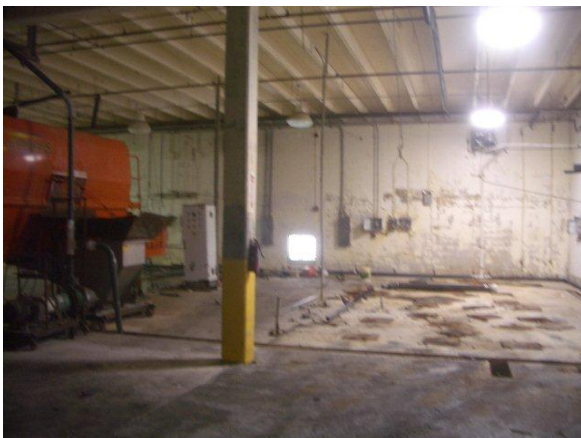
dismantled process area
