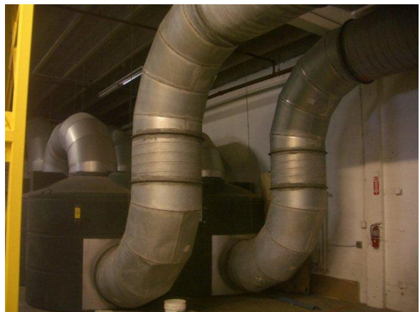
process exhaust system
