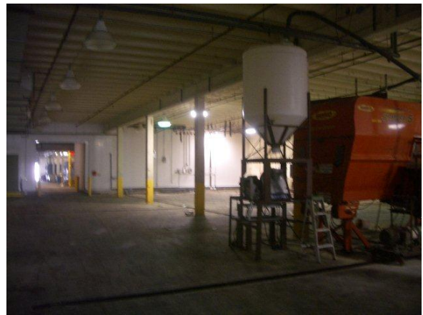
remaining process equipment
