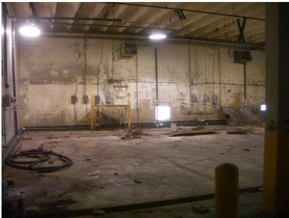
dismantled process area
