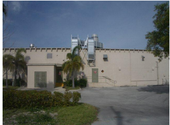
East side of facility
