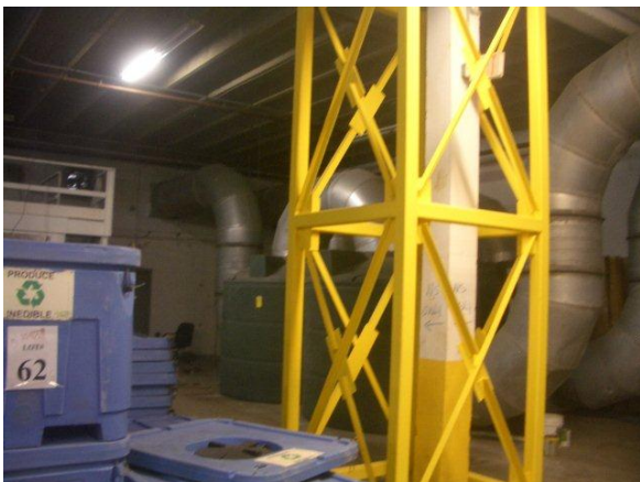
repaired roof support column
