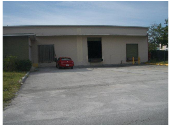
North end of facility
