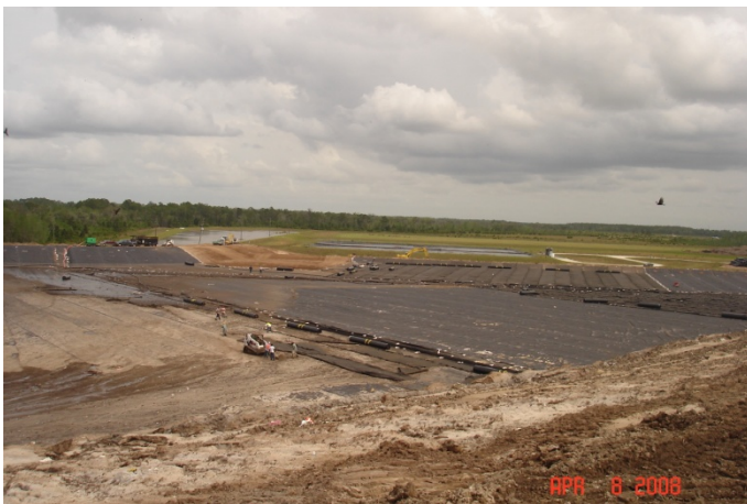
Fig. 5 – Liner Installation activities
