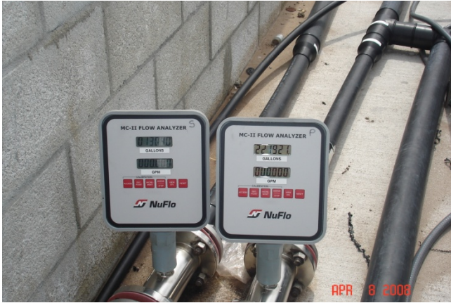
Fig. 1 - Cell 1 Replaced Totalizer
