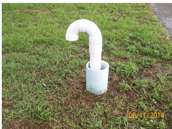
Gas Vent on West Side of Asphalt
