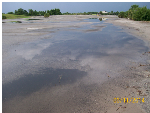
Asphalt Cover Ponding
