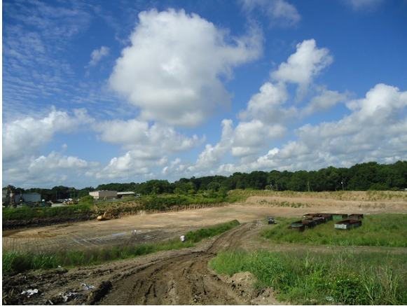
Construction of Cell 2
