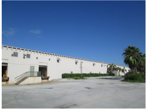
east side building
