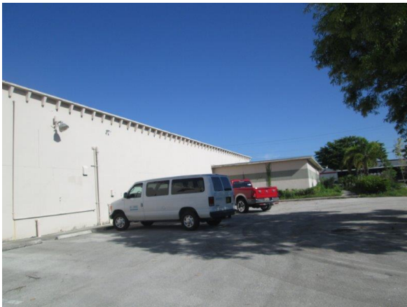
east side building
