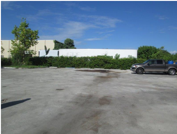
south end of facility
