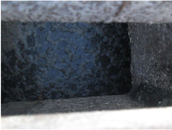
inside storm drain
