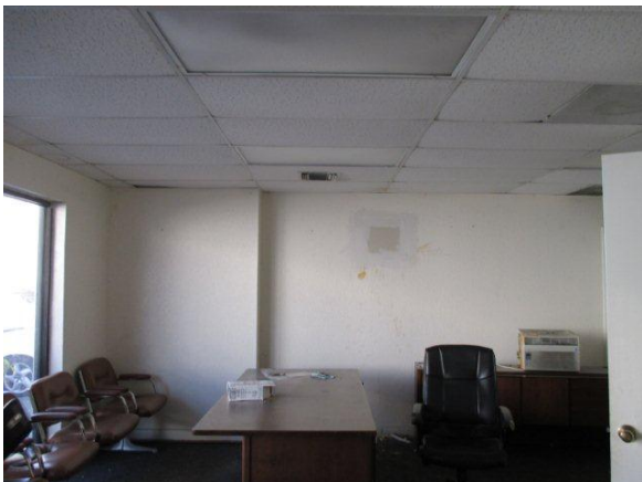
interior office to be removed
