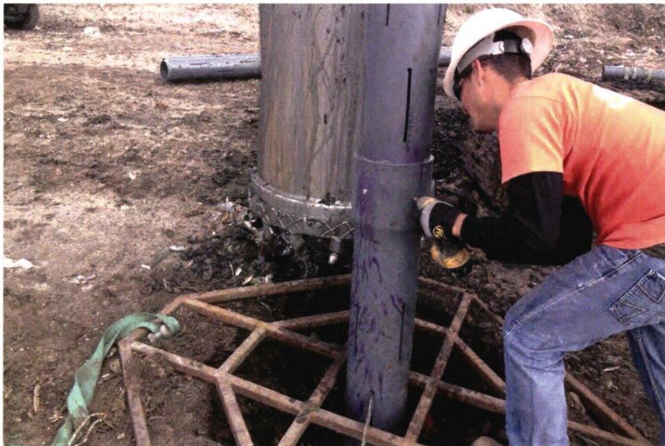
Photograph 8: Lag bolting joints to provide additional support (typical).
