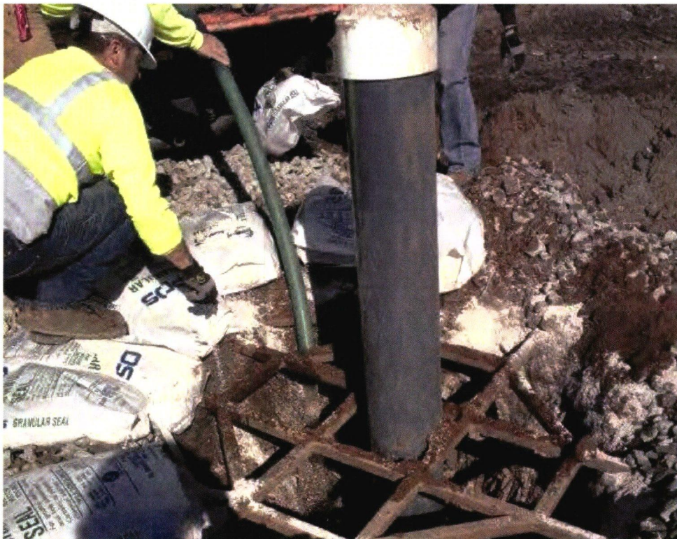
Photograph 10: Hydrating bentonite plug at extraction well (typical).
