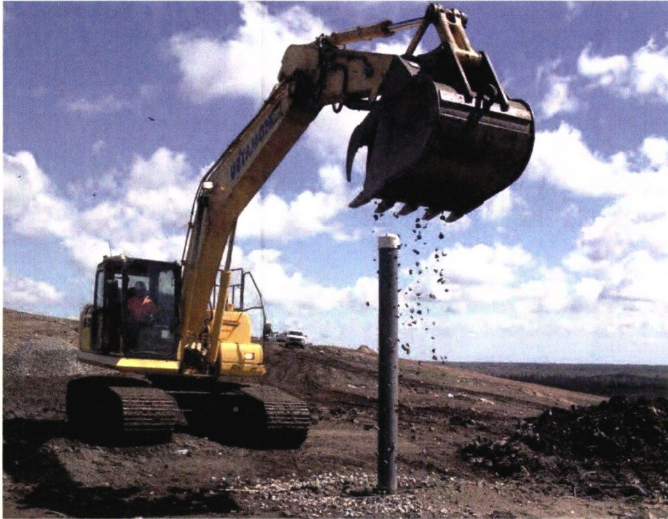
Photograph 9: Backfilling extraction well with approved stone (typical).
