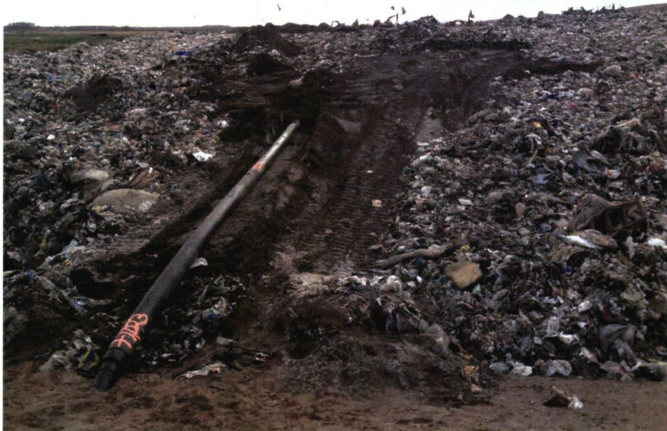
Photograph 43: Covering solid pipe sections of HGC with clean fill (typical).
