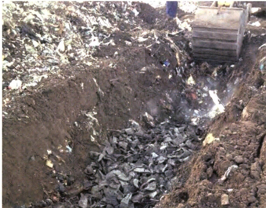
Photograph 35: Tire chips used for drainage fill in HGC trenches (typical).
