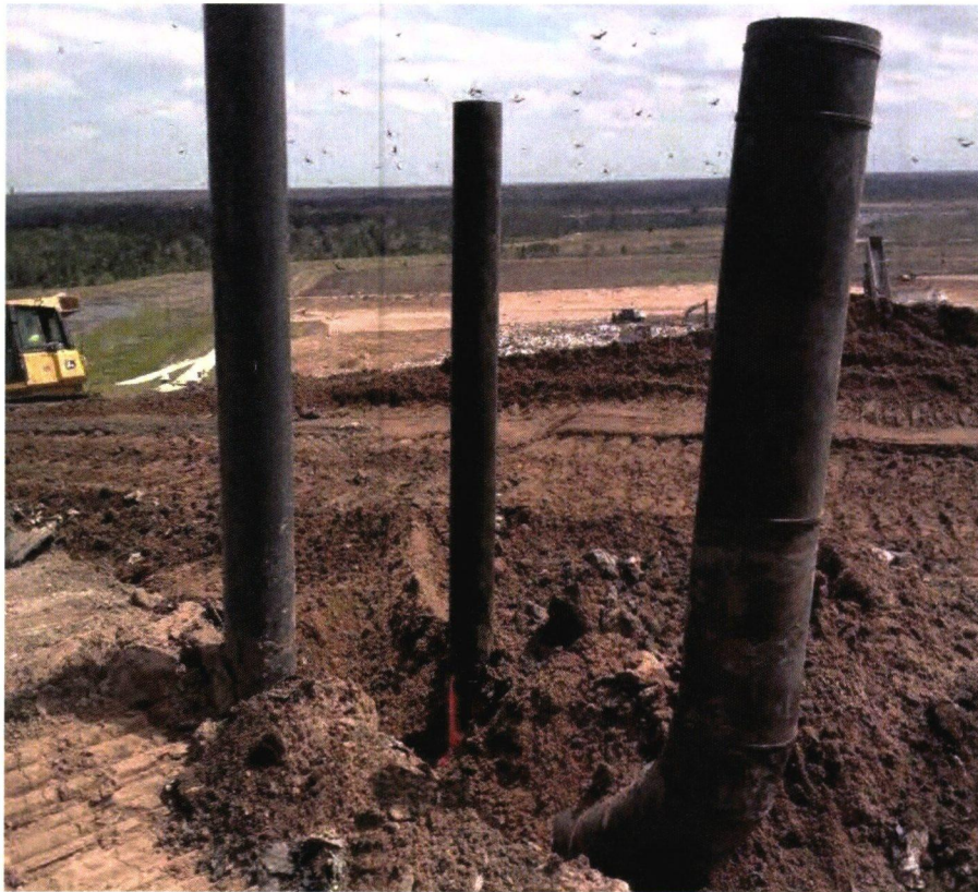
Photograph 30: New 12" subheader riser at GW-71.
