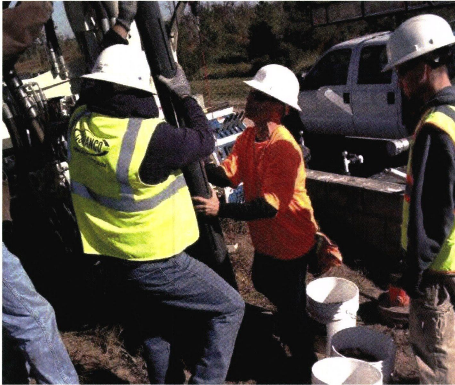
Photograph 46: Installing 4-inch SCH 80 PVC through center of auger bit (typical).
