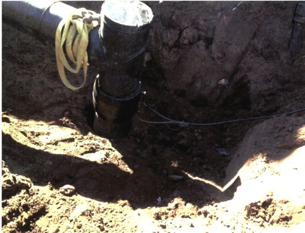
Photograph 17: Electrofusion for 12" subheader tie-in at GW-89.
