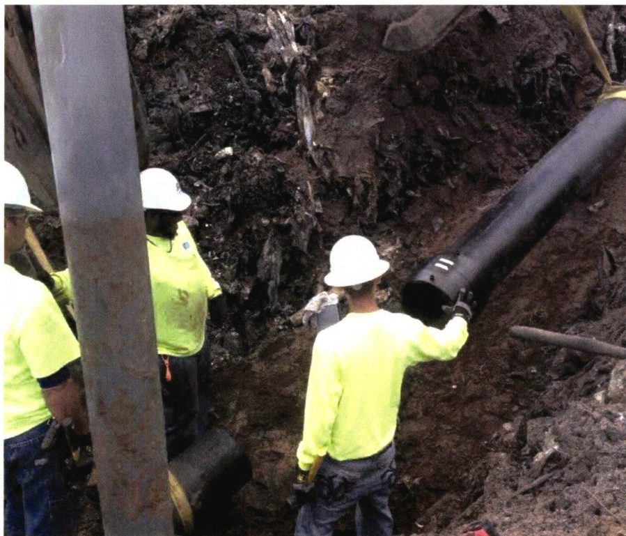
Photograph 29: Subheader tie-in at GW-70.
