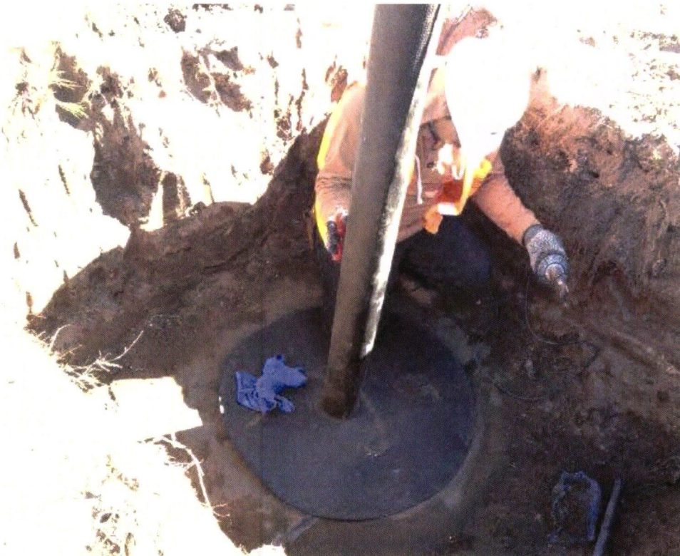
Photograph 49: Comanco repairing liner (typical).
