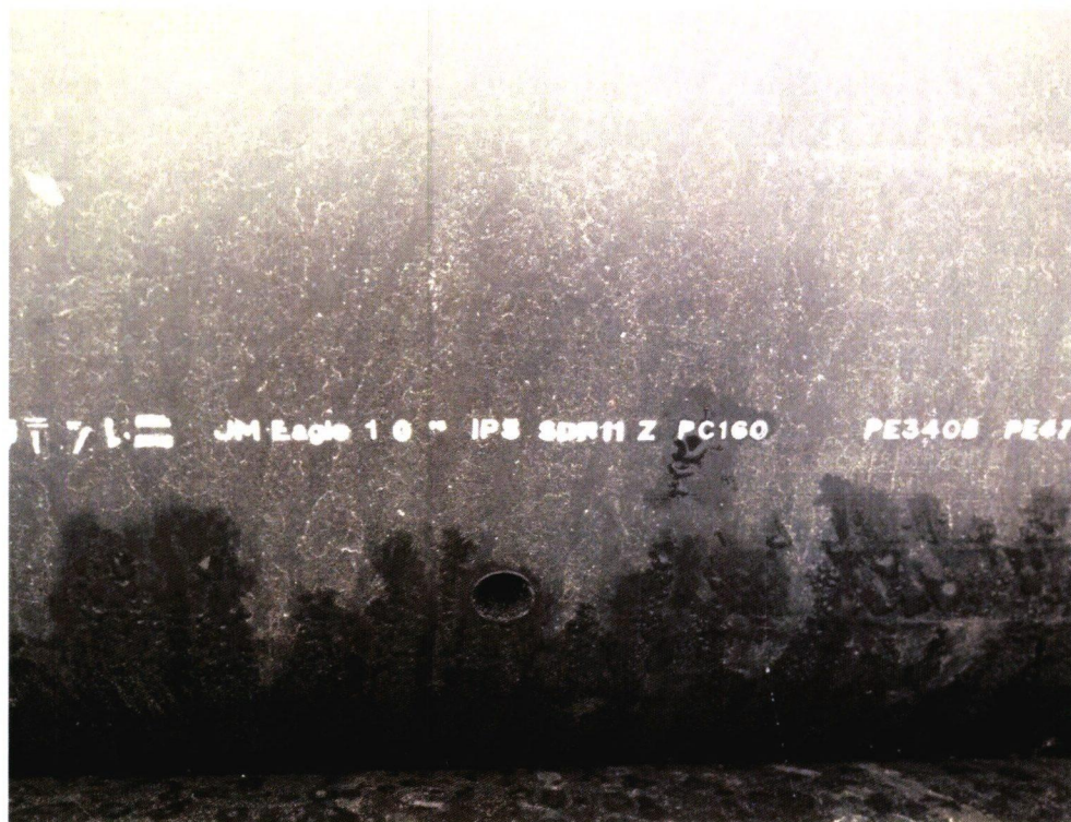
Photograph 33: 10" HDPE SDR 11 pipe for HGC's
