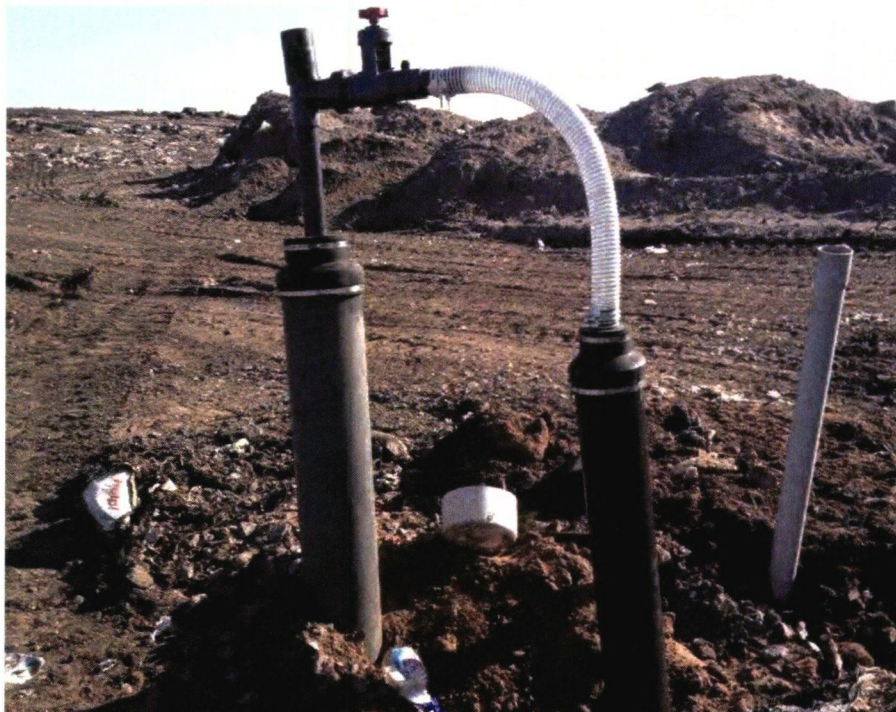
Photograph 31: Completed wellhead.
