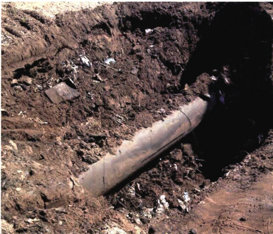
Photograph 25: Excavation of existing 18" main header in Cell 8.
