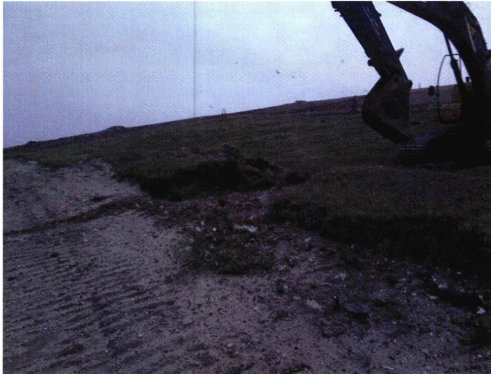
Photograph 11: Digging out lower tier berm prior to drilling.
