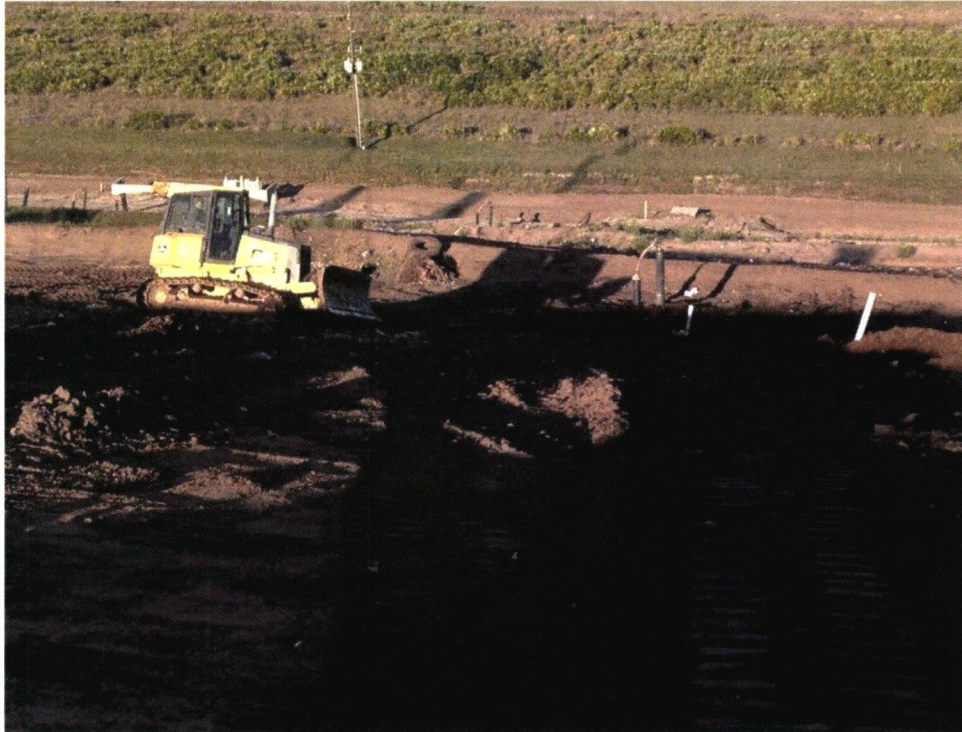
Photograph 24: Regrading slopes with dozer (typical).
