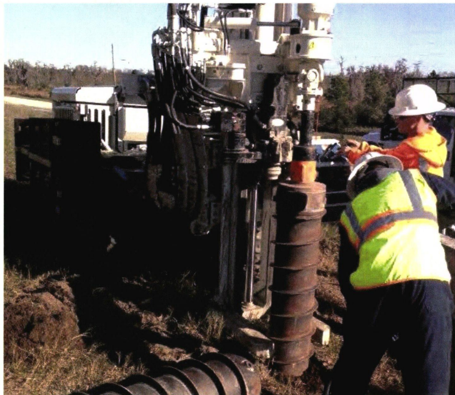
Photograph 45: Drilling borehole for soil vapor extraction well installation (typical).
