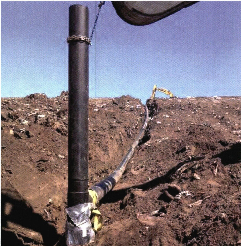
Photograph 16: Installing new lateral assembly (typical).
