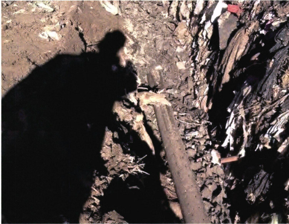
Photograph 40: Covering HGC pipe with tire chips (typical).
