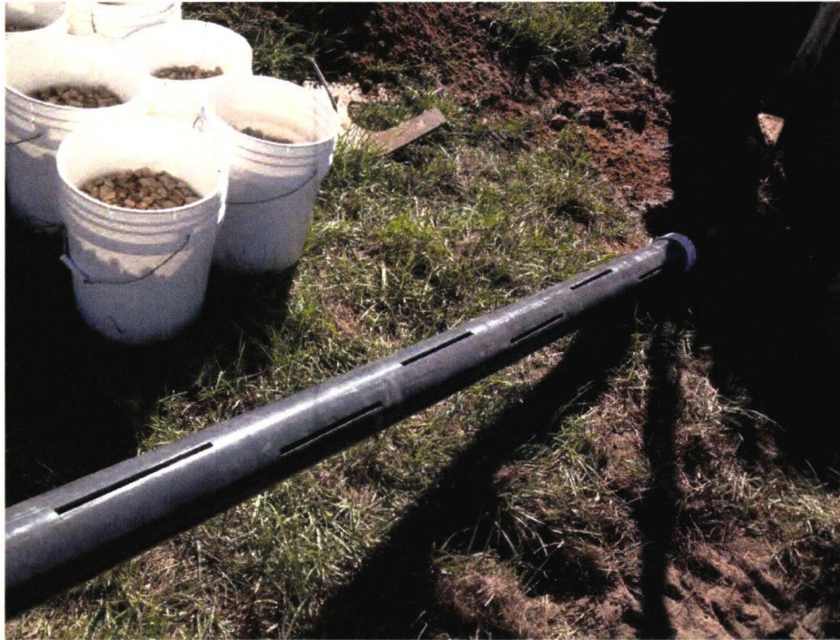
Photograph 44: Slotted SCH 80 PVC used for soil vapor extraction wells (typical).
