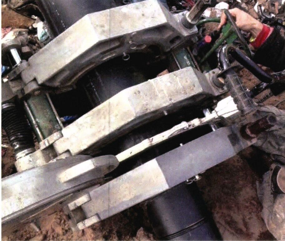
Photograph 36: 10" HDPE SDR 11 pipe weld (typical).
