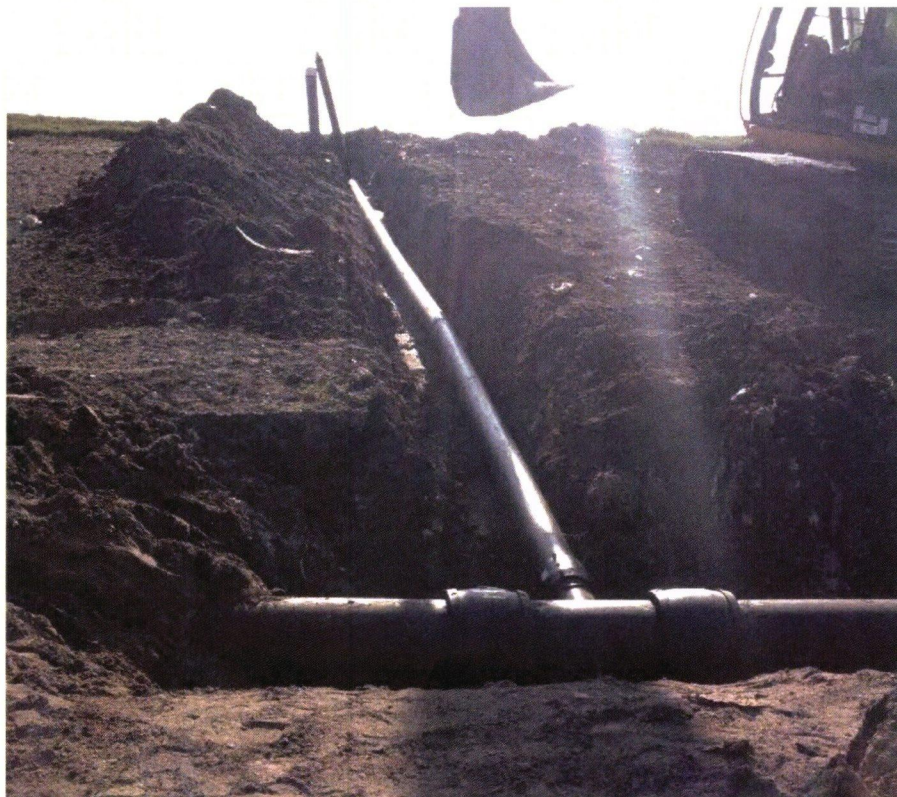
Photograph 27: Completed tie-in to 18" main header.
