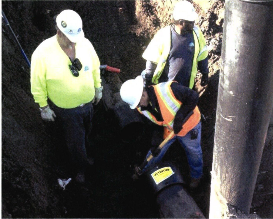
Photograph 22: 8" lateral tie-in to 14" header in Cell 8 (typical).
