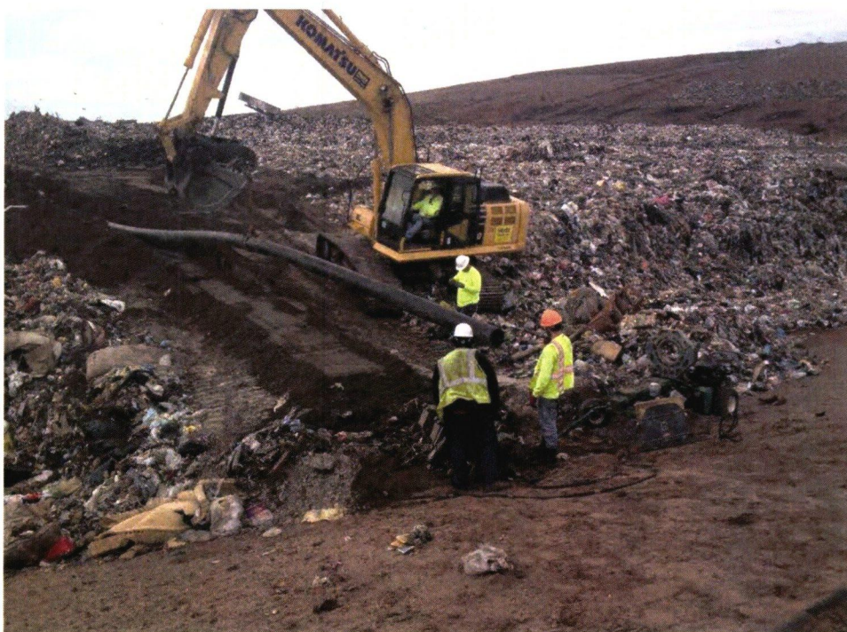
Photograph 39: Placing horizontal gas collector into excavated trench (typical).
