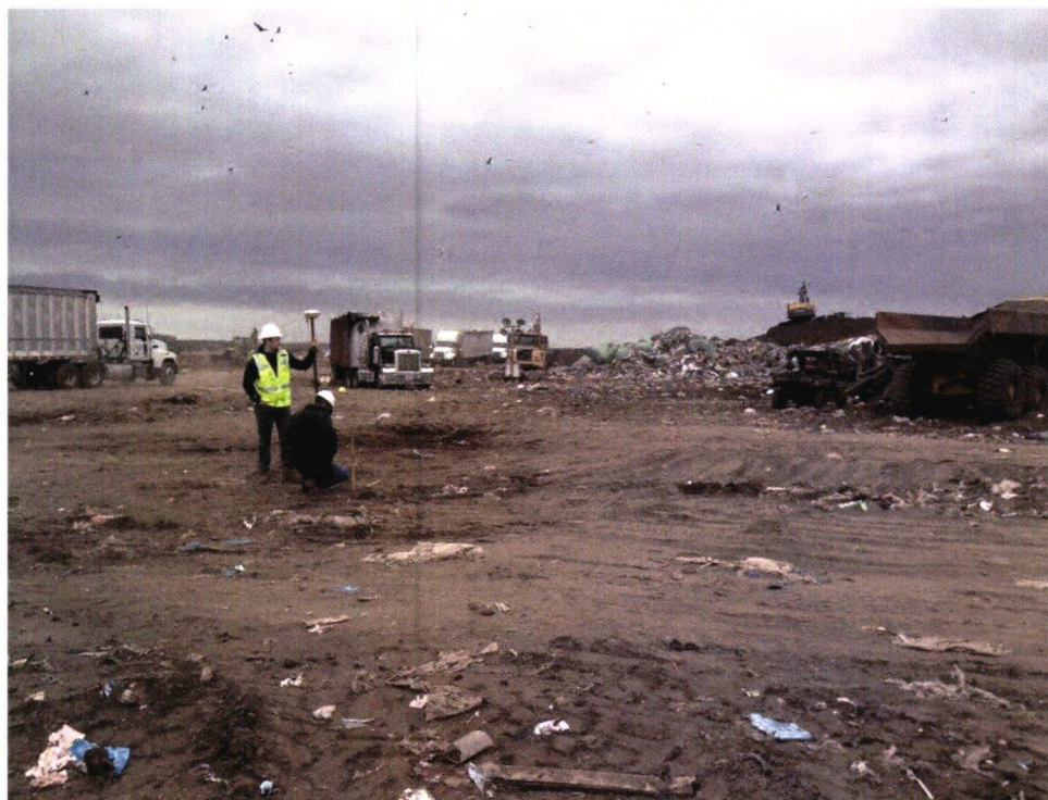
Photograph 32: Progressive staff staking horizontal gas collector (HGC) locations.
