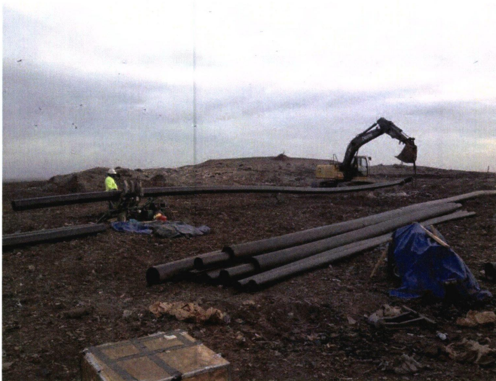
Photograph 14: Welding HDPE lateral piping (typical).
