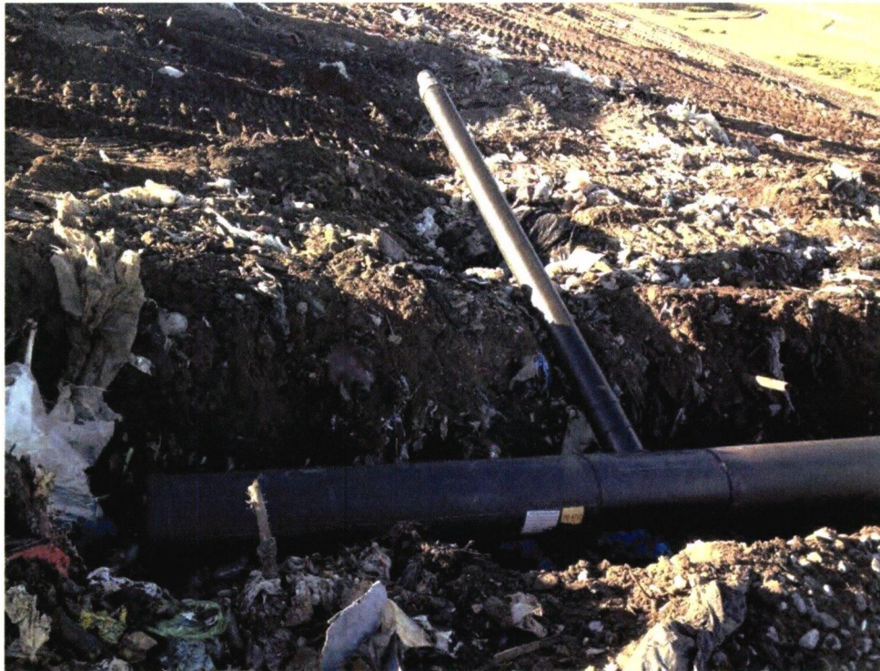
Photograph 19: New 12" subheader stubout at GW-90.
