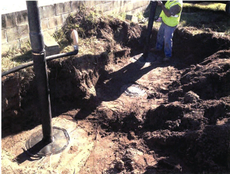
Photograph 50: Completed liner repairs (typical).
