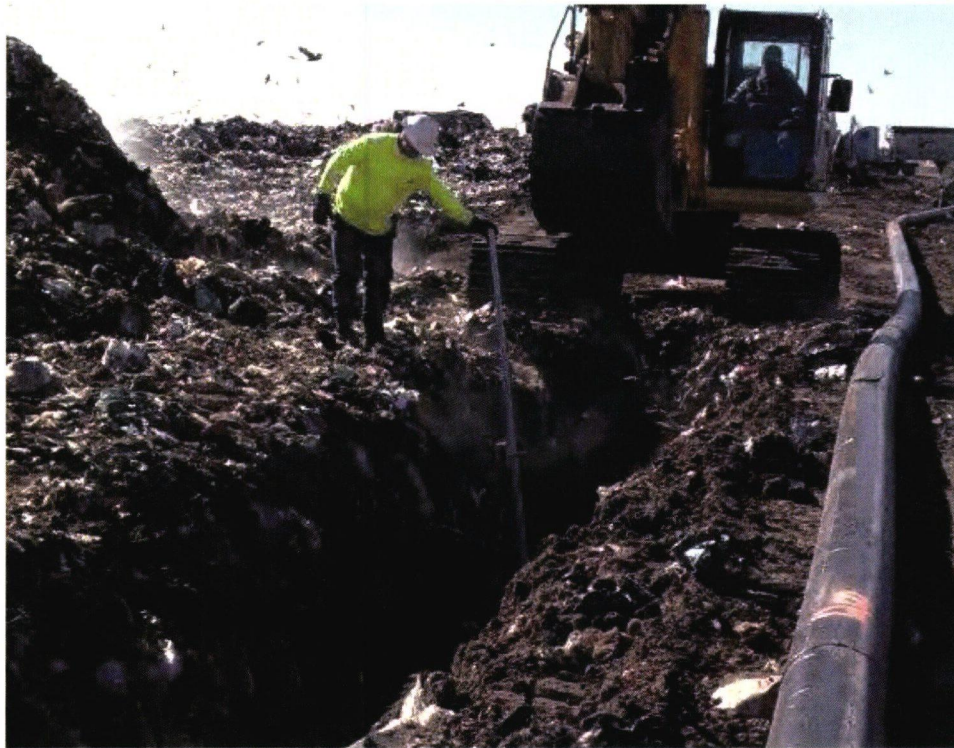
Photograph 38: Confirming slope as excavation progresses (typical).
