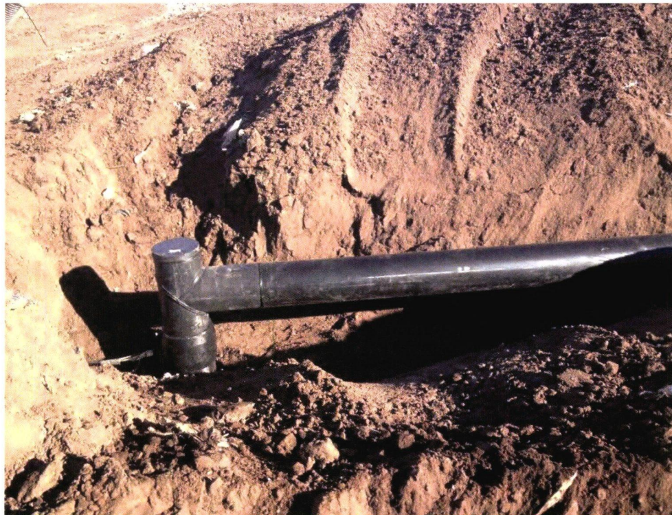
Photograph 18: Tie-in to 12" existing gas conveyance subheader.
