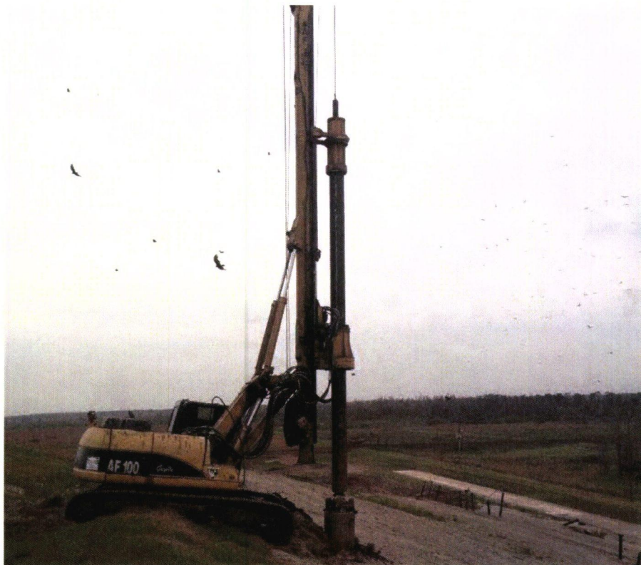
Photograph 12: Drilling lower tier wells.
