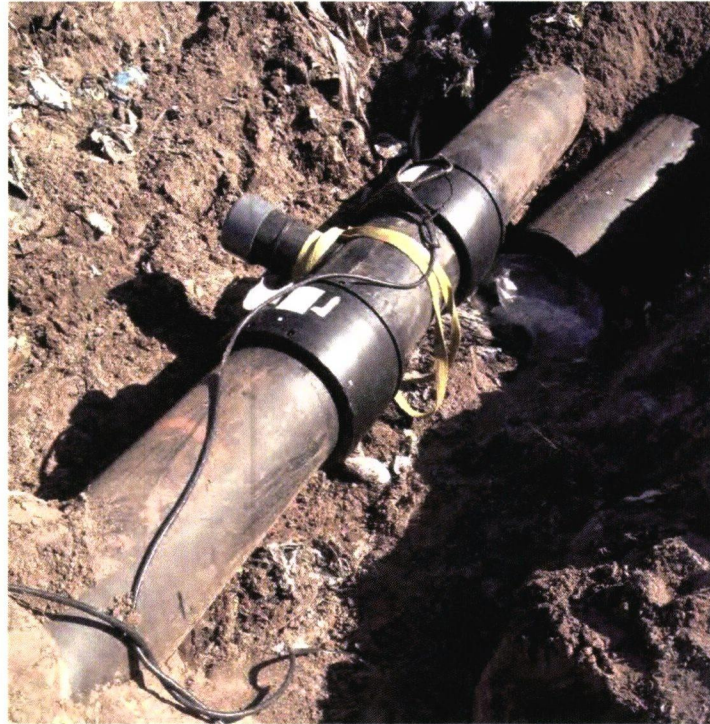
Photograph 26: Electrofusion welding of tie-in to 18" main header.
