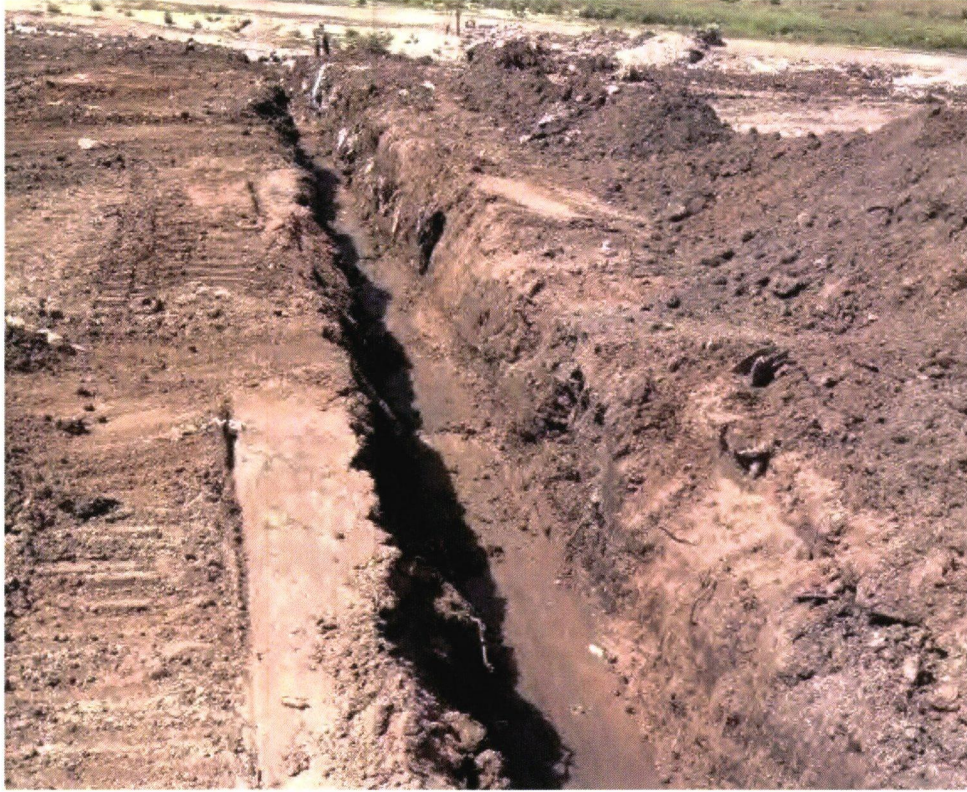
Photograph 13: Standard trench for lateral (typical).
