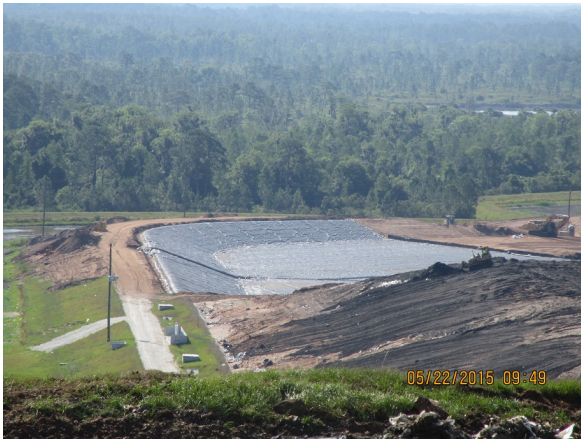
Liner installation Cell 11
