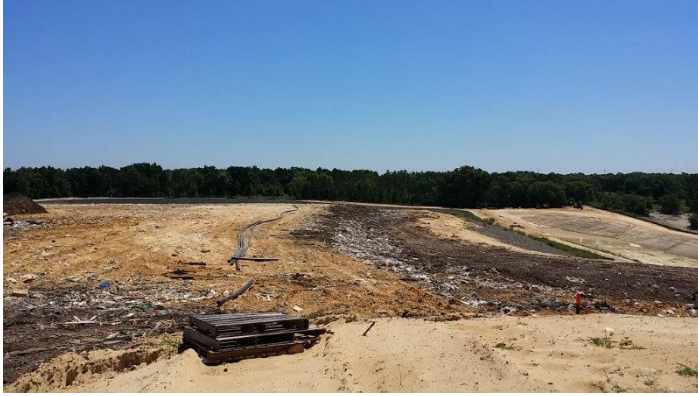
Cell 3 where pipe HC-10 was laid
