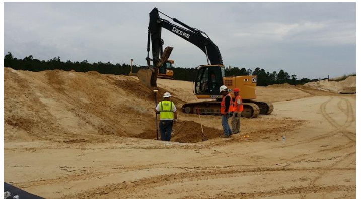
Construction of leachate sump
