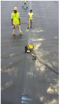
Join 2 HDPE panels by welding
