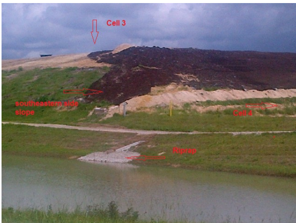
Repaired side slope & riprap
