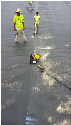
Join 2 HDPE panels by welding
