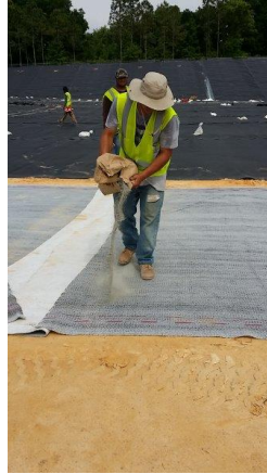
Join 2 GCL panels by overlapping
