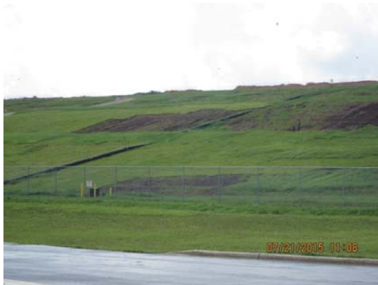
Stage III Erosion Repair
