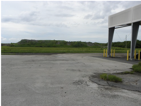
RSM Stockpile for LF Uses
