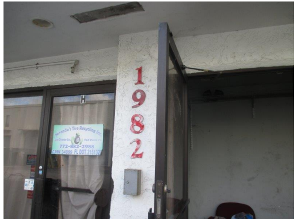
frontage of building
