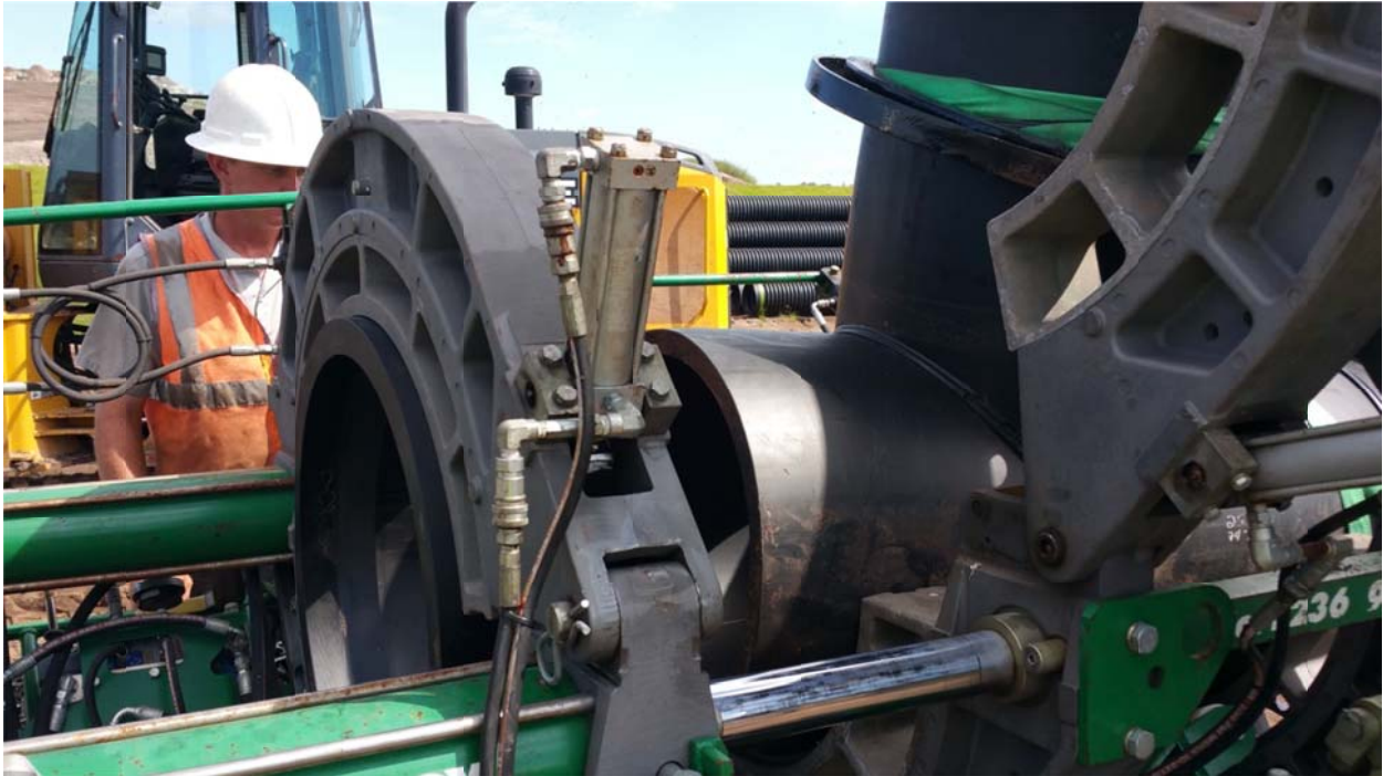
Butt Fusion Welding of 36" HDPE Pipe
