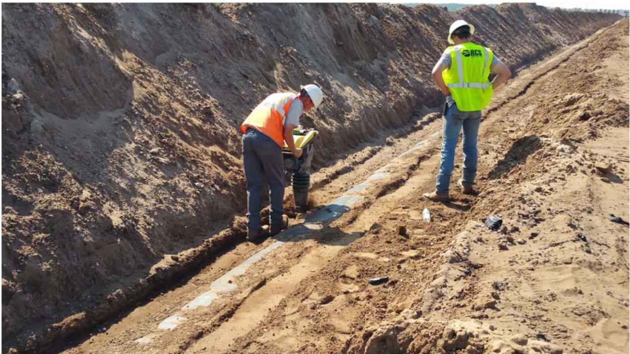
Compaction Around 36" HDPE Pipe with Jumping Jack Compactor
