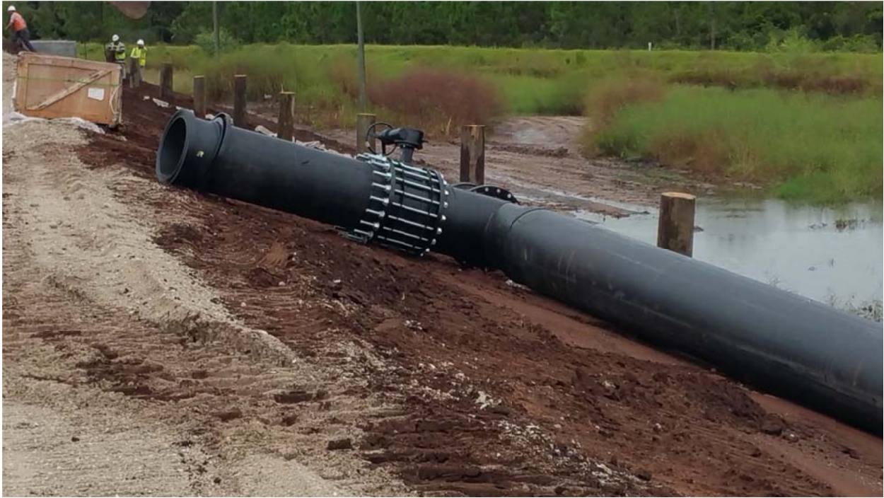
Wooden Pipe Support for 28" HDPE Pipe On Backside of Perimeter Berm
