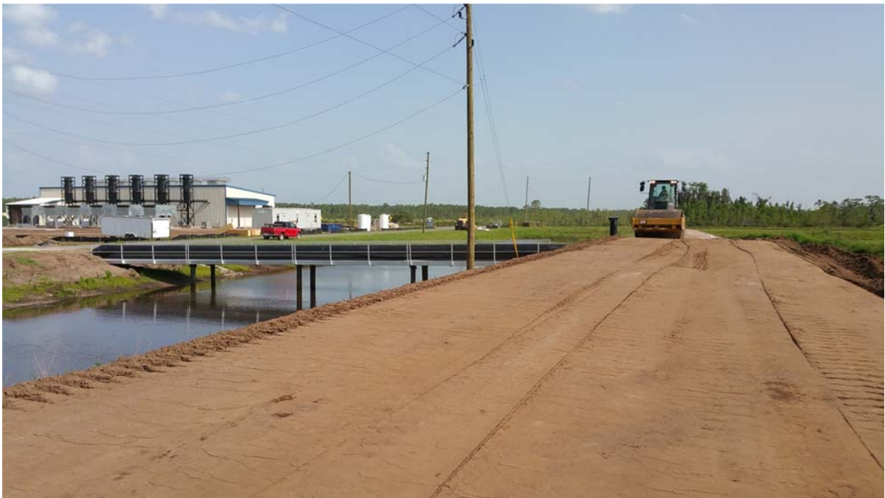
Aluminum Bridge at Completion and Compaction of Finished Grade
