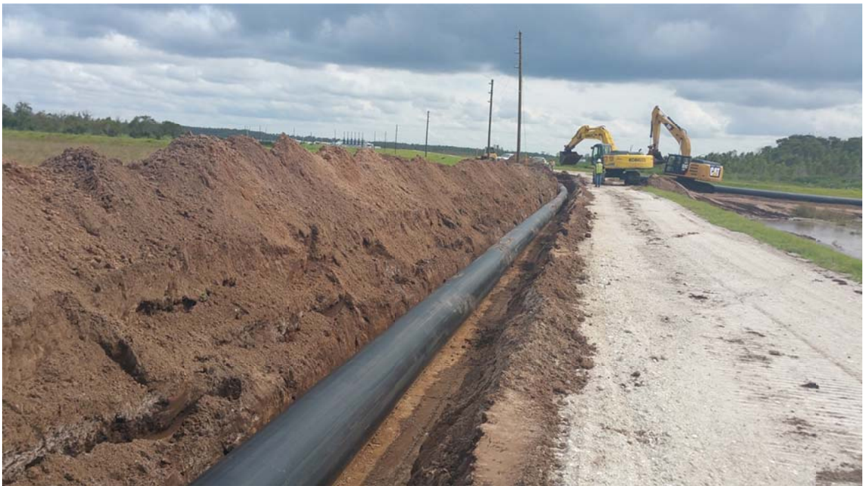
Placement of 36" HDPE Pipe in Trench
