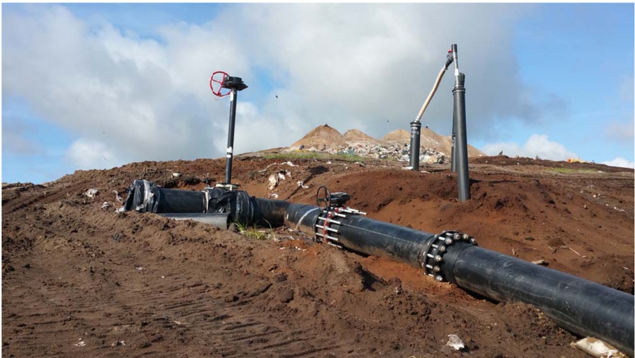
18" HDPE Tie In To Existing Header
