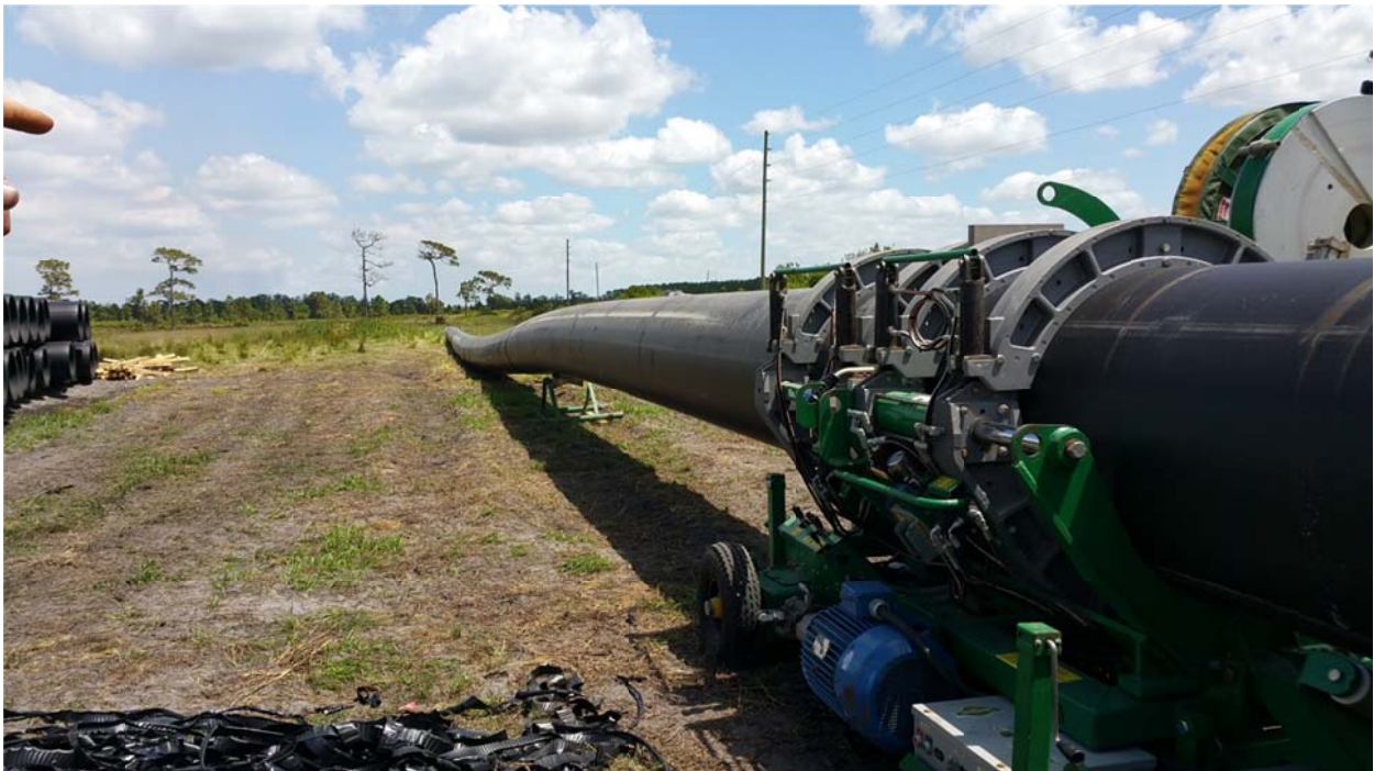
Butt Fusion Welding of 36" HDPE Pipe
