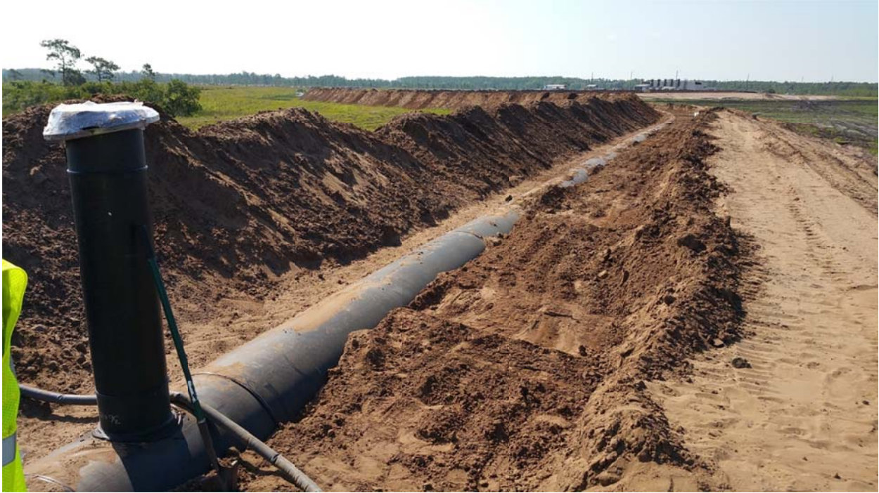
Backfill Around 36" HDPE Pipe
