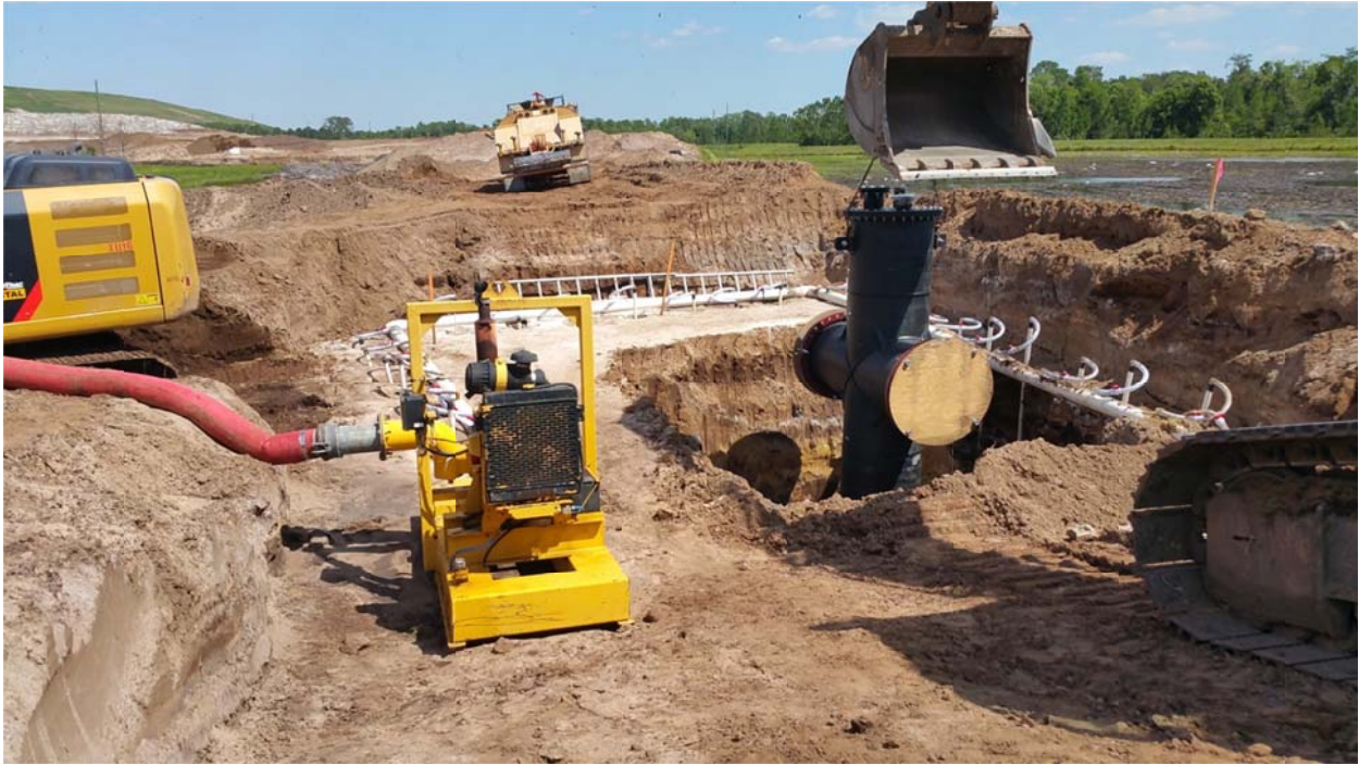
Placement of 36" Condensate Sump
