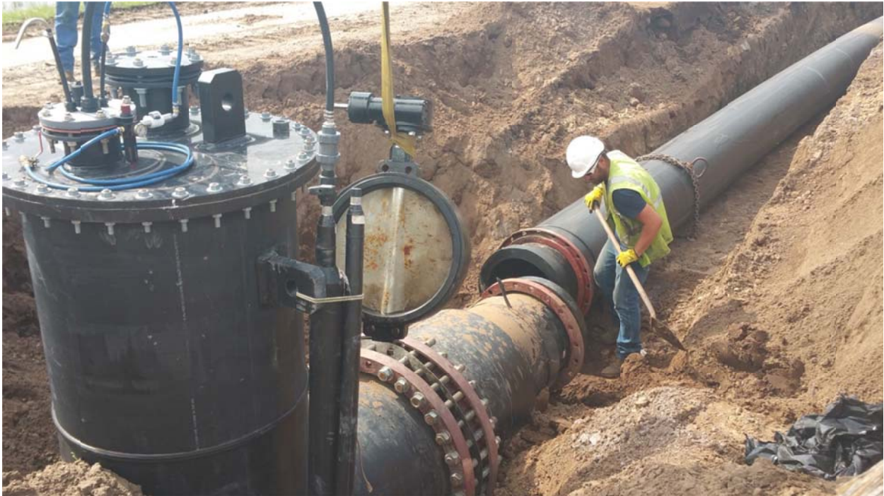
Connection of 36" HDPE Pipe to Condensate Sump
