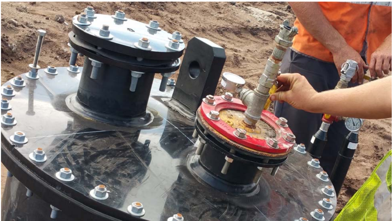
Pneumatic Pressure Test of 36" Pipe Network (Note Pneumatic Pressure test of Air Line to Far Right)
