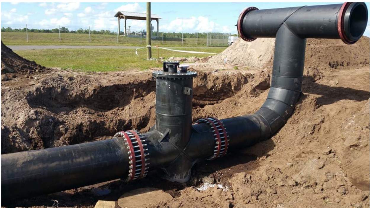
"T" Tie-in to LFGTE Blower Station
