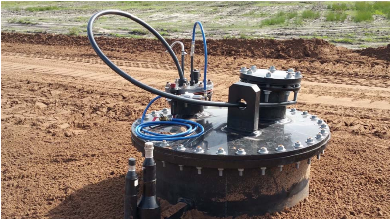
Completed Condensate Sump with Air and Forcemain
