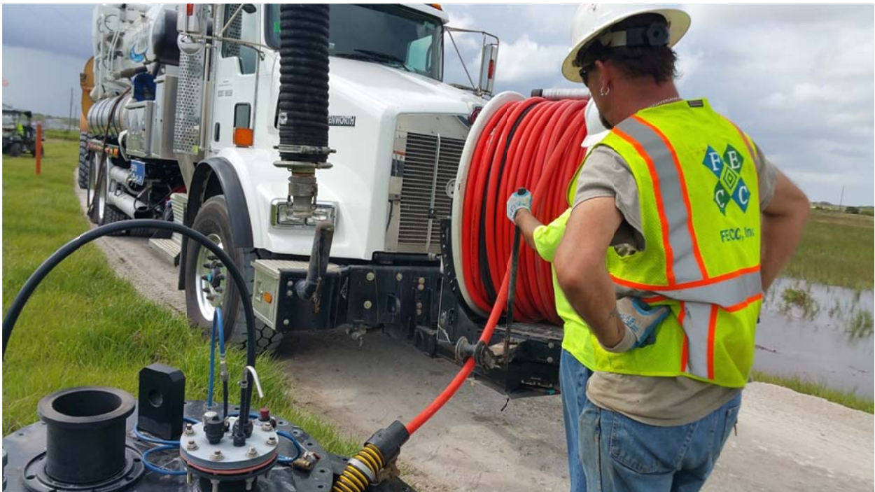
Water Pressure Jet Cleaning of HDPE Pipe Network
