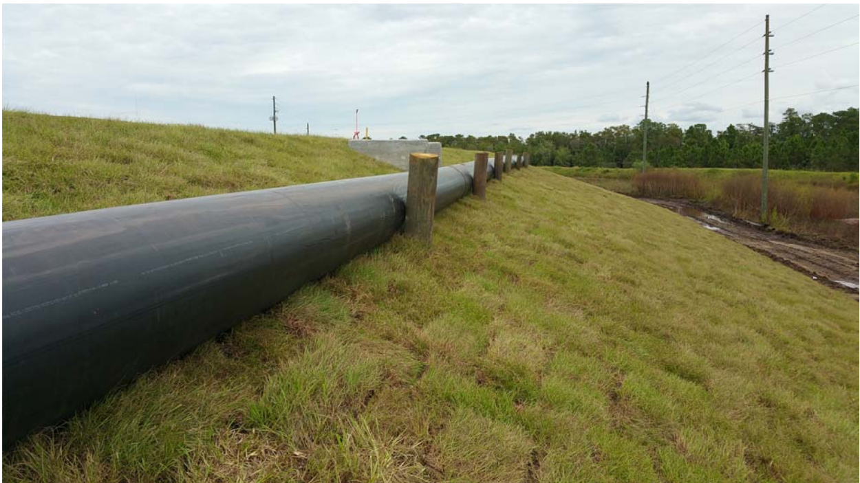
28" HDPE Pipe Support on Slope
