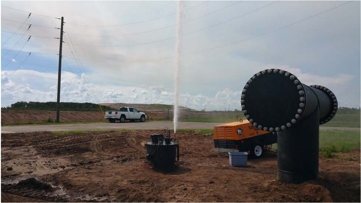
Release of Hydrostatic Pressure in 4"HDPE Forcemain
