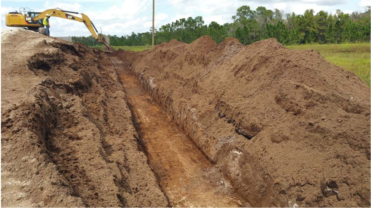
Excavation of Trench for 36" Pipe Placement
