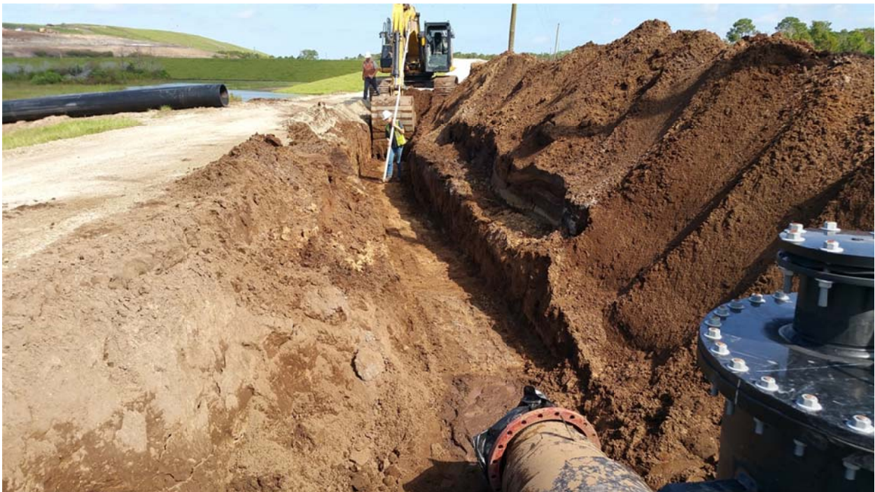
Survey of Slope for Pipe Placement
