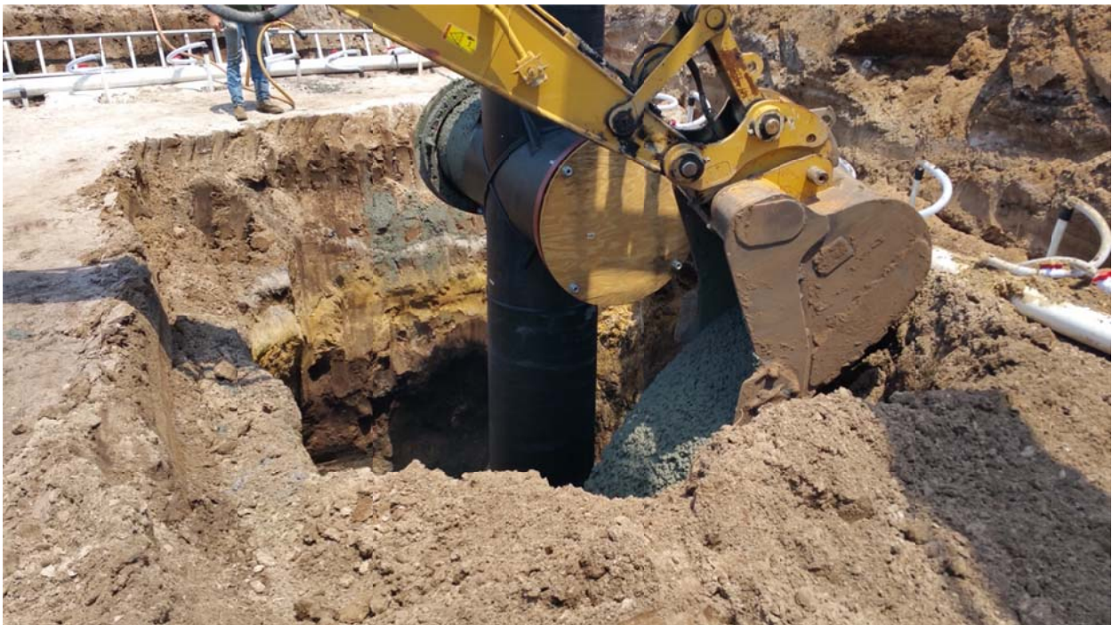
Placement of Concrete for Anti-Flotation
