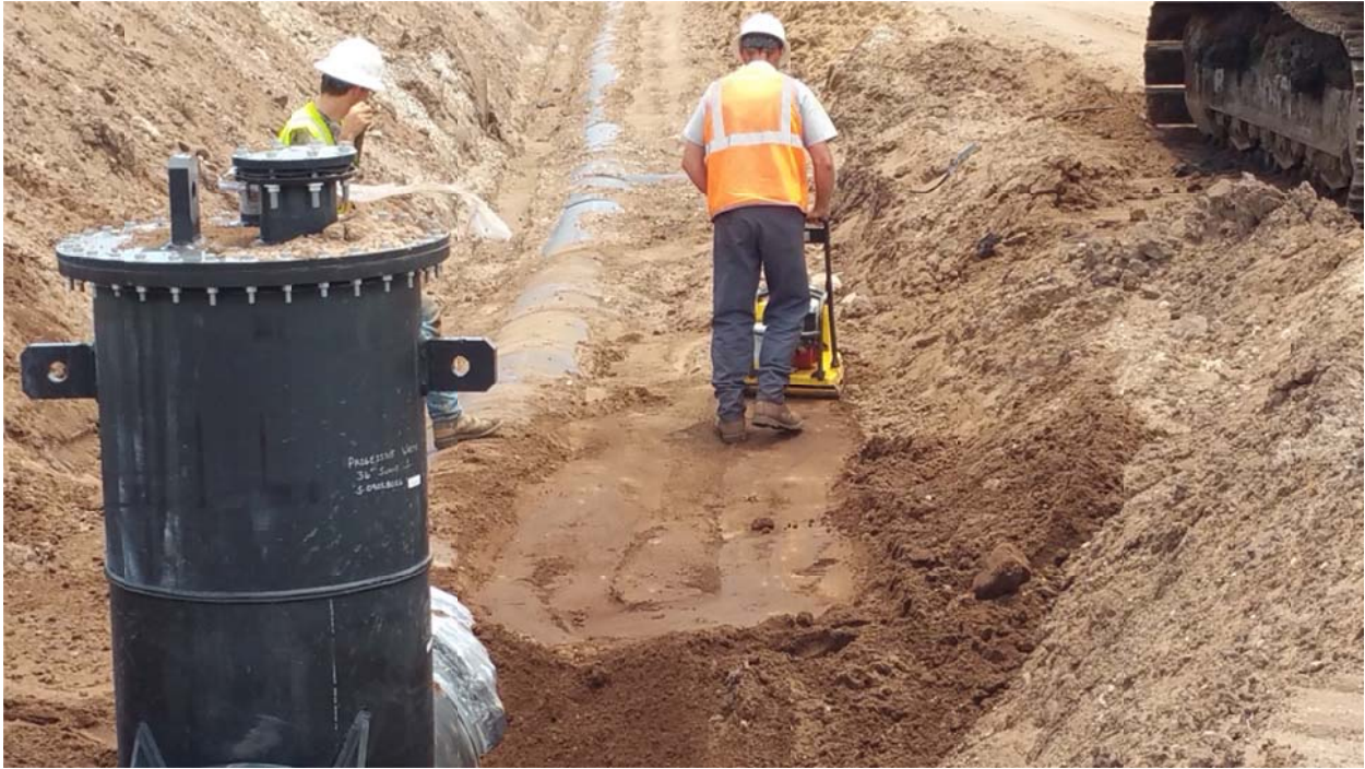
Compaction Around 36" HDPE Pipe with Vibratory Whacker Packer
