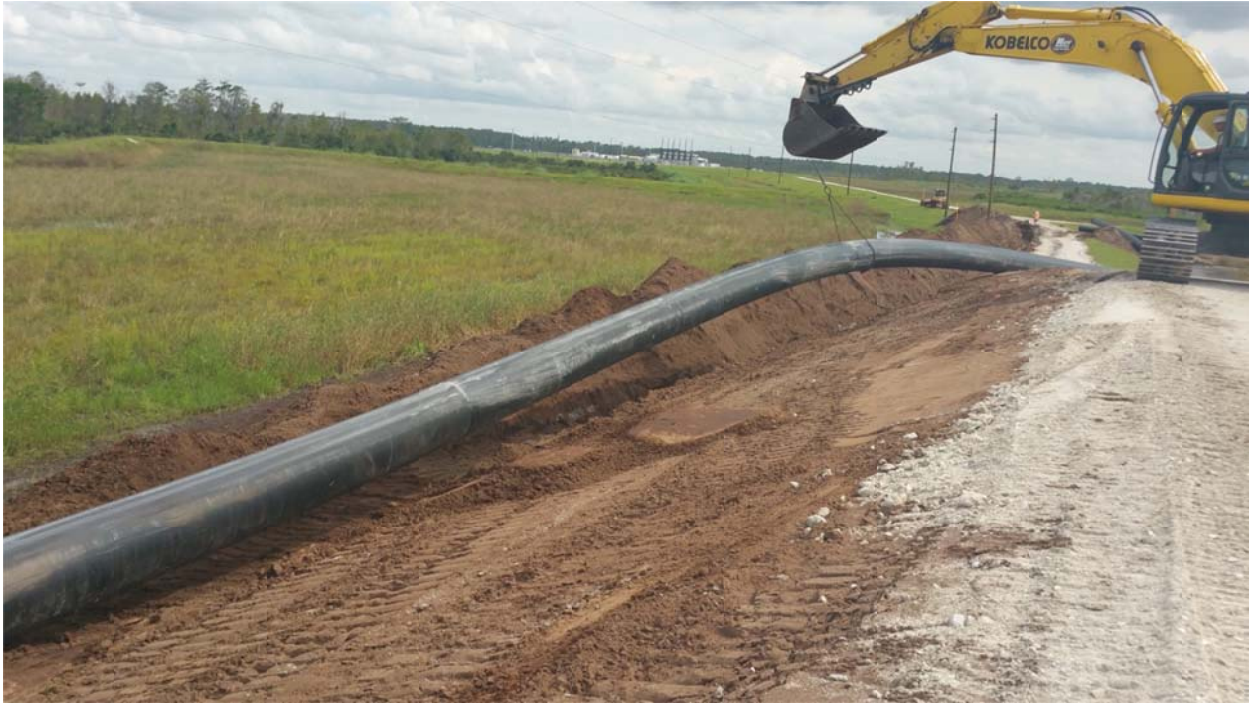
Placement of 36" HDPE Pipe in Trench
