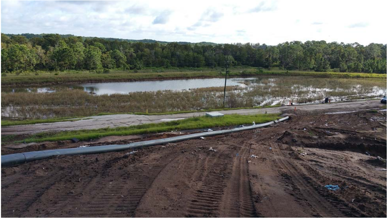
18" HDPE Up the Slope to Tie In to Existing Header
