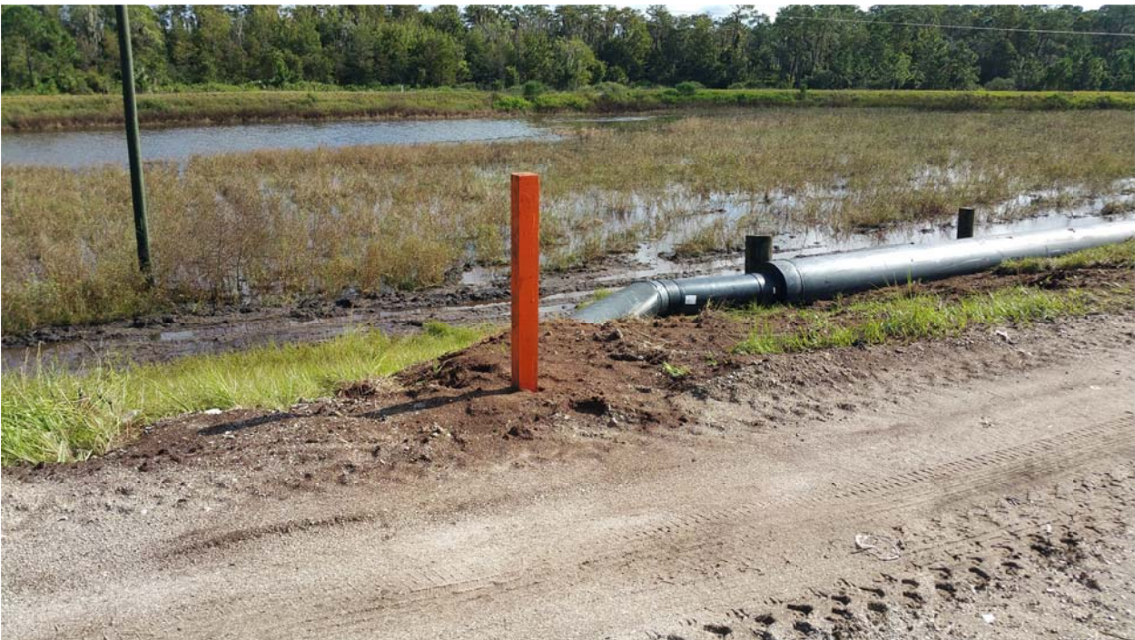
Perimeter Road Crossing of 18" HDPE
