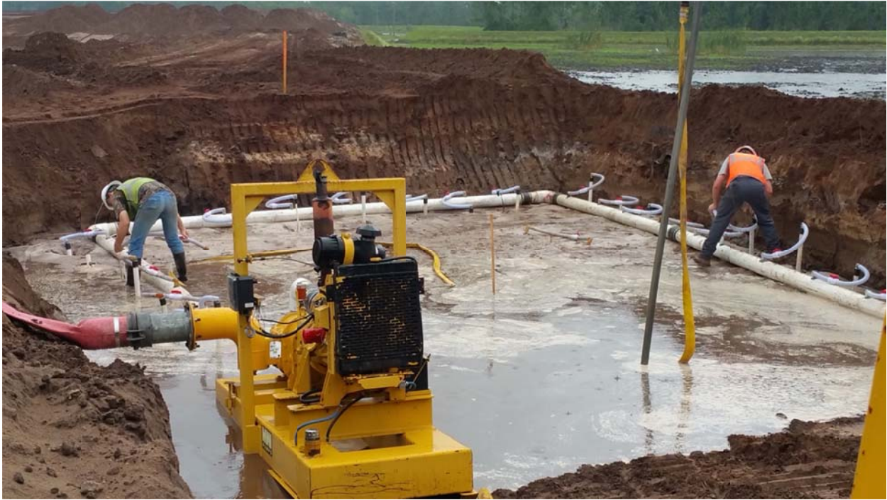
Well Point to Dewater in Condensate Sump Locations
