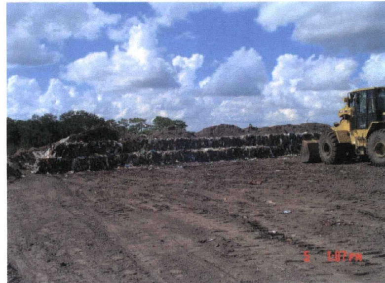
12. General view of baled CLI working face
