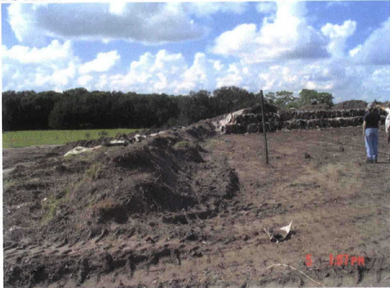
13. Berm adjacent to working face
