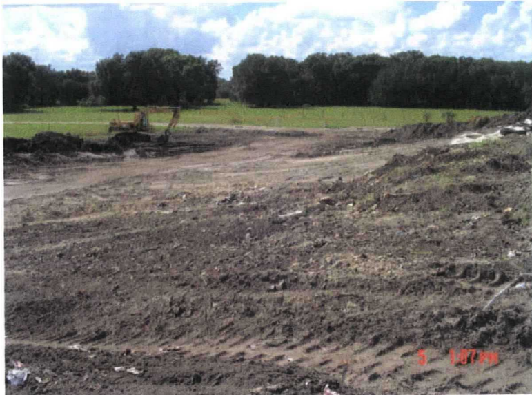
14. View looking below berm
