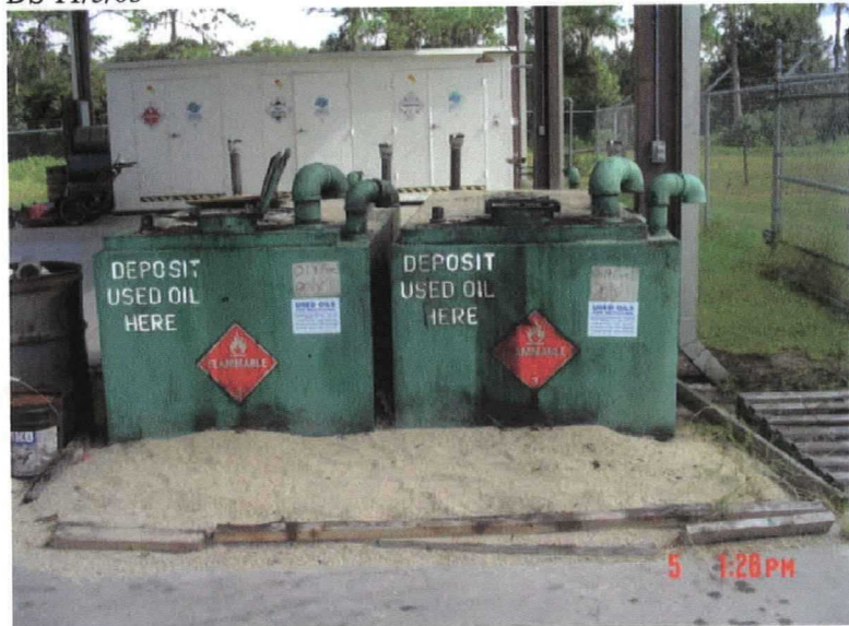
29. General view of used oil storage area
