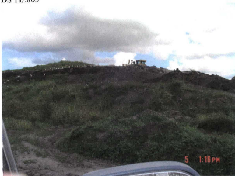
21. View from north side of working face looking up
