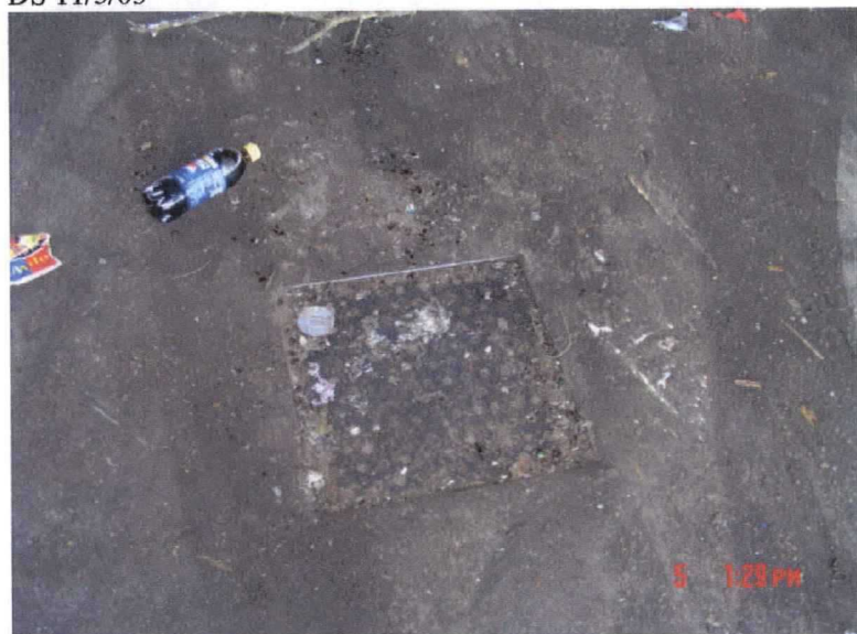
31. Leachate drain inside of MRF
