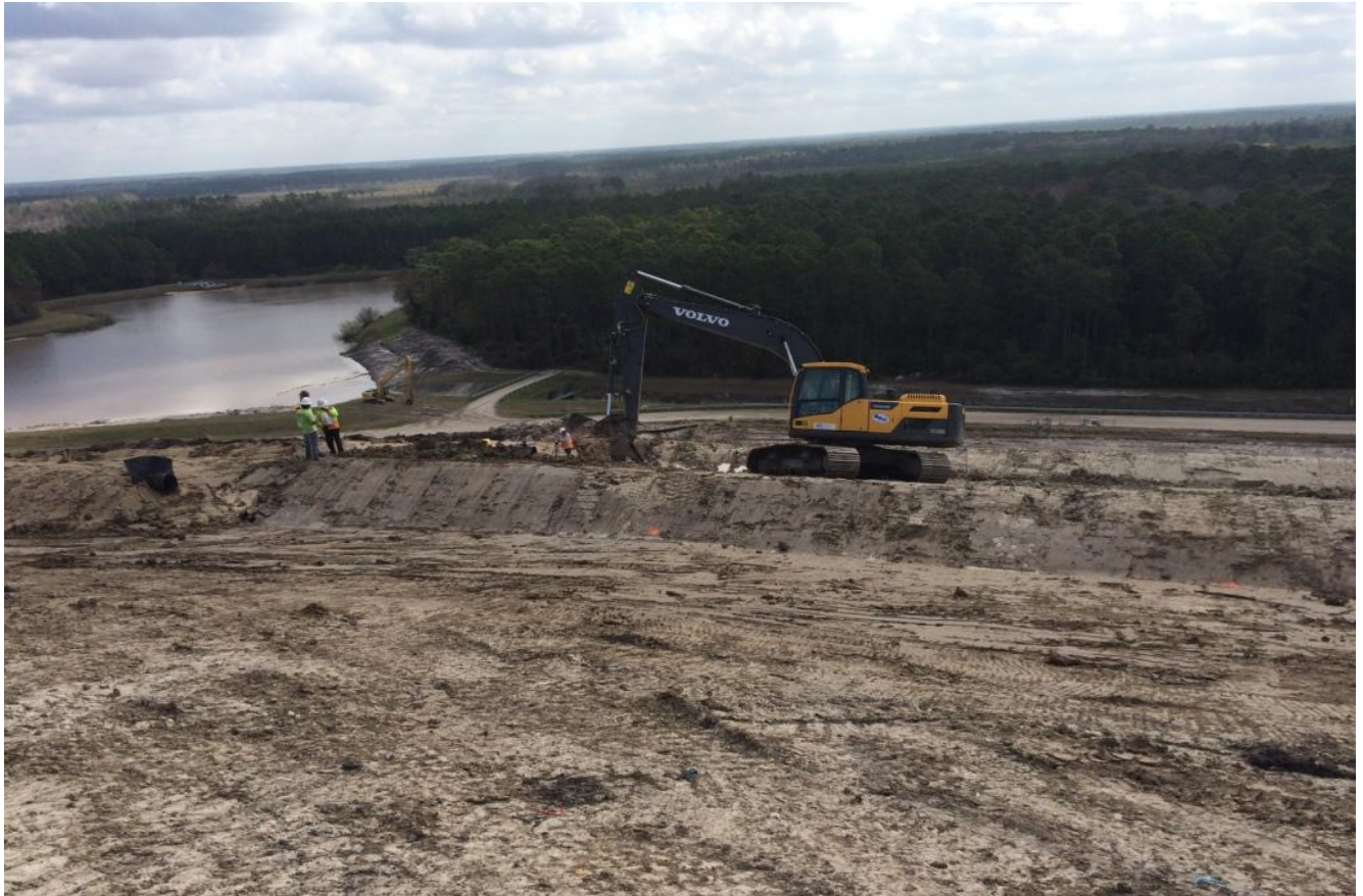
Grading Clay for Terrace Underdrain within Units 51 thru 53 (Facing Easterly) (March 2015)
