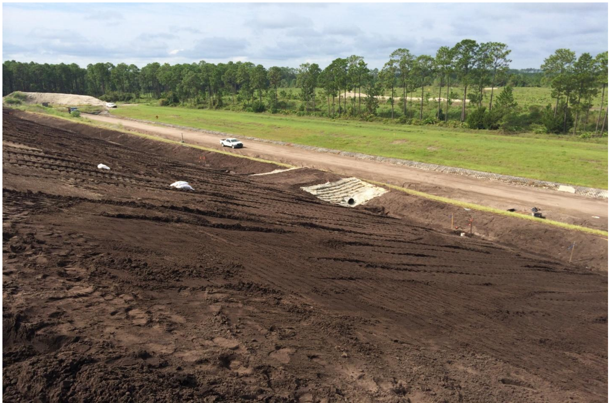
Completed Rip Rap – Downcomer D-52 at Terrace 2 (Facing Southwesterly) (August 2014)
