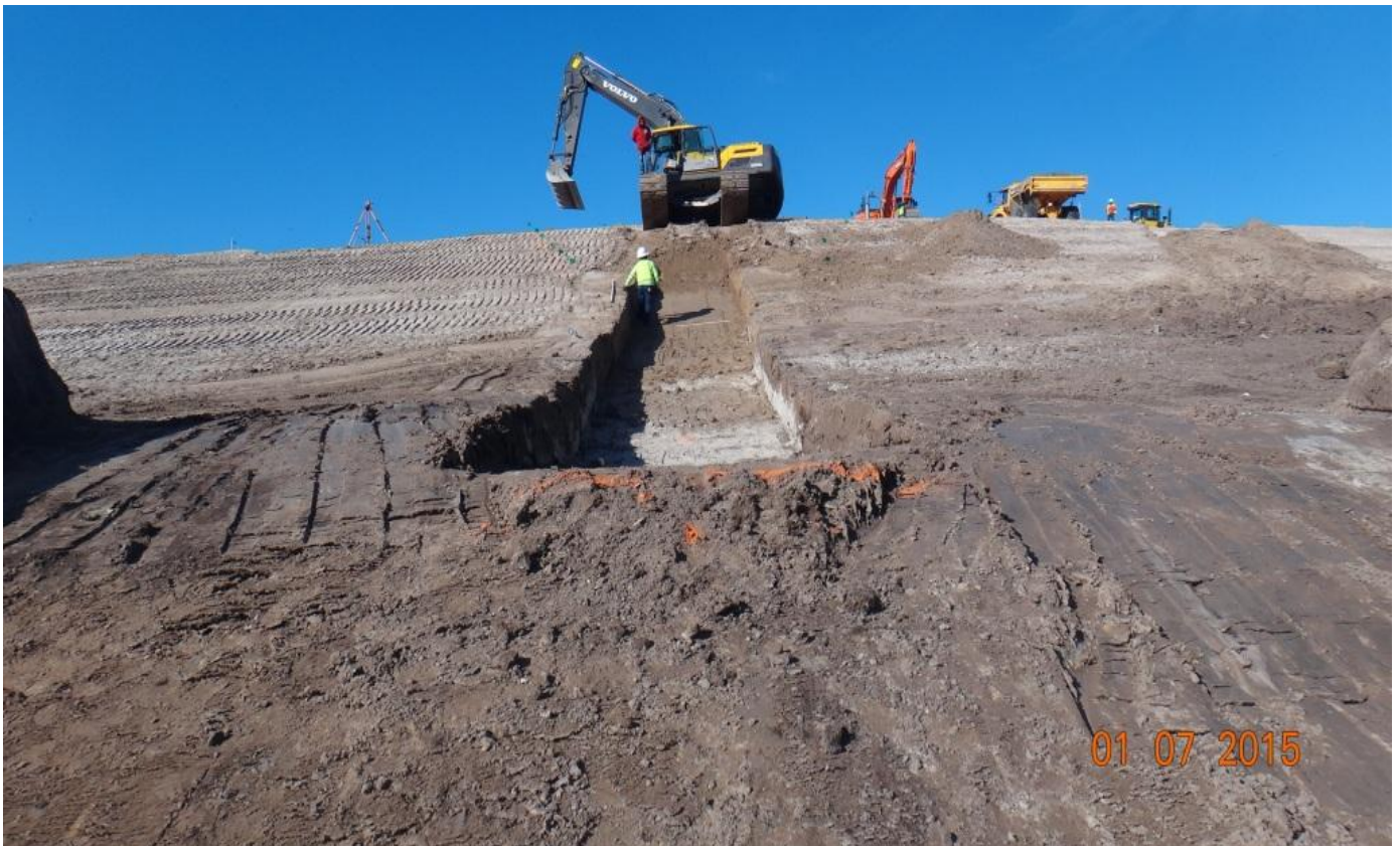
Excavating Initial Cover for Downcomer D-38 (Facing North) (January 2015)
