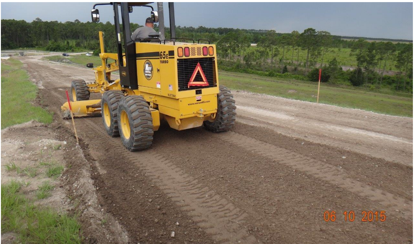
Grading Maintenance Road prior to prime coat installation (facing southwesterly) (June 2015)
