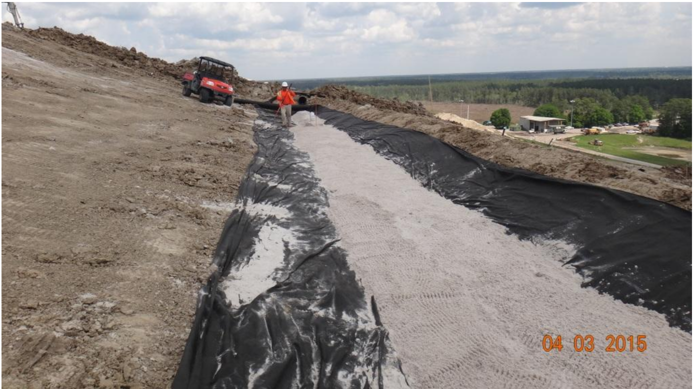
Installing Underdrain within Unit 52 (Facing Northerly) (April 2015)
