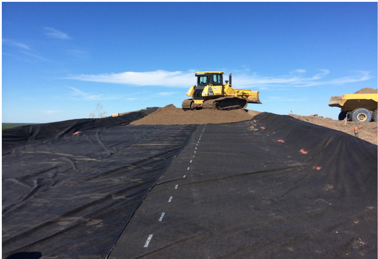
Placing crushcrete over geotextile for Maintenance Road (Facing North) (October 2014)
