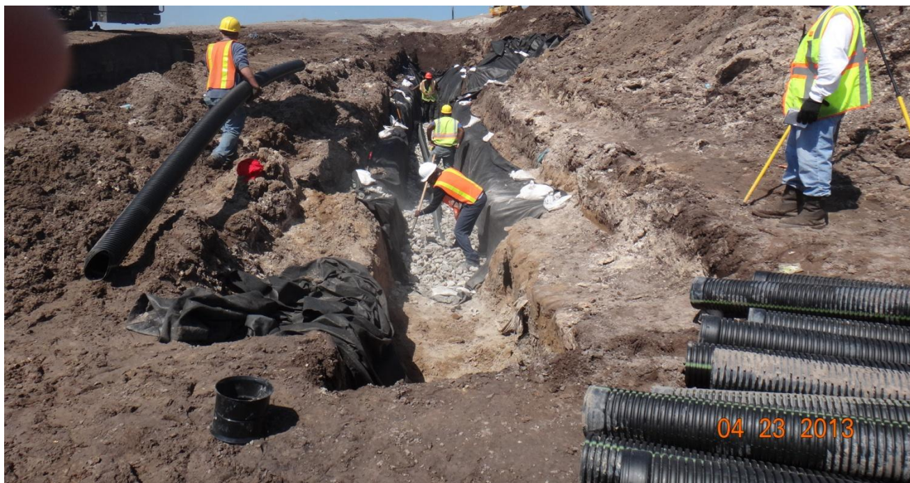
Installing Seep Drain – Units 71 and 72 (Facing easterly) (April 2013)
