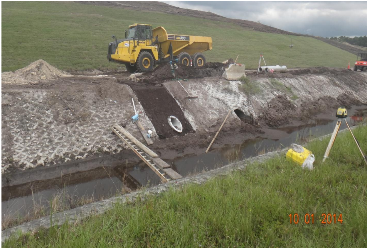
Finished subgrade at fabra-form replacement S-110 (Facing Southeasterly) (October 2014)
