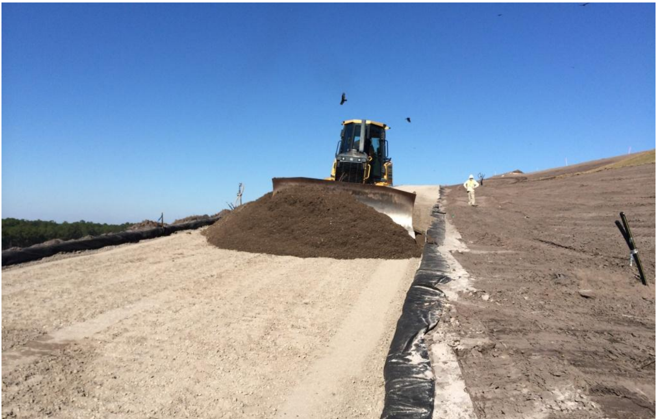
Placing Second Lift of Crushcrete for Maintenance Road (Facing North) (November 2014)
