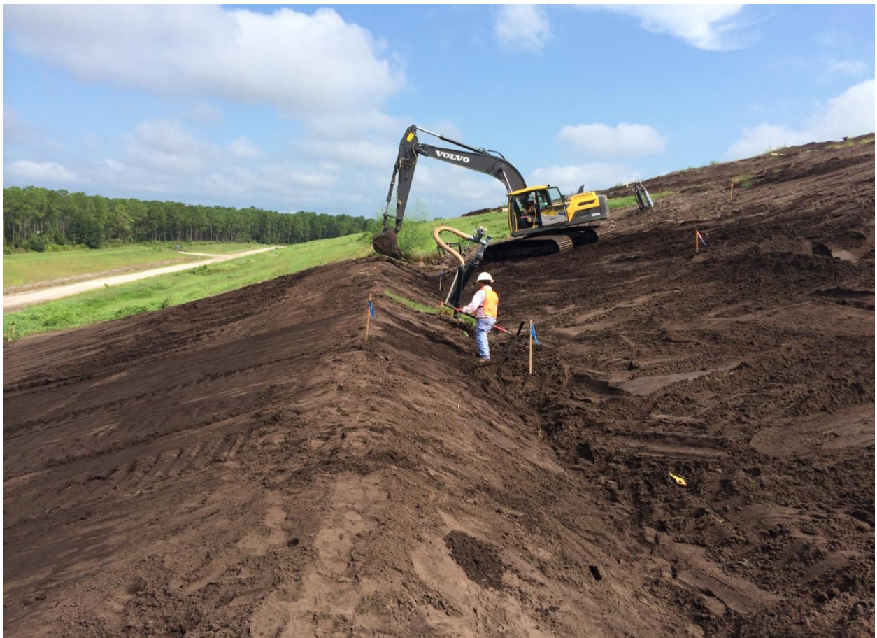
Grading terrace swales – Unit 77 at Terrace 3 (Facing Northerly) (September 2014)
