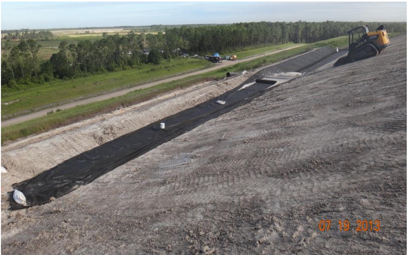
Underdrain wrapped with filter fabric (facing north) (July 2013)
