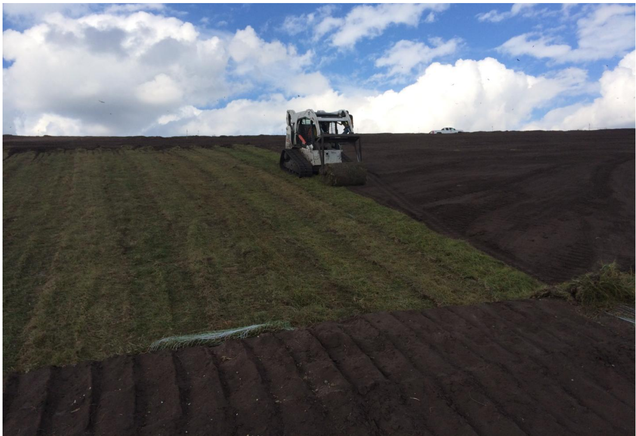
Installing rolled sod with overlapping joints Unit 66 (Facing North) (October 2014)
