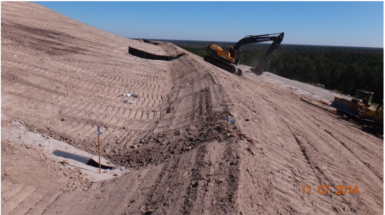
Grading Initial Cover (Units 57 – 59) (Facing East) (November 2014)
