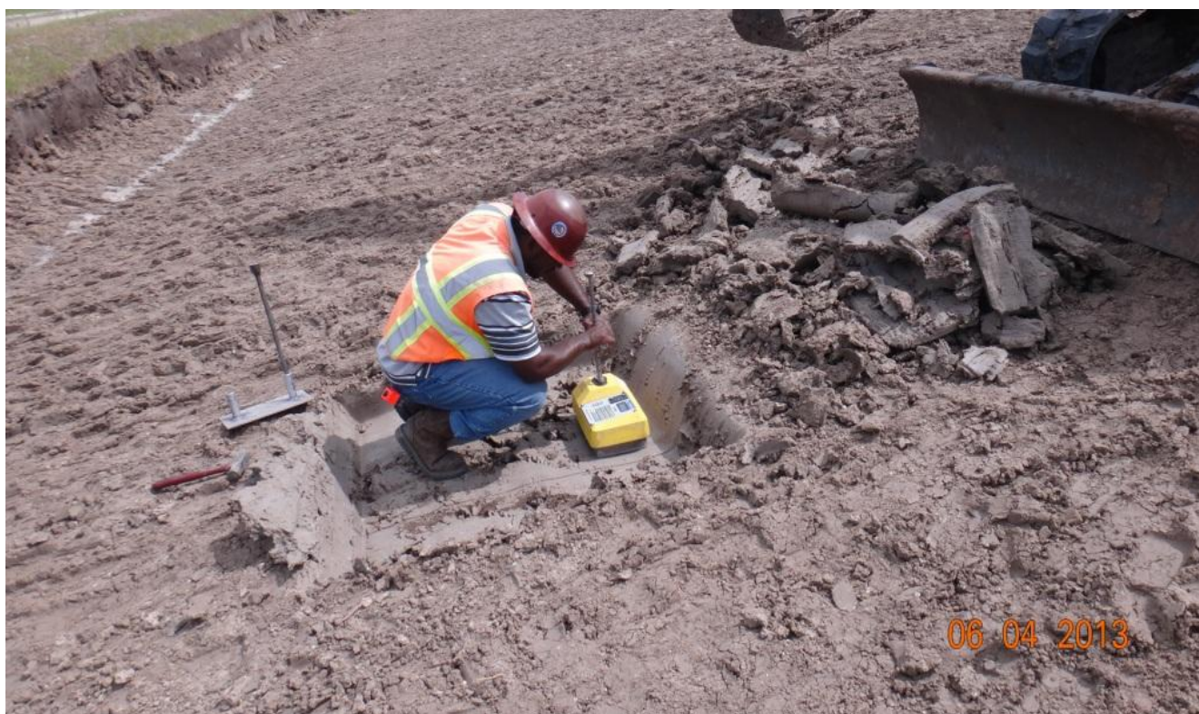
Density Testing Clay – Units 79 (Facing North) (June 2013)
