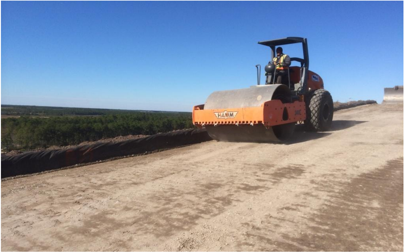
Compacting First Lift Crushcrete for Maintenance Road (Facing Northwesterly) (November 2014)
