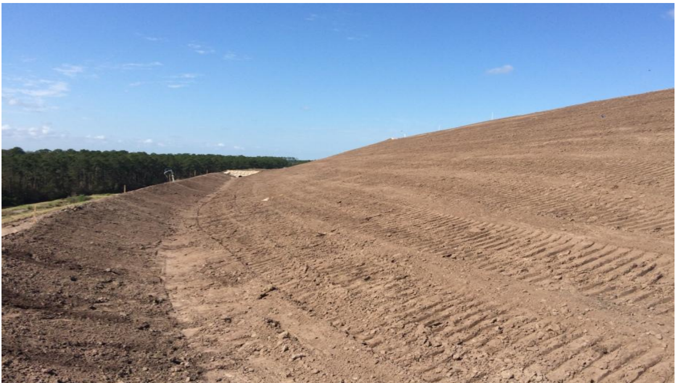
Graded Top Soil within Units 57 thru 59 (Facing Southwesterly) (March 2015)
