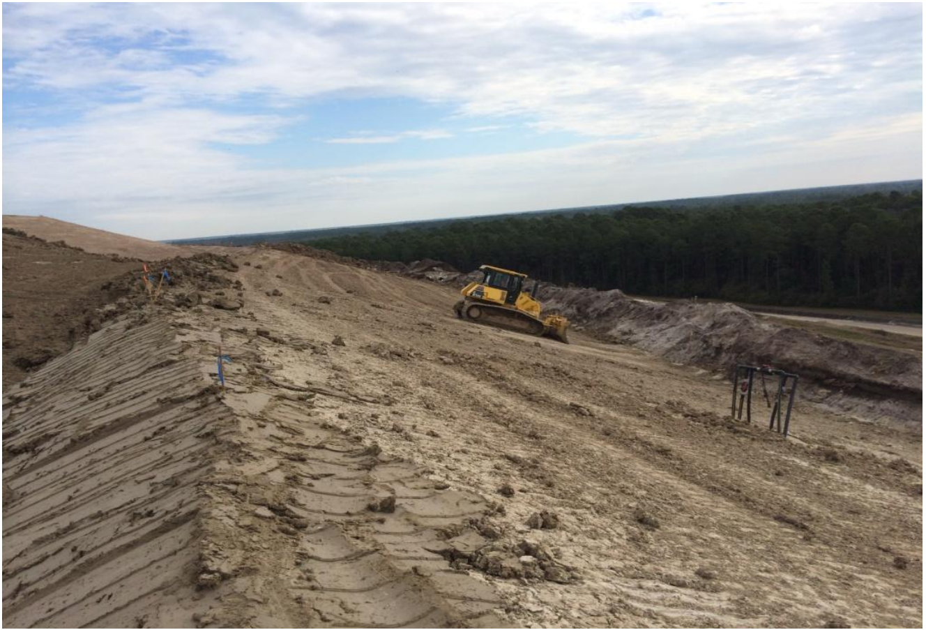
Grading Clay (Unit 60) (Facing East) (December 2014)
