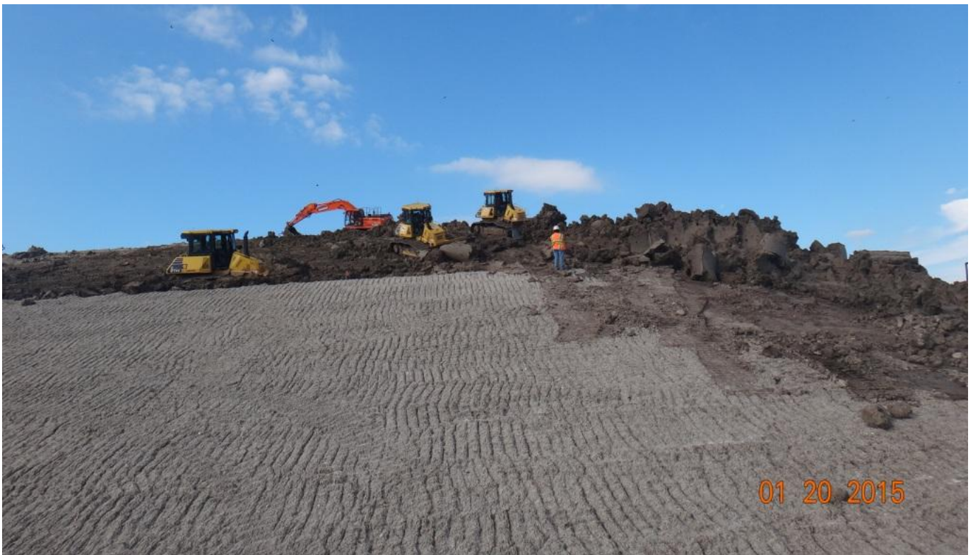
Placing Clay (Unit 55) (Facing Northwesterly) (January 2015)
