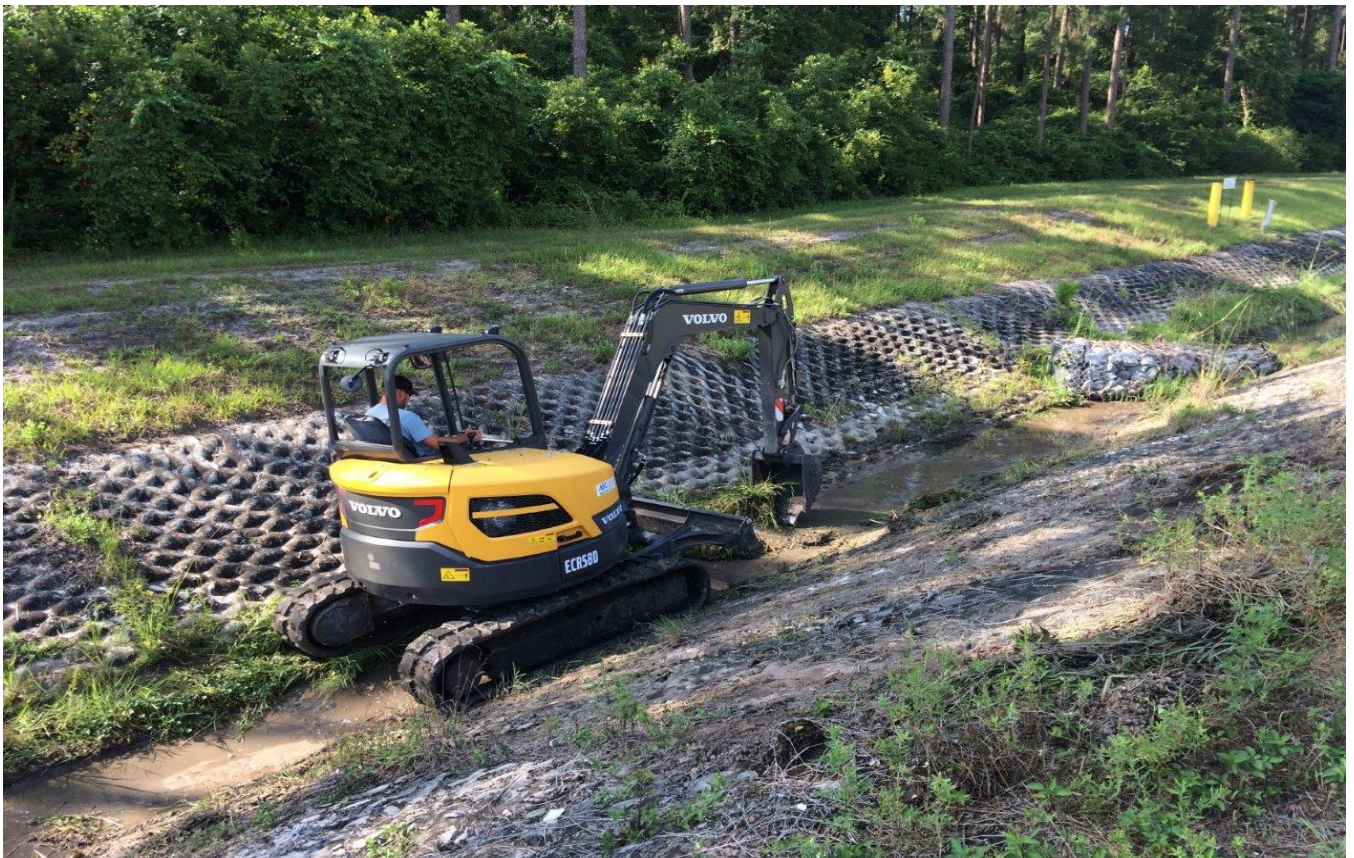
Cleaning Fabra form Ditch – Southside of Landfill (facing westerly) (June 2015)
