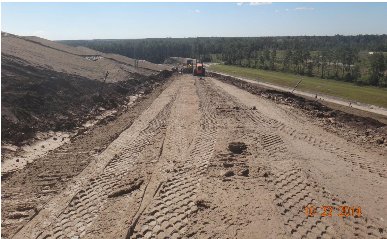
Compacting Clay along Maintenance Road (Facing South) (October 2014)
