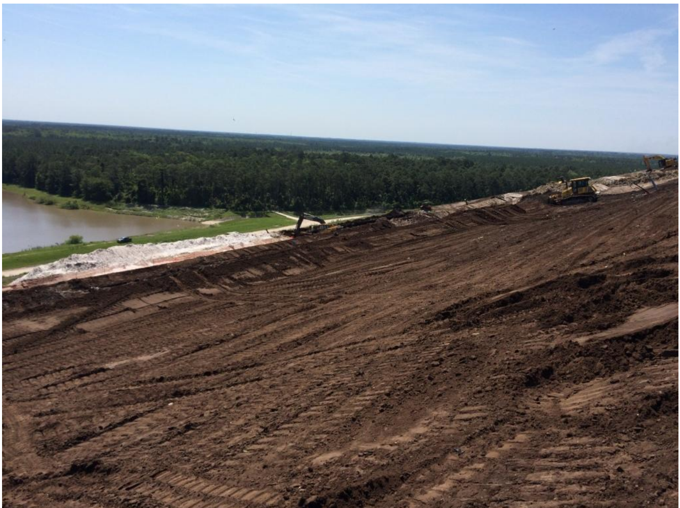
Graded Terrace Swale within Units 51-53 (Facing Southeasterly) (April 2015)
