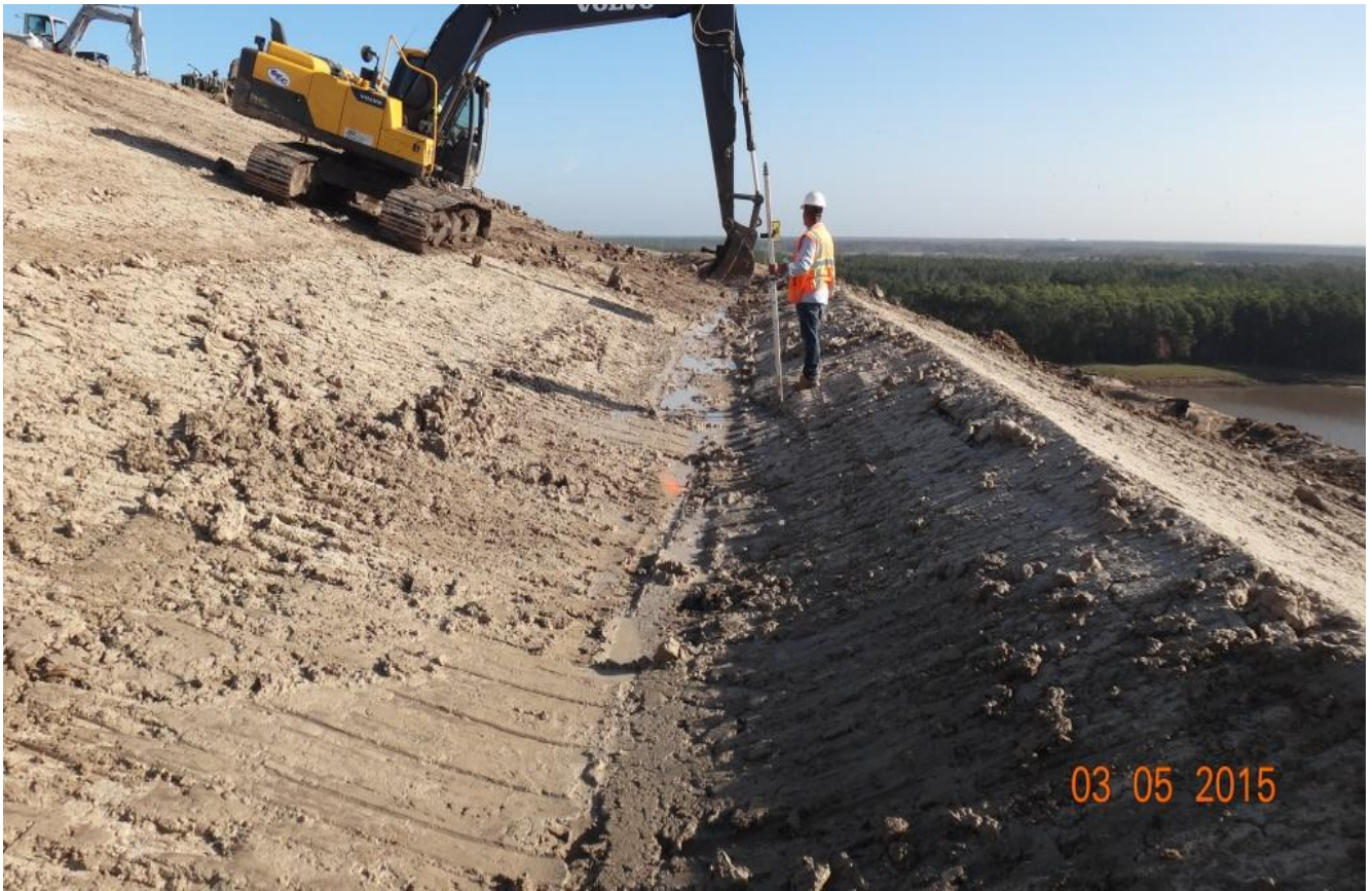
Grading Clay Swale for Underdrain Installation within Units 54 thru 56 (Facing Northeasterly) (March 2015)
