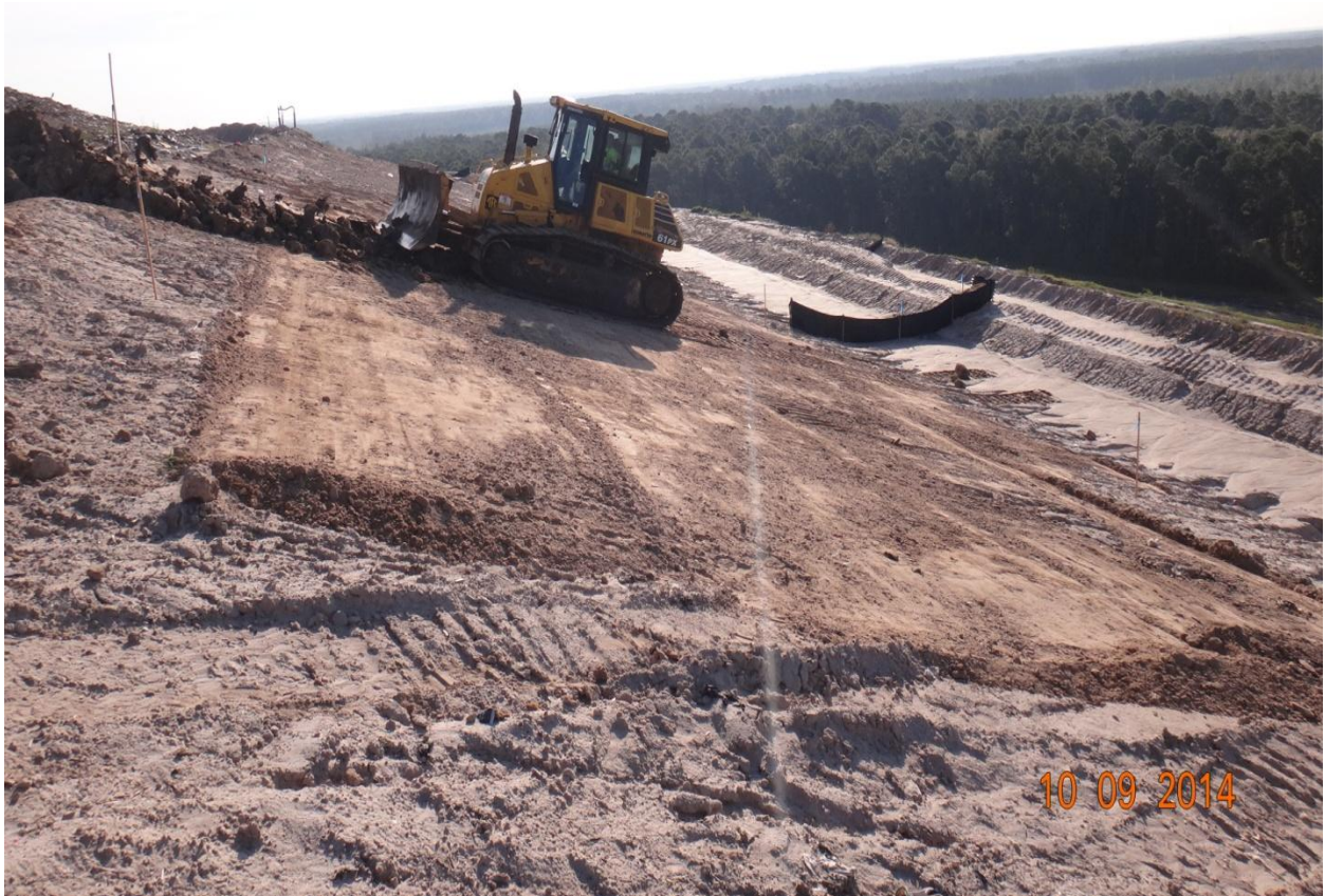
Grading initial cover at clay test strip (Facing East) (October 2014)
