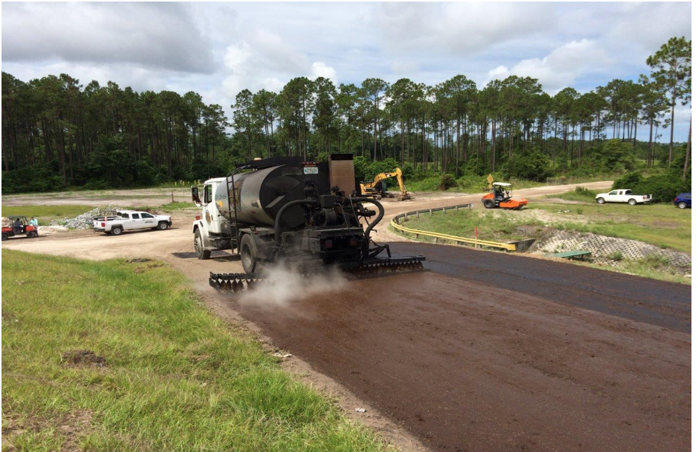
Prime coat installation for the maintenance road (facing southwesterly) (June 2015)
