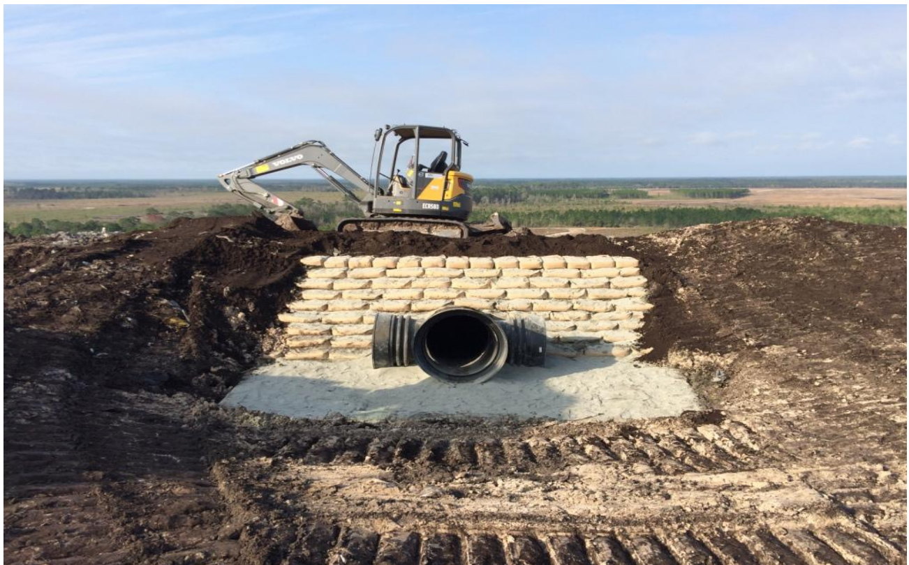
Installation of Rip Rap for Temporary Downcomer D-52 at Terrace 10 (Facing West) (March 2015)
