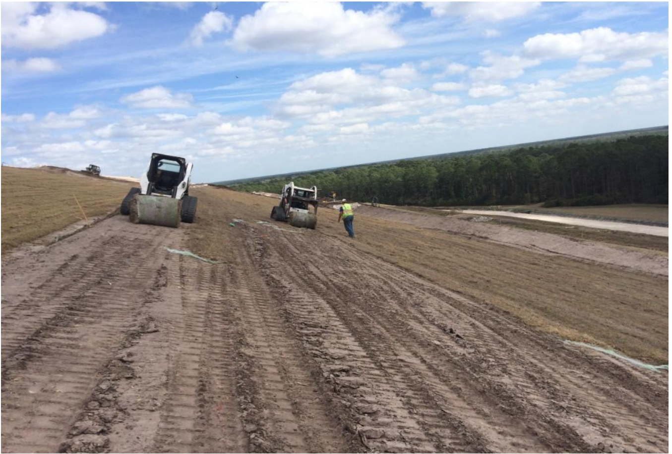
Placing Rolled Sod within Units 60 thru 62 (Facing East) (March 2015)
