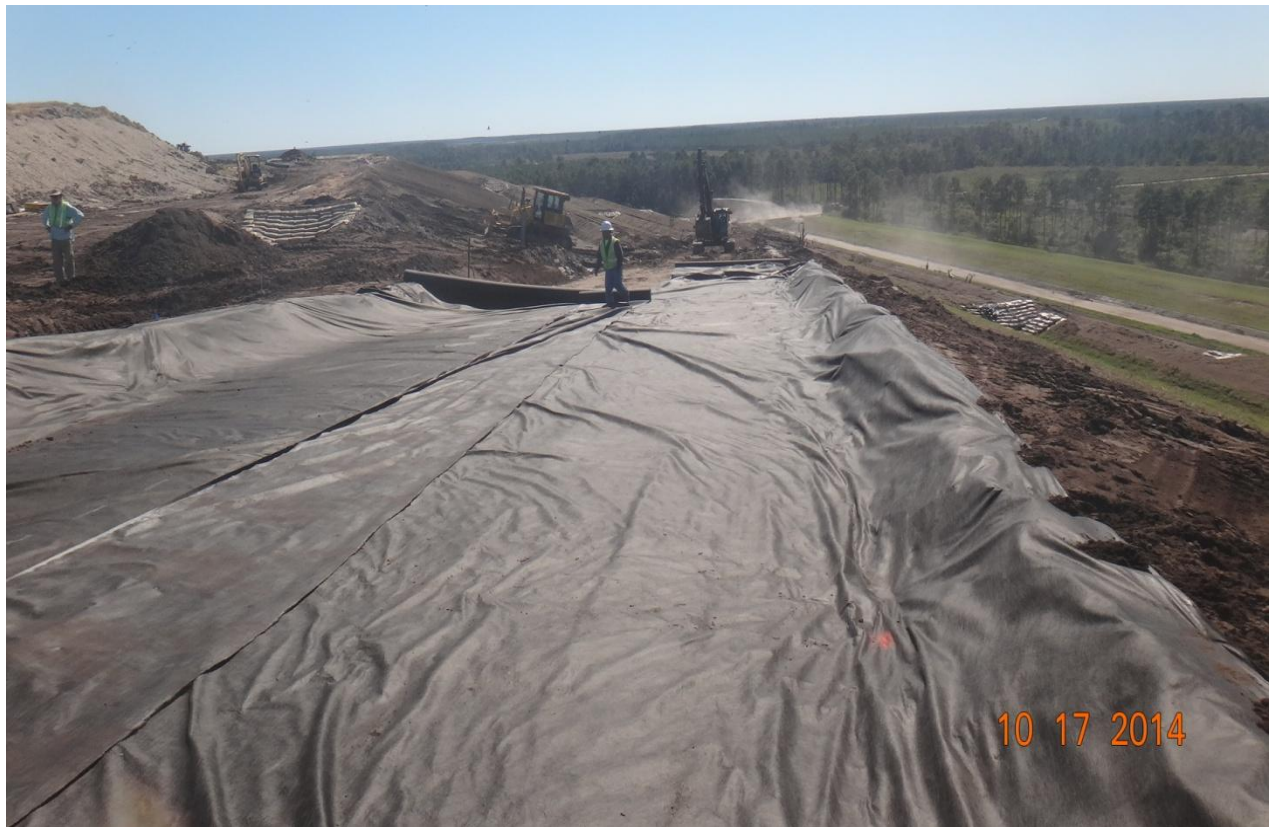
Installing geotextile prior to crushcrete placement for Maintenance Road (Facing South) (October 2014)
