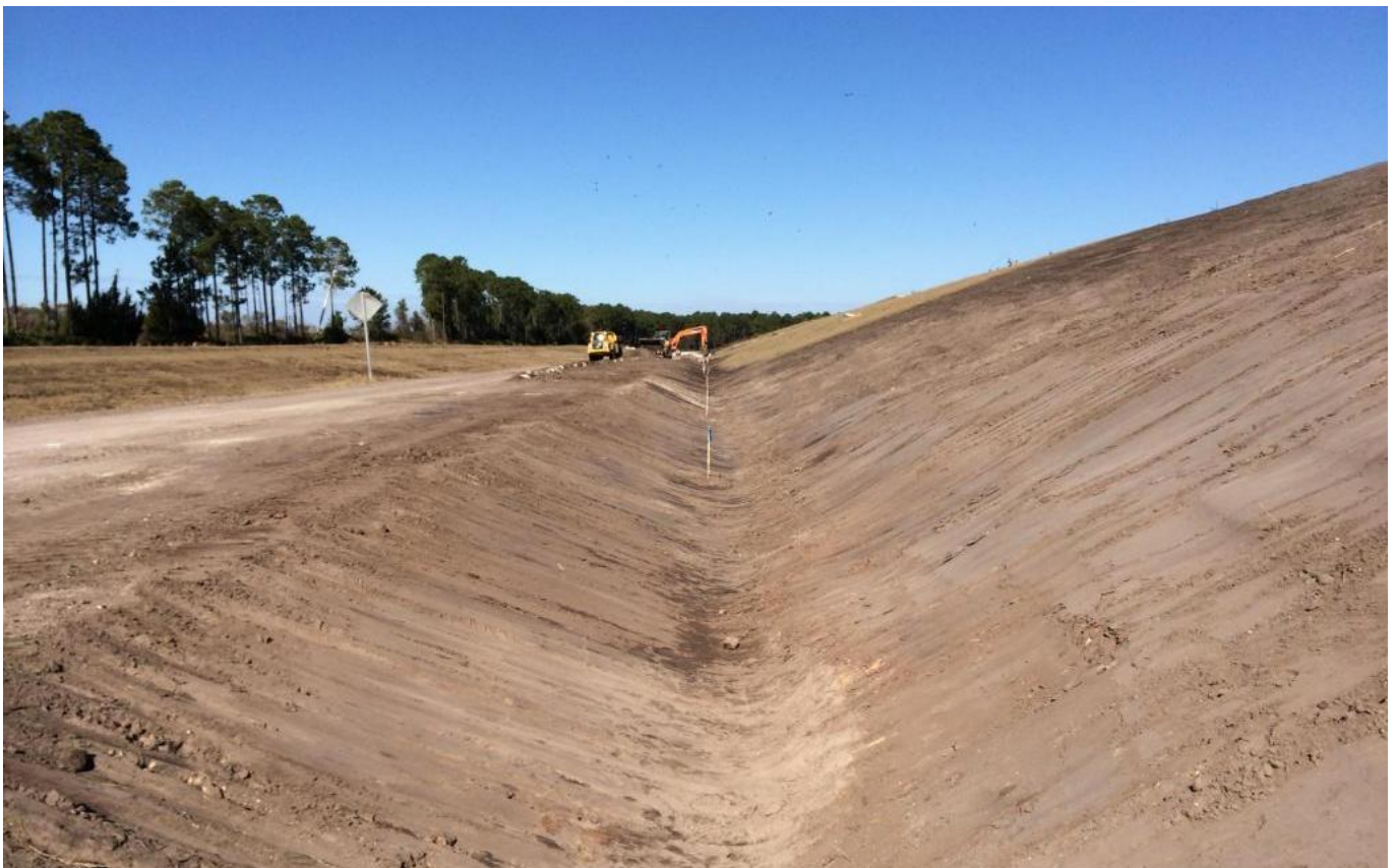
Grading Perimeter Road Swale (Unit 75) (Facing North) (December 2014)
