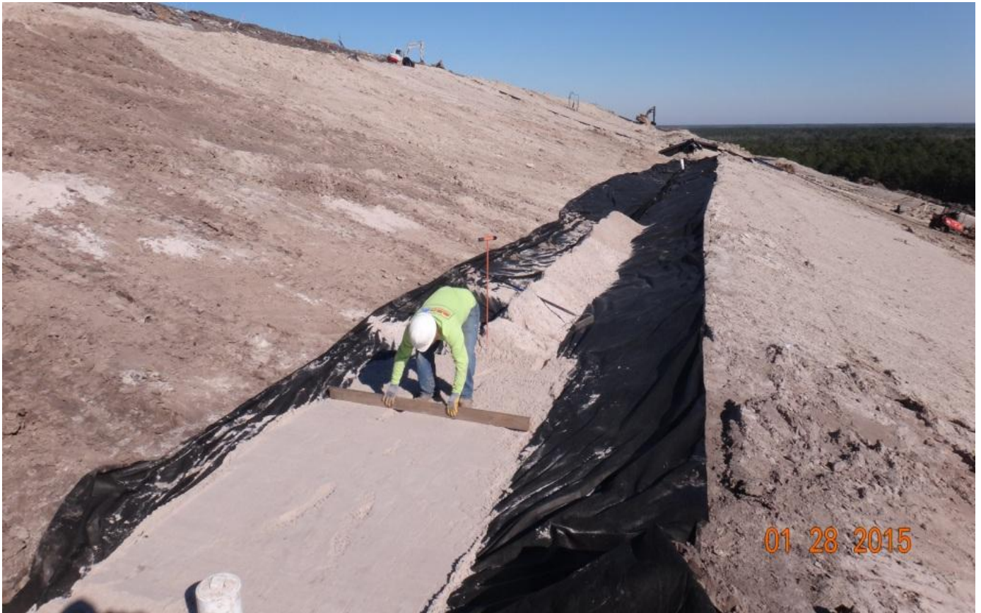
Leveling Underdrain Sand at Terrace 6 adjacent to D-41 (Facing East) (January 2015)
