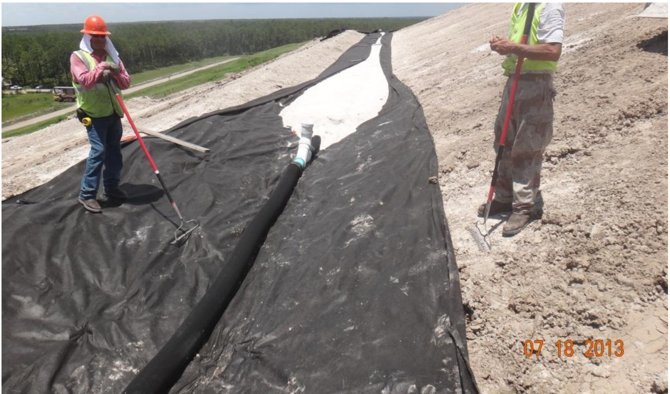
Installing Underdrain – Terrace 6 – Units 79-81 (facing North) (July 2013)
