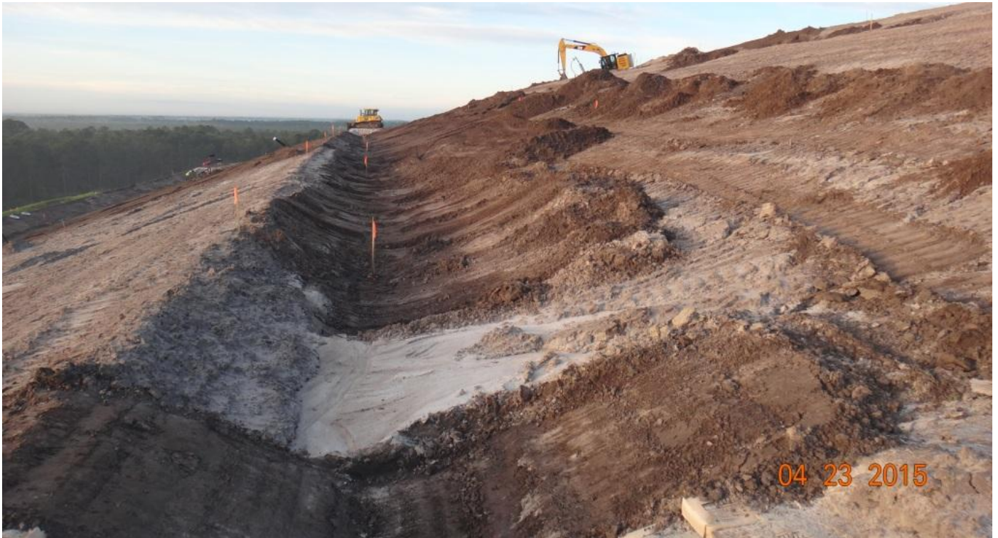
Grading Initial Cover within Units 51 -53 (Facing Southerly) (April 2015)
