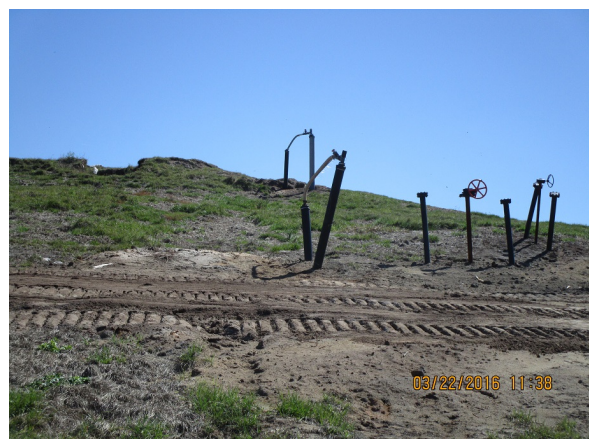
Additional wells installed Cell 8
