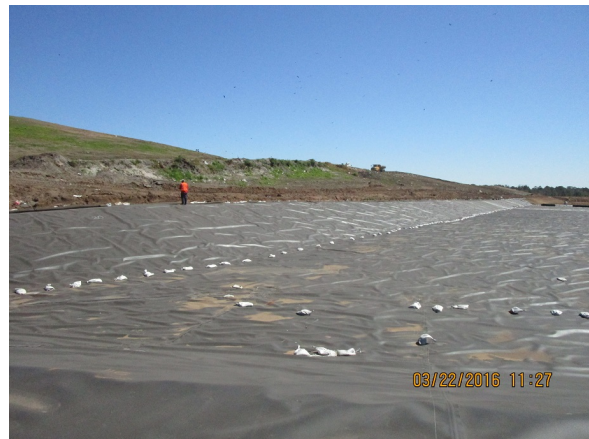
Liner installation Cell 13
