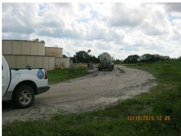
Leachate Storage Area
