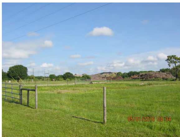
DEP May 1, 2016 Landfill Covered
