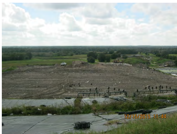
Working Face Overview Dec 2015
