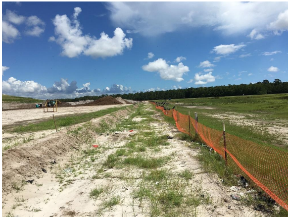
Berm and Fence Between Areas 3 & 4
