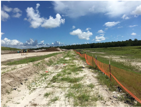
Berm and Fence Between Areas 3 & 4
