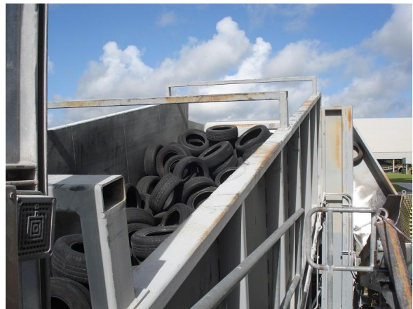
Tire feed bin to conveyer belt
